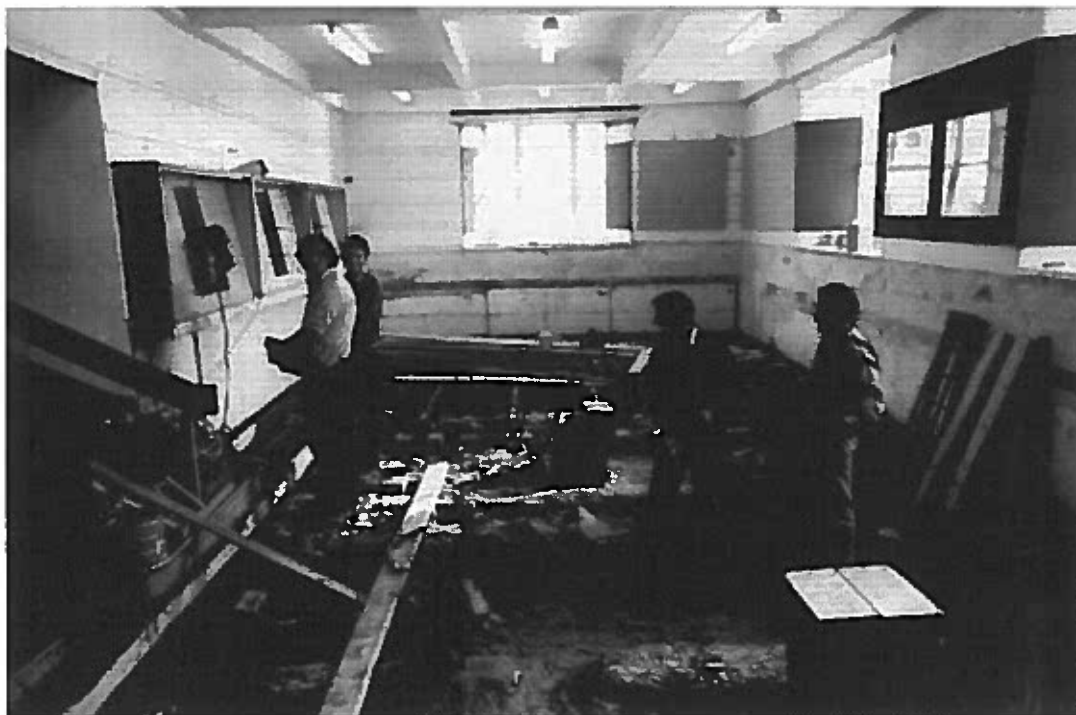
9. Lower Gallery, floor removed for lowering, 1987 TM&AG archive collection
