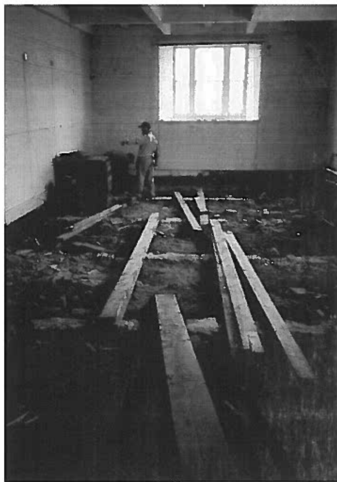
10. The Lower Gallery, floor removed before raising, April 2000 TM&AG archive collection
