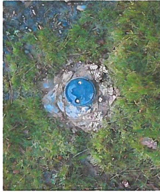
c. View of inspection well cover
