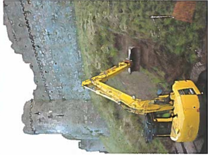
b. Landslip area under excavation
