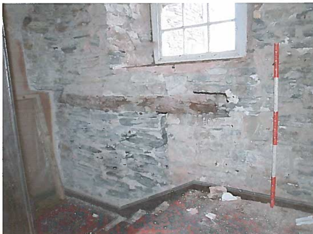
Plate 30. Gilfach-y-berthog - Evidence for blocked in 1st floor window in west wall of former early 17th century house. Looking west.
