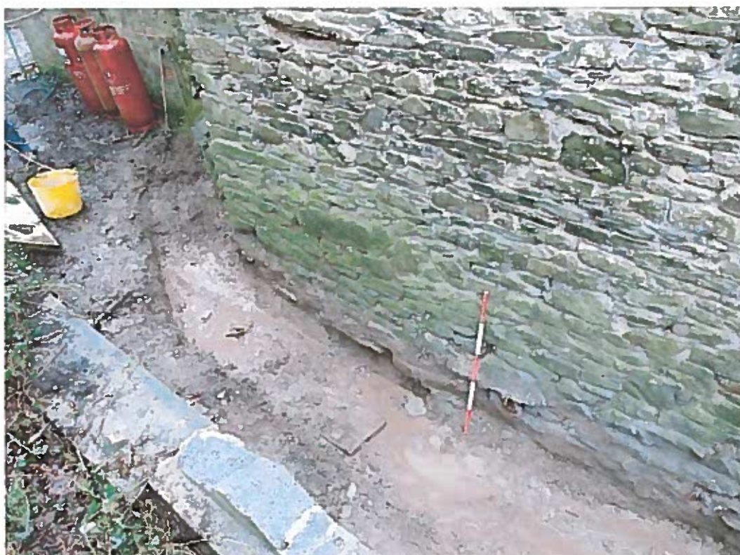
Plate 46. Galfach-y-berthog - Rear of house following removal of modern concrete base and ground reduction for drainage (ST1). Looking west.
