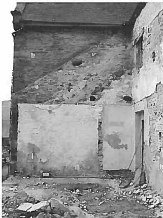
Plate 82. Gylfach-y-berthog - Former 19th century kitchen extension demolished in preparation for new proposed kitchen extension. Note earlier extension outline. North facing elevation.
