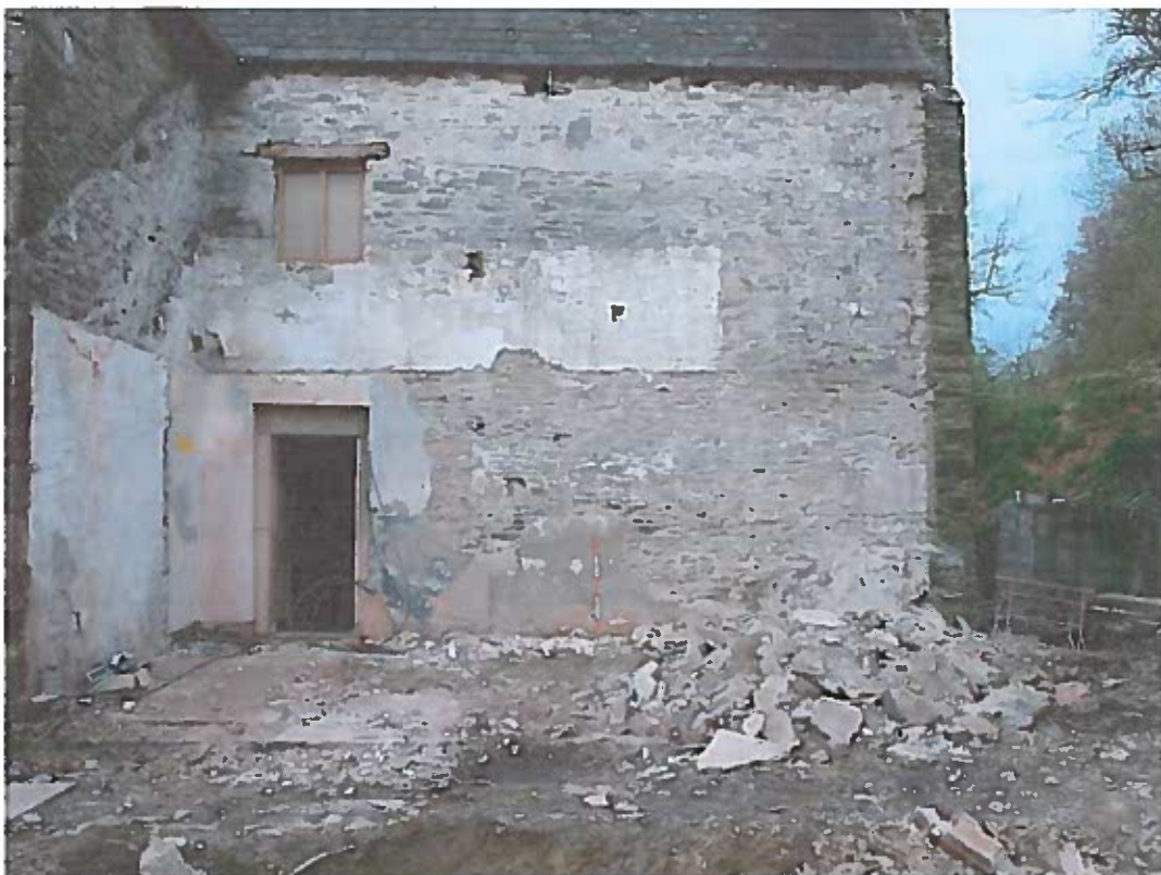
Plate 80. Gilfach-y-berthog - Former 19th century kitchen extension demolished in preparation for new proposed kitchen extension. East facing elevation.
