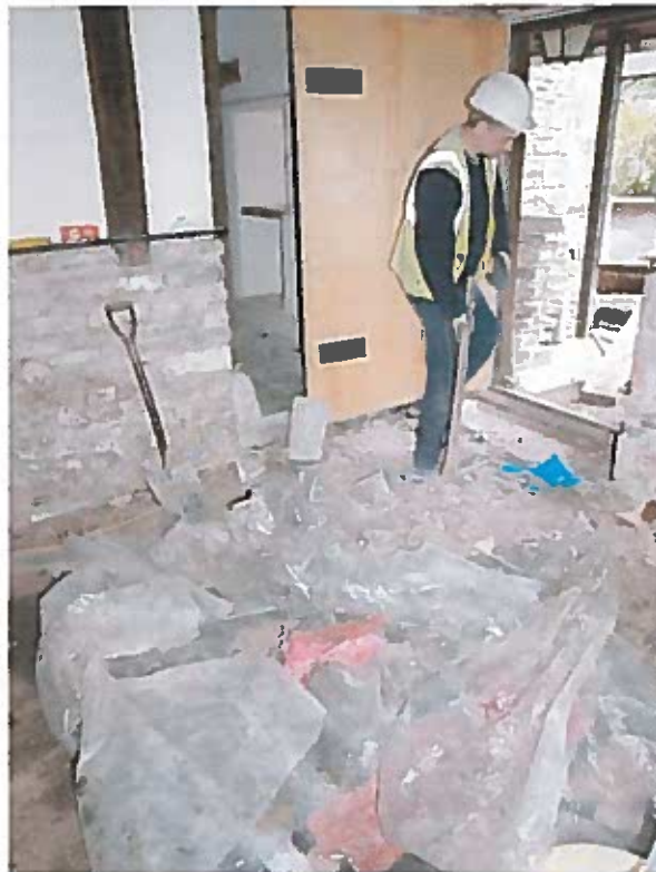
Plate 49. Gilfach-y-berthog - Working shot during removal of modern stone floor tiles from Lower Parlour Room during ground reduction. Looking southwest.
