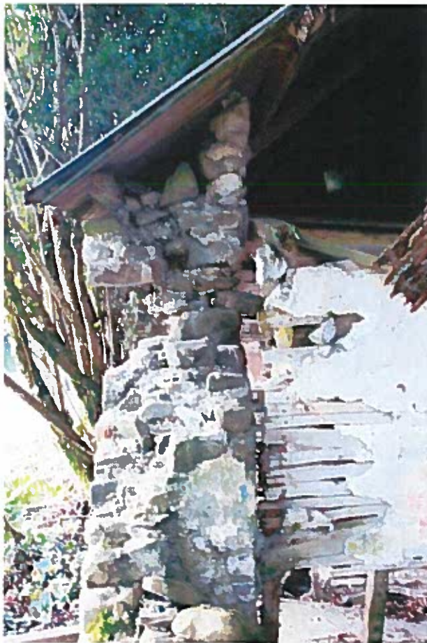
Figure 8. Tairheol: infill between wall top and underside of roof.
