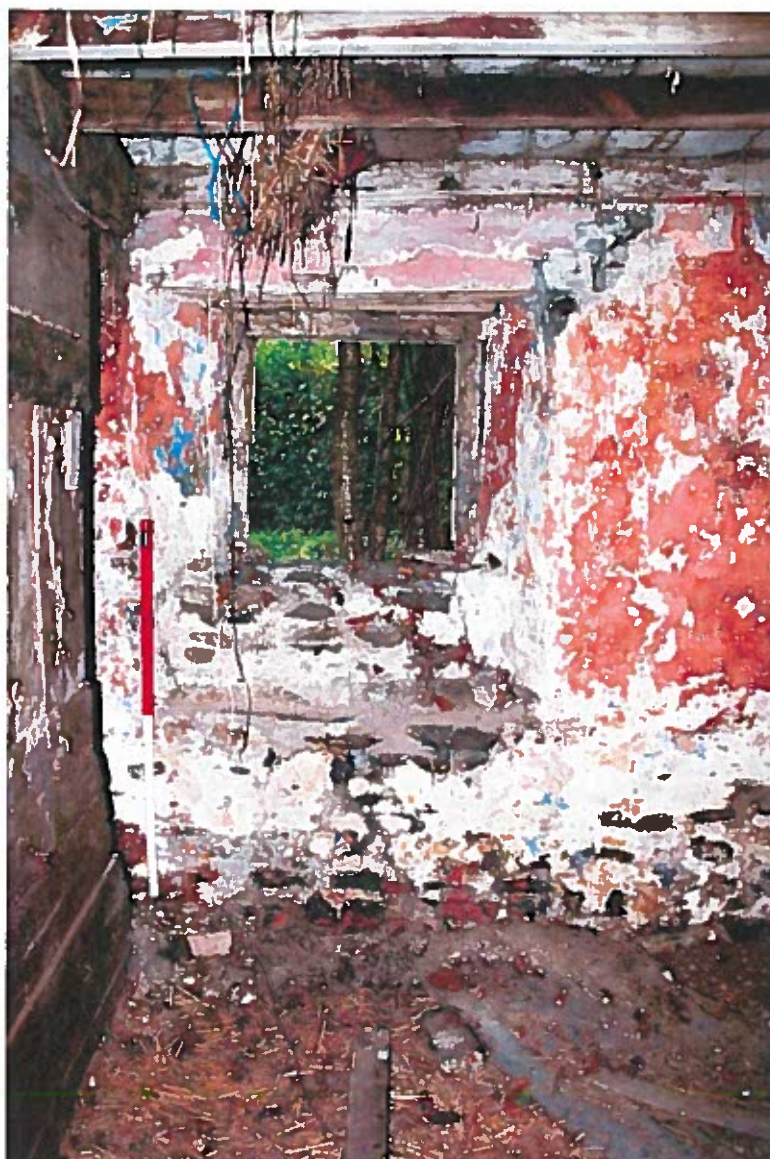
Figure 13. Tairheol: rubble stone in-fill above window sill.
