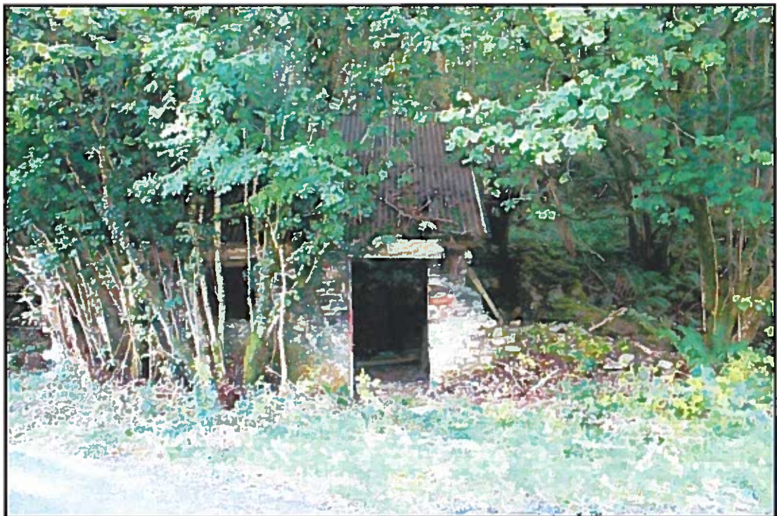
Figure 2. Tairheol: collapse of northern elevation and northern part of front elevation.
