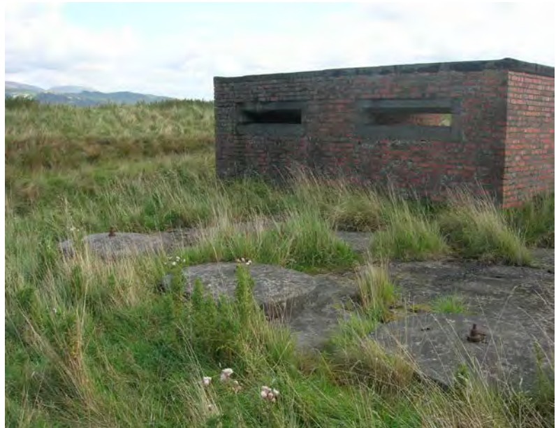
Figure 20: A camera/observation post built to a specification forwarded by the Experimental Establishment at Walton-on-the-Naze with concrete bases for Kine Theodolite or experimental radar (NPRN 408403-4, 506534)
