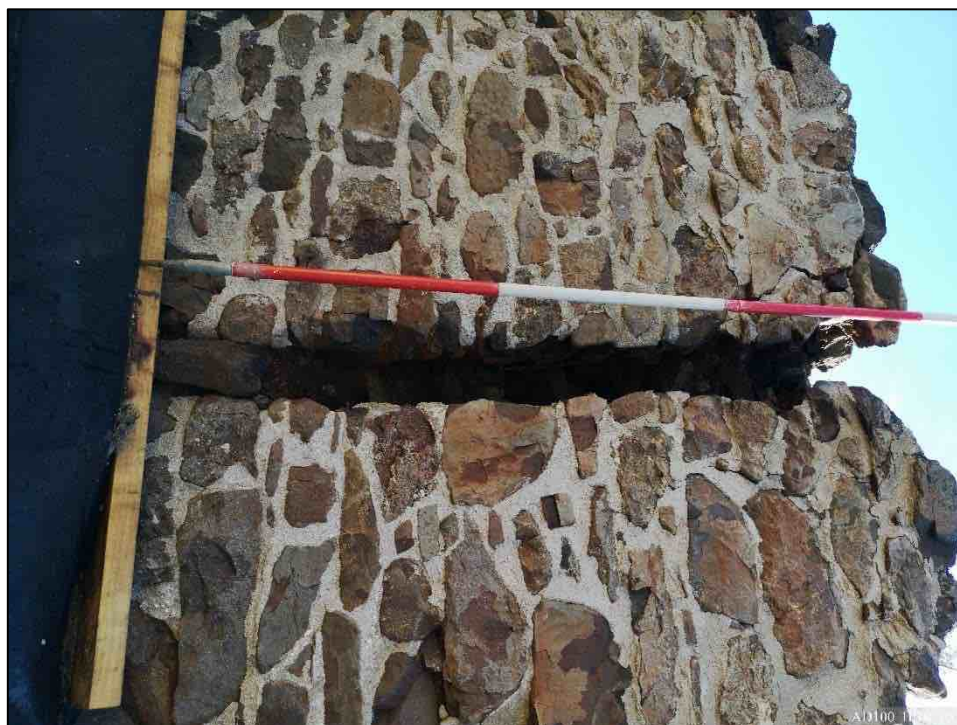
Plate 53 – Cruck pocket for T5 to east lateral wall.
