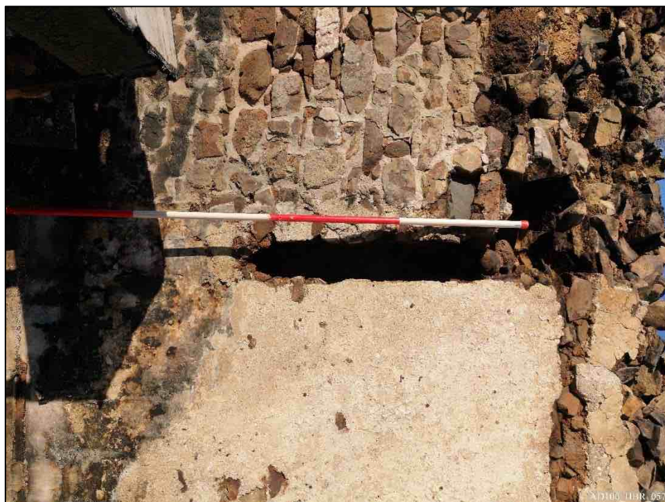
Plate 57 - Cruck pocket for T5 to west lateral wall.
