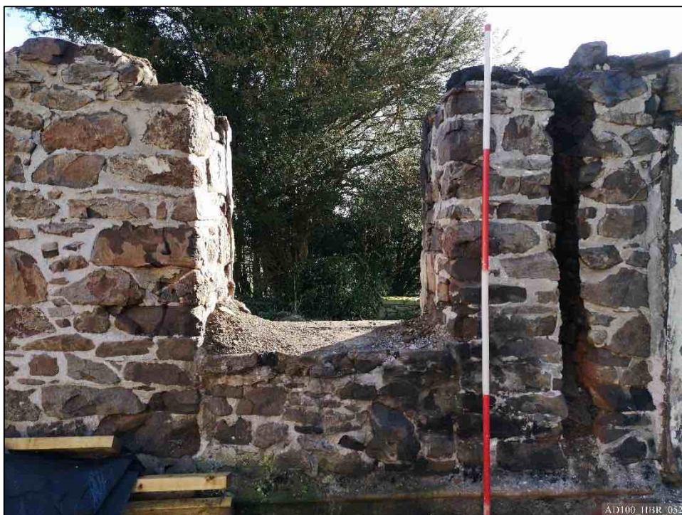
Plate 52 – View east, showing infill to 18 th century doorway to create a window.
