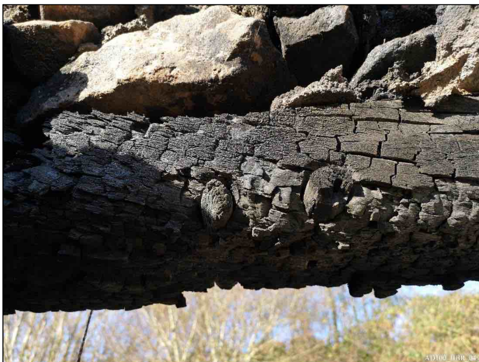
Plate 49 – Reused timber lintel, showing pegs in situ.
