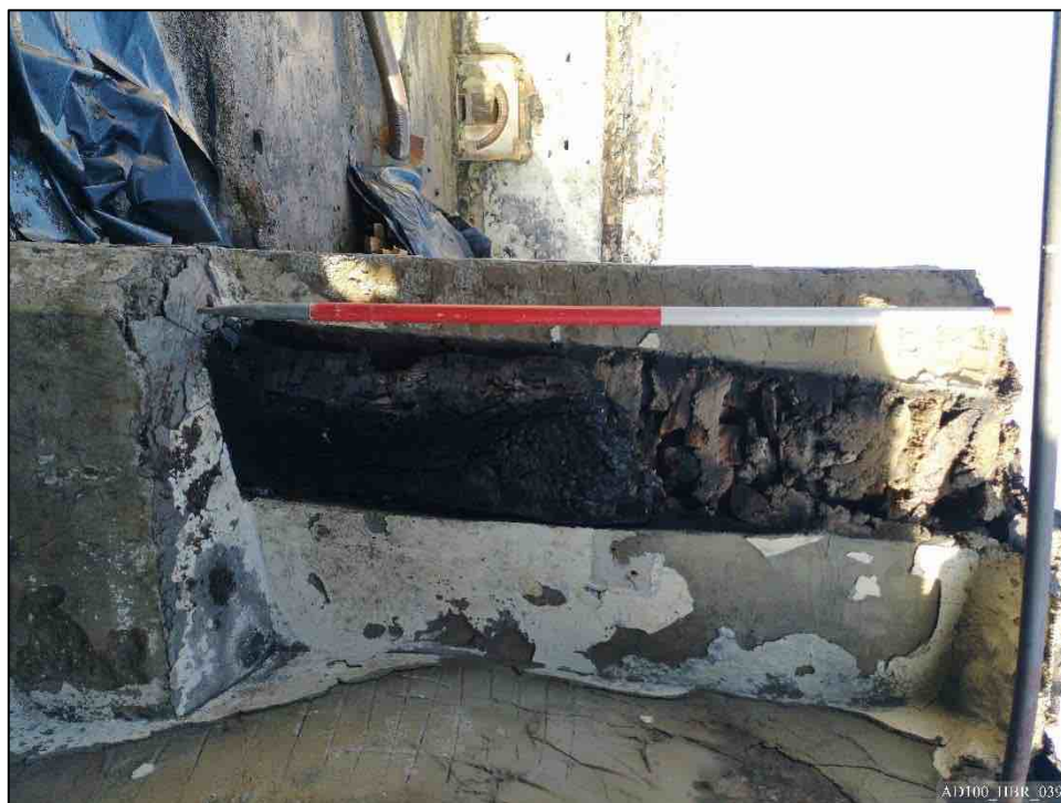
Plate 39 – Remains of cruck T2 to east lateral wall.
