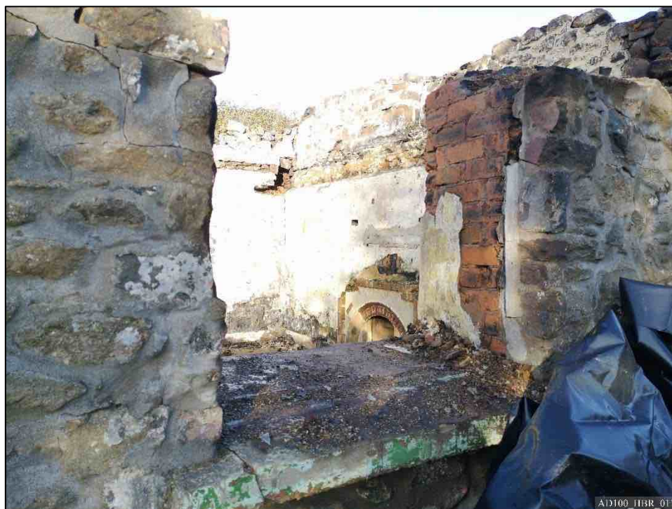
Plate 11 – East elevation showing enlarged window to parlour.
