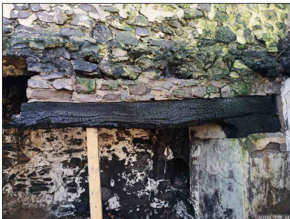
Plate 42 – View south, showing remains of fireplace bressummer and transverse beam over.
