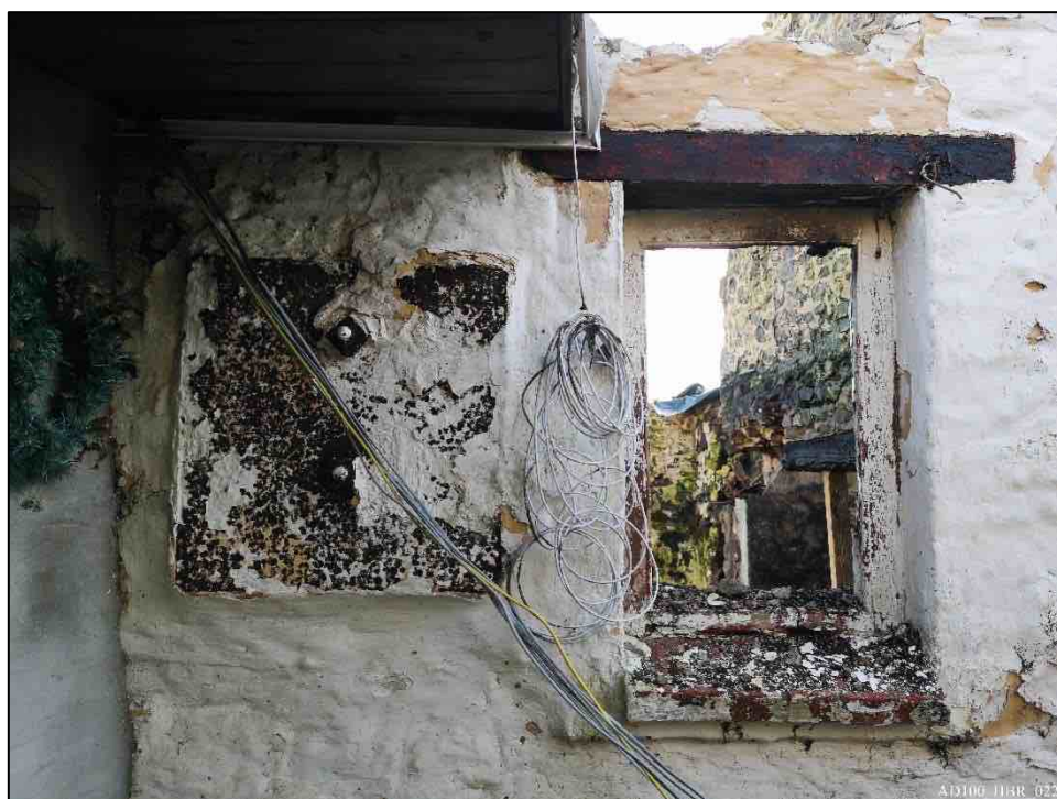
Plate 22 – West elevation, showing wall tie plate.
