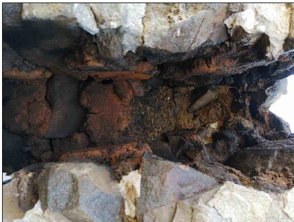
Plate 46 – View inside of cruck pocket T3, showing clay-earth mortar.
