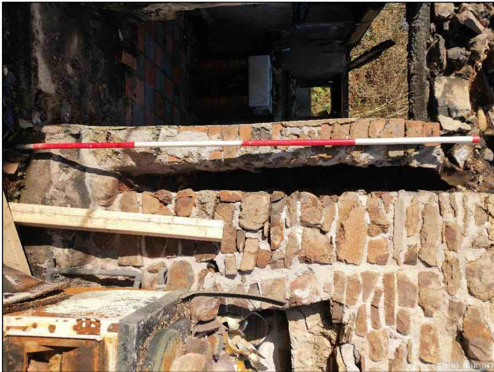
Plate 47 – Cruck pocket for T3 to west lateral wall.
