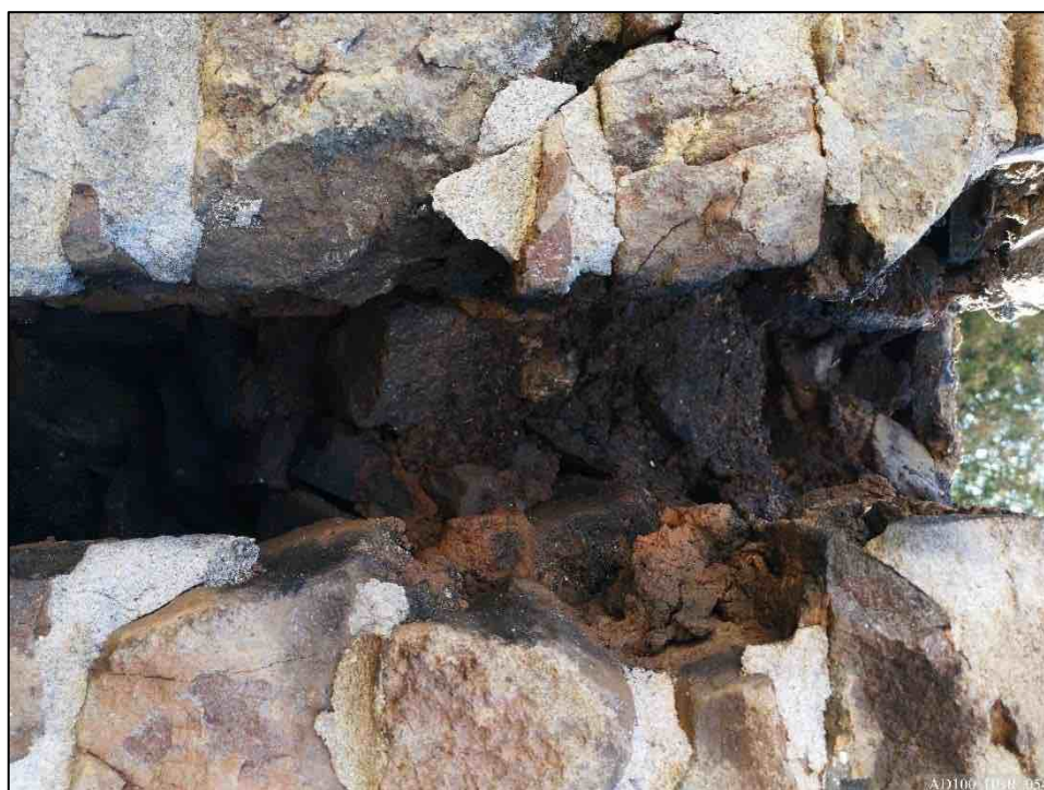
Plate 54 – View inside cruck pocket, showing clay-earth mortar.
