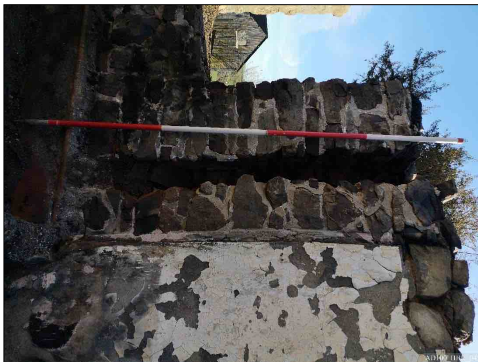
Plate 45 – Cruck pocket for T3 to east lateral wall.
