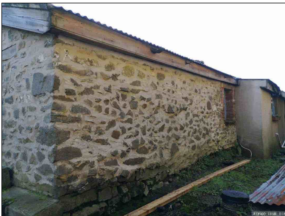
Plate 18 – West elevation of pantry, showing later window with red brick reveals.
