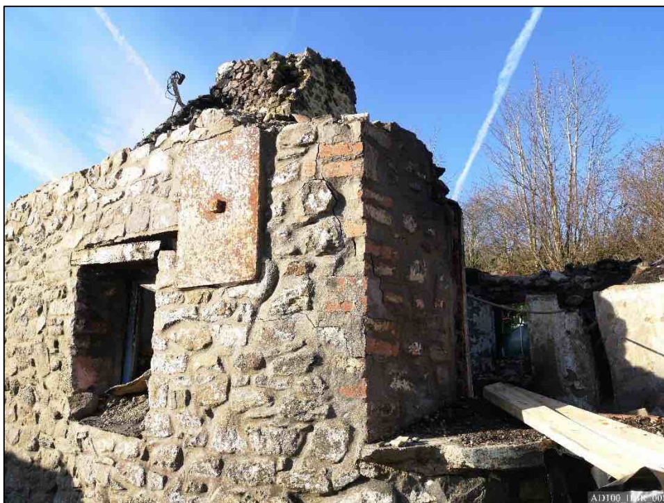
Plate 8 – East elevation, showing rebuild window reveal in red brick.
