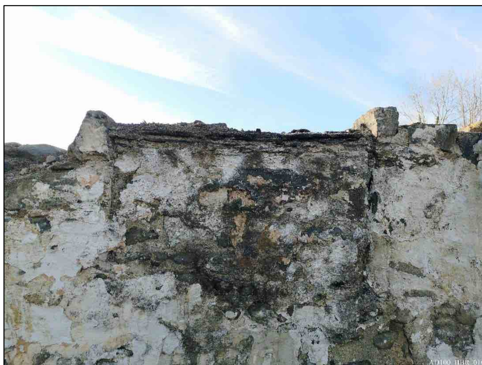
Plate 16 – North elevation, showing joints in masonry from first floor doorway.
