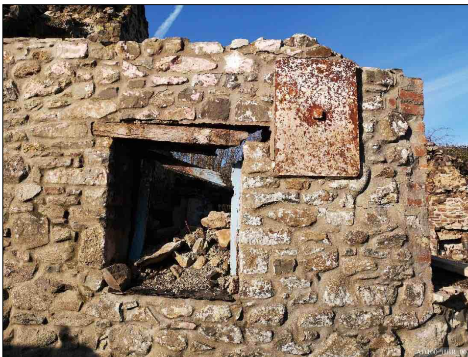
Plate 7 – East elevation, showing tie plate to stair projection.
