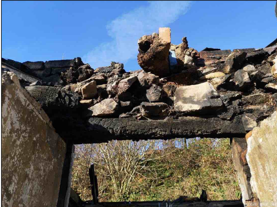
Plate 48 – View to north of south doorway to kitchen, showing reused timber as lintel.
