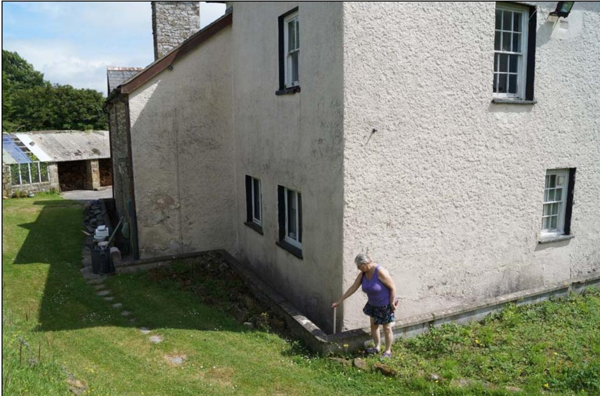
*Plate 35: RWT2017\_135, corner of northwestern and northeastern faces of Robeston House showing how the house is set down into the slope, looking southeast.*
