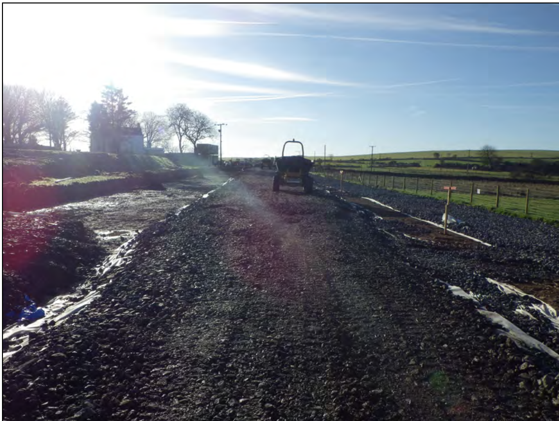
Plate 4: POB2013_103, the stripped area with the central section laid with membrane and stones laid north northeast.
