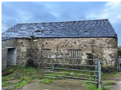
04. Northern facing stone wall with partly in-filled openings, along with the existing courtyard.
