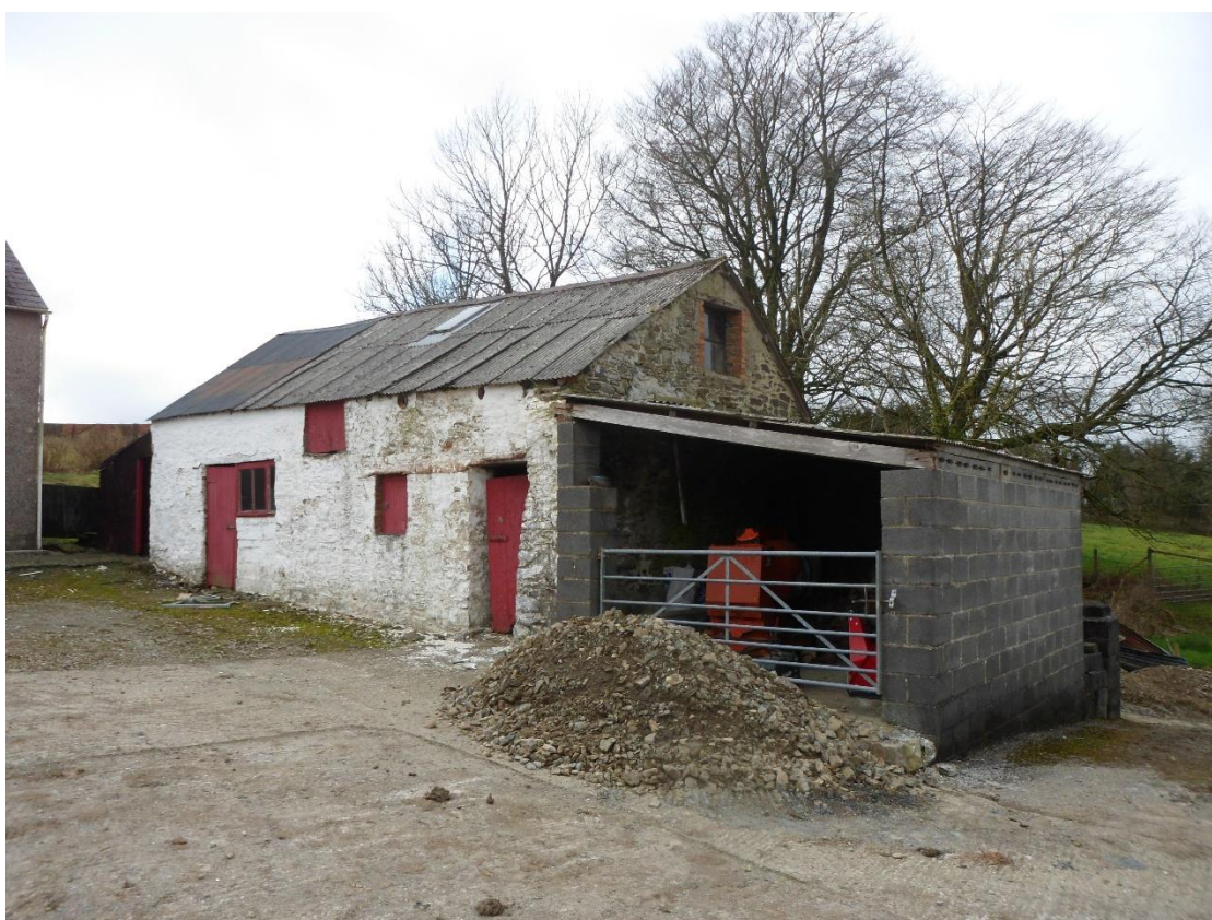
South East facing / Front Elevation to outbuilding – part traditional part blockwork
