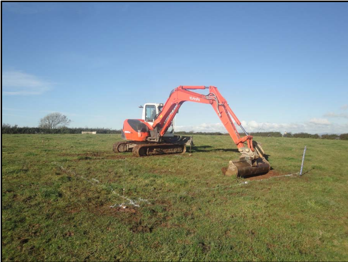
Plate 1: MYD2012_001, Stripping turf in Area 1 for foundation of turbine, looking west southwest.
