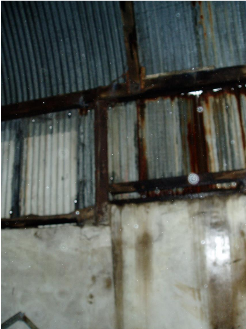
8) South Wall of Barn D (Interior)
