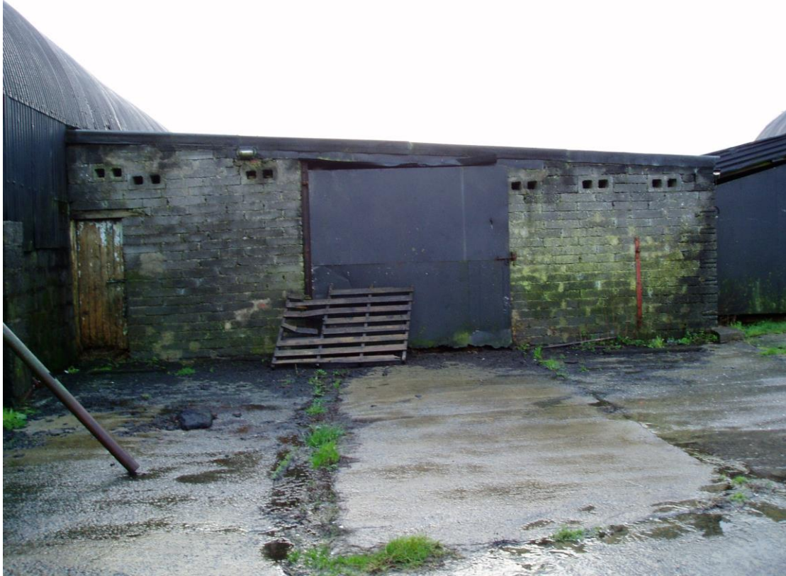
23) North East Elevation of Building C – Doors
