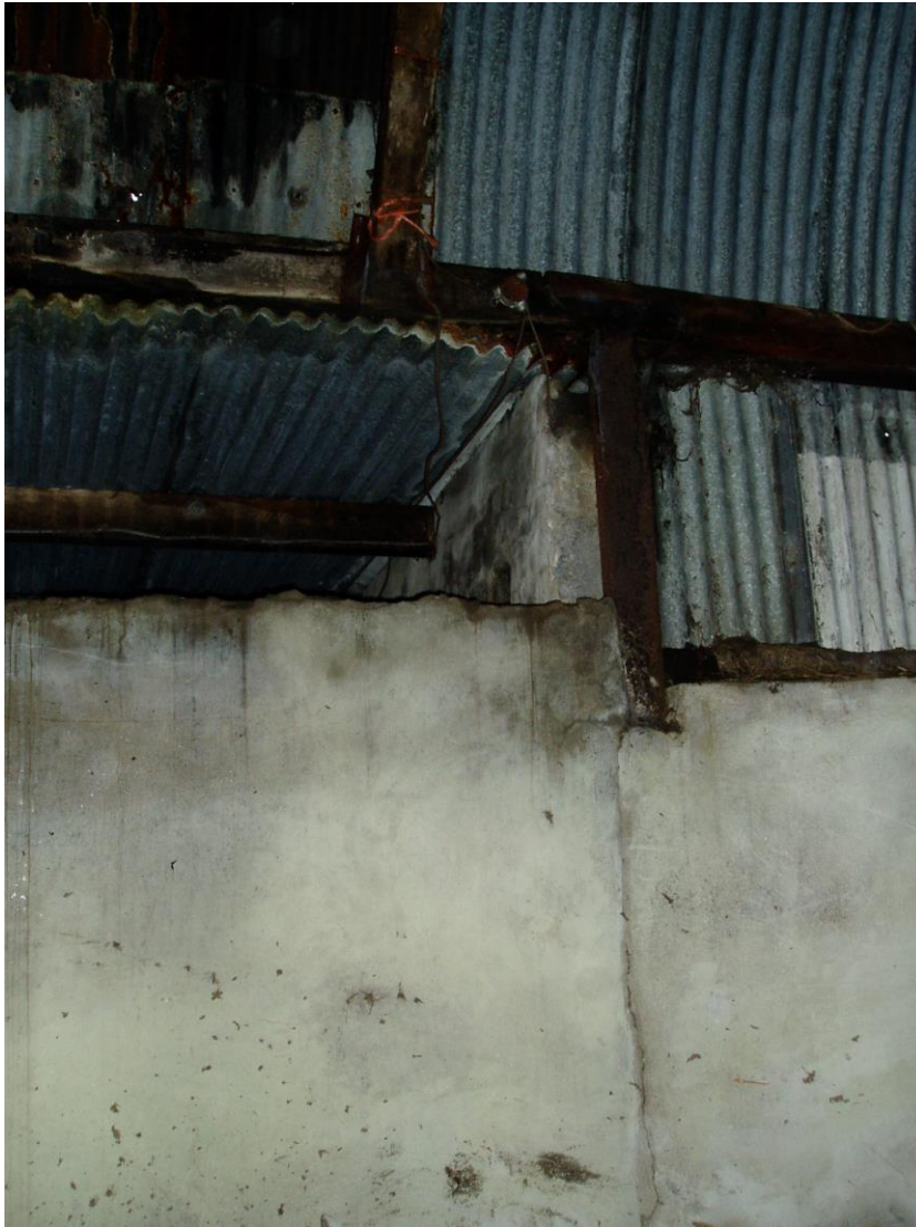
7) North Wall of Barn D (Interior)
