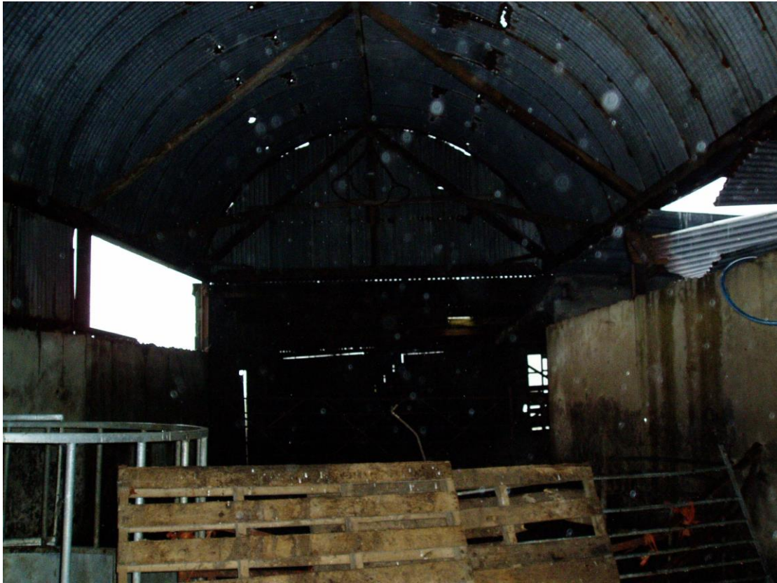
5) Interior of Barn D Looking to J
