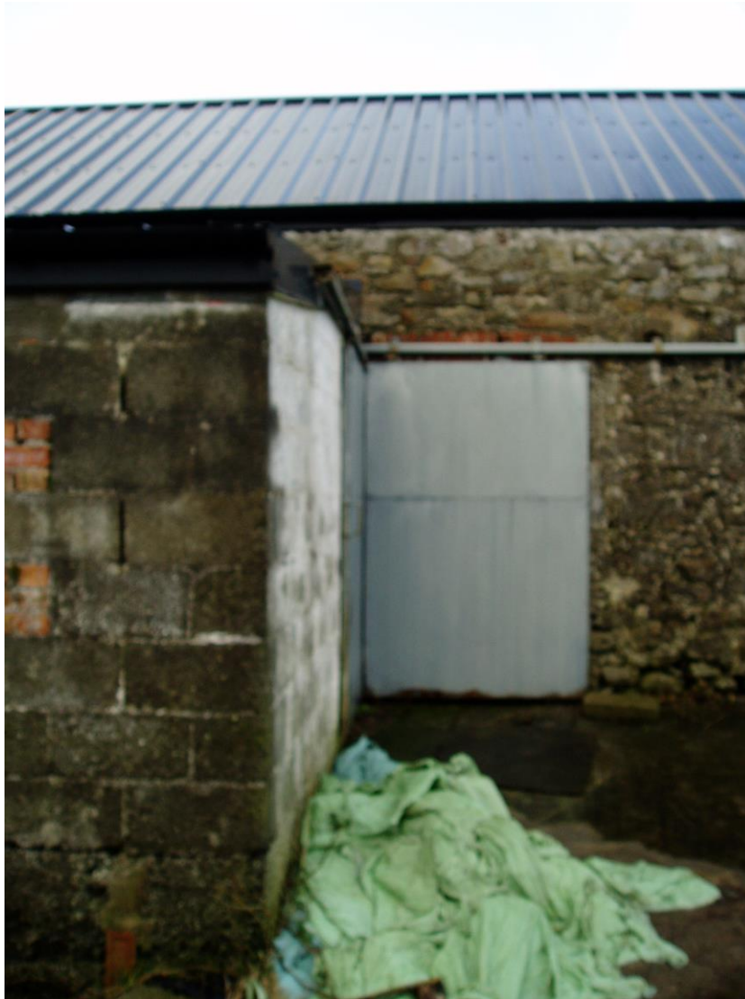
43) South East Elevation of Buildings F - Doorway
