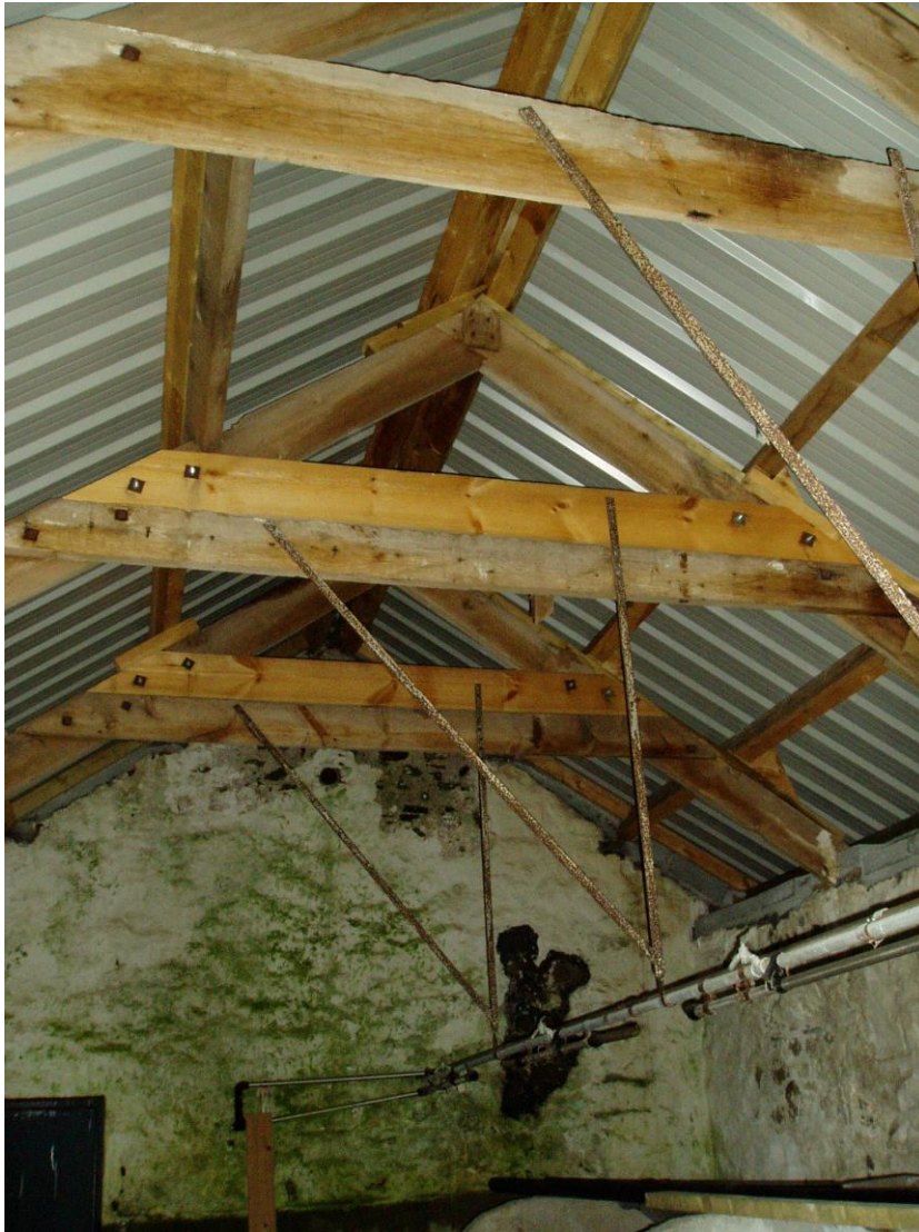
12) Interior of Milking Parlour F – Roof Detail
