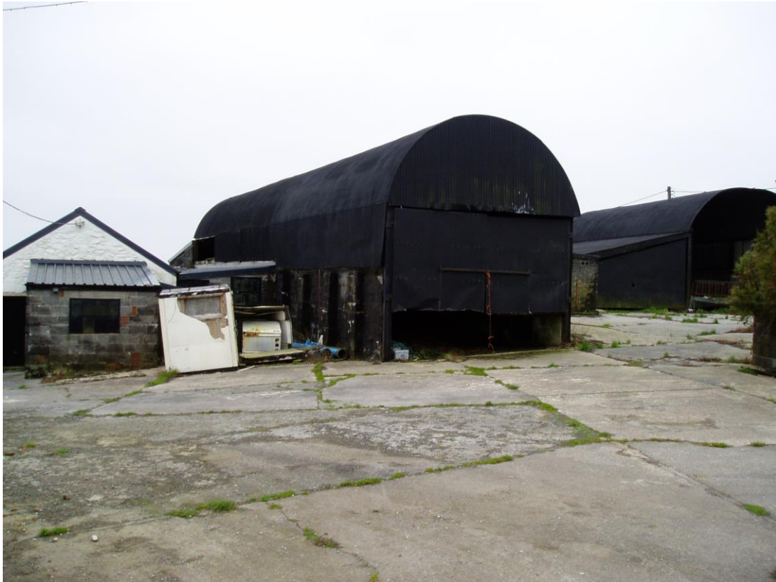
48) General View From the East Showing Buildings A, B, D, E, G and H
