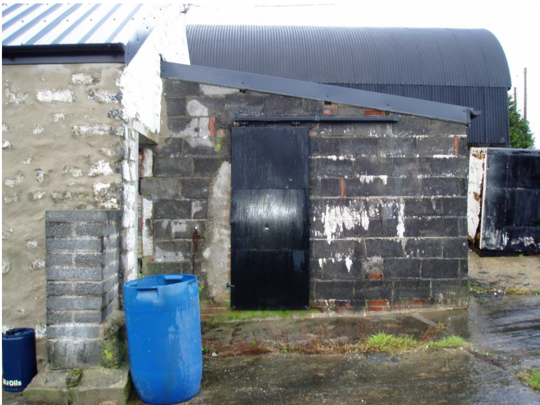
45) South East Elevation of Building H
