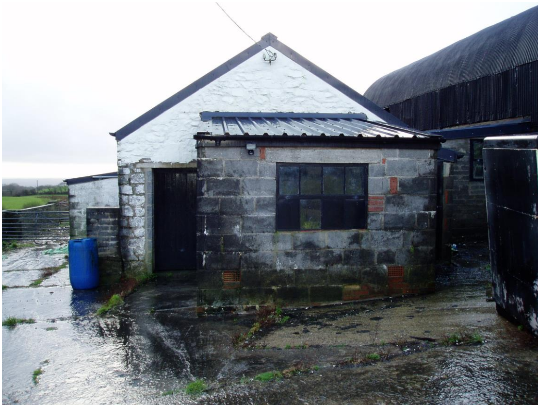
18) Exterior Elevation North East Wall of Building H
