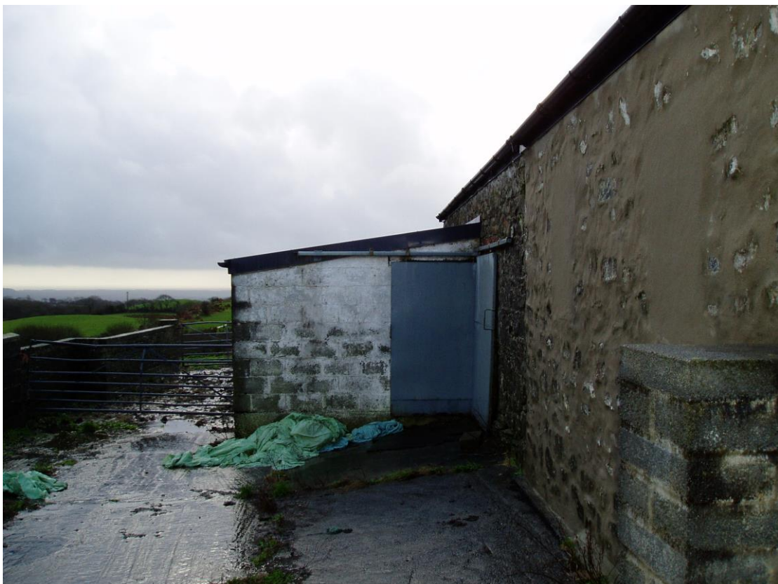
19) Exterior Elevation North East Wall of Building I
