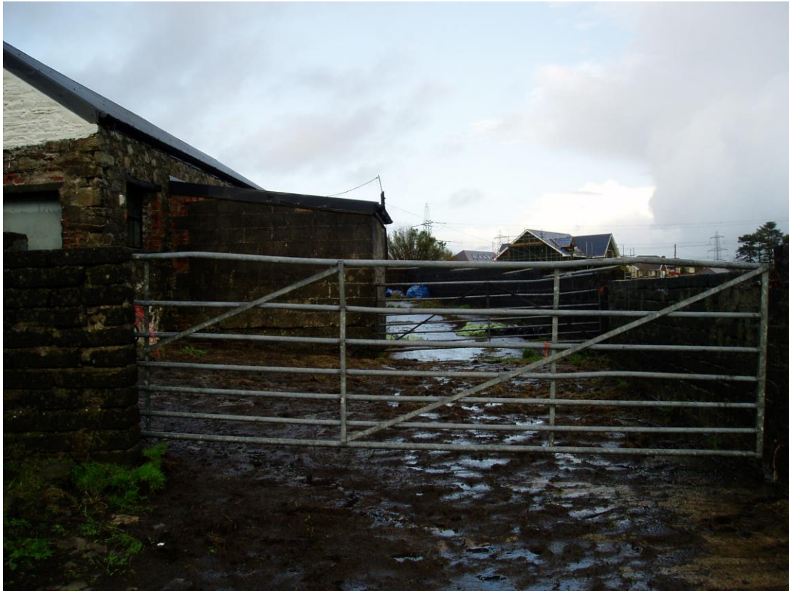
40) South West Elevation of Building I and Gate
