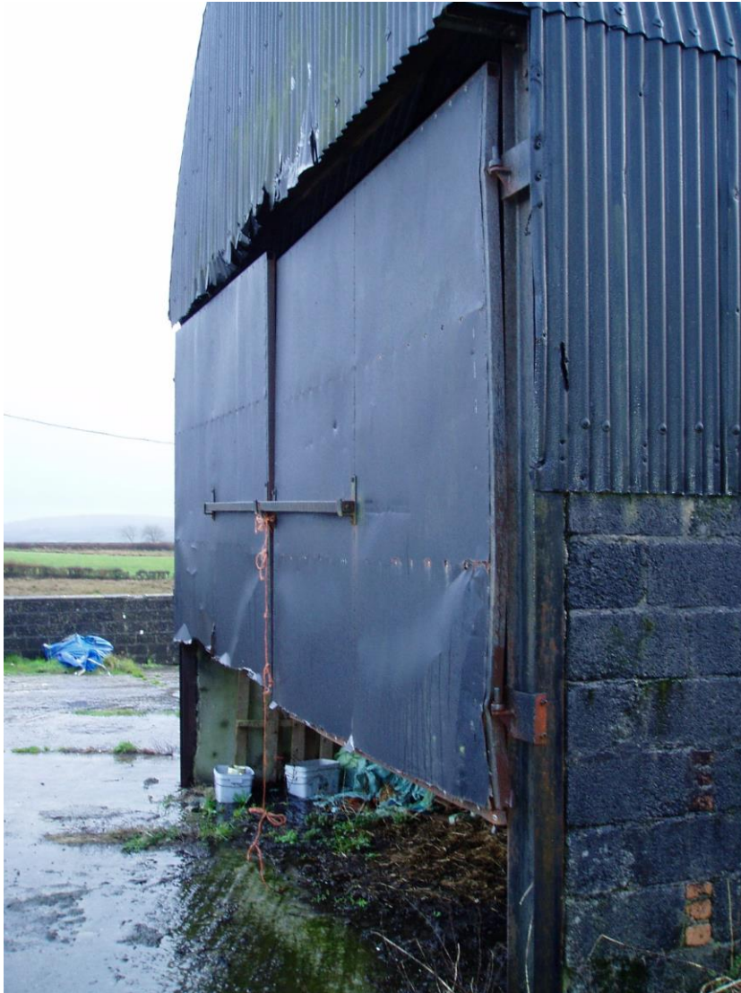
22) North East Double doors of Barn D – Detail
