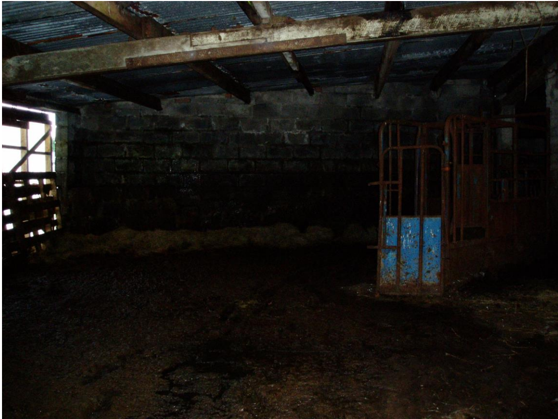
36) Interior of Building J From the South East Doorway
