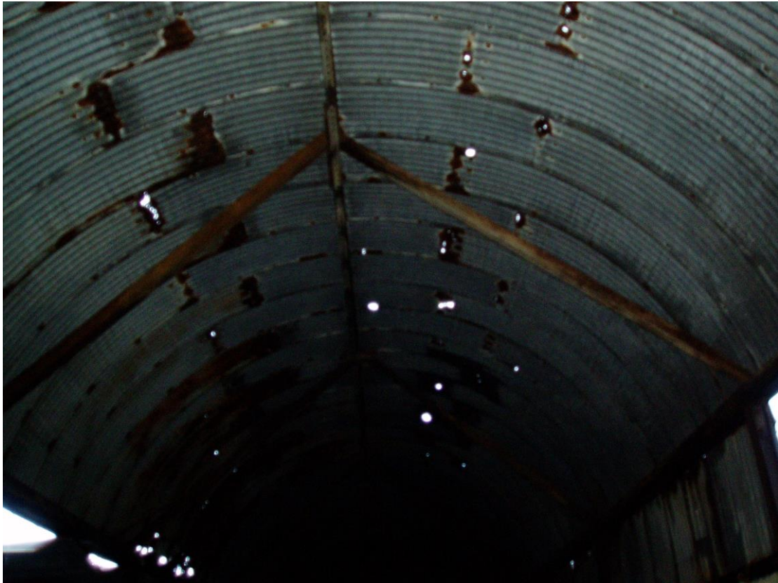
34) Interior of Building D Roof Showing Crane Arrangement
