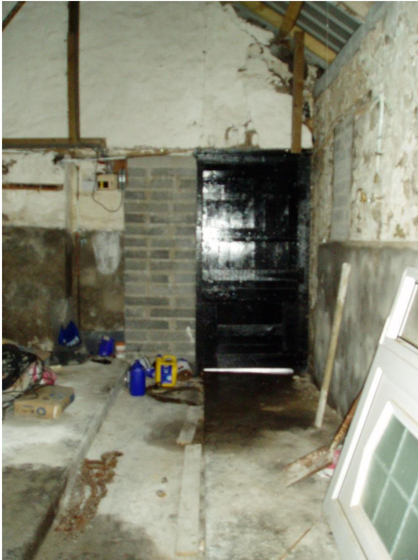
11) Interior of Milking Parlour Extension G, Looking to the East Door
