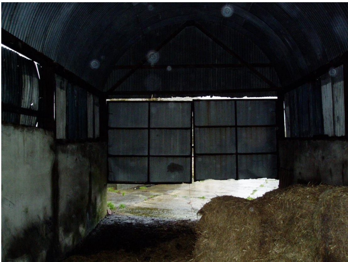
6) Interior of Barn D Looking to Entrance Doors
