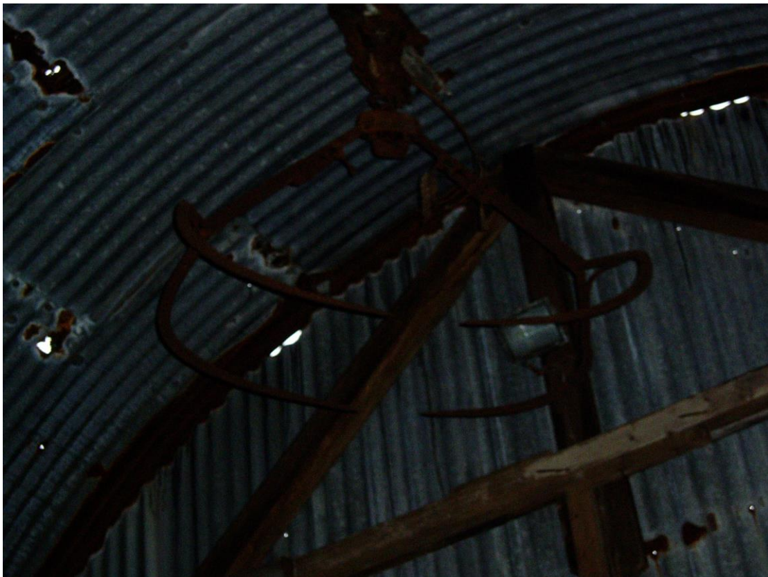
51) Interior of Roof D Showing Crane Equipment
