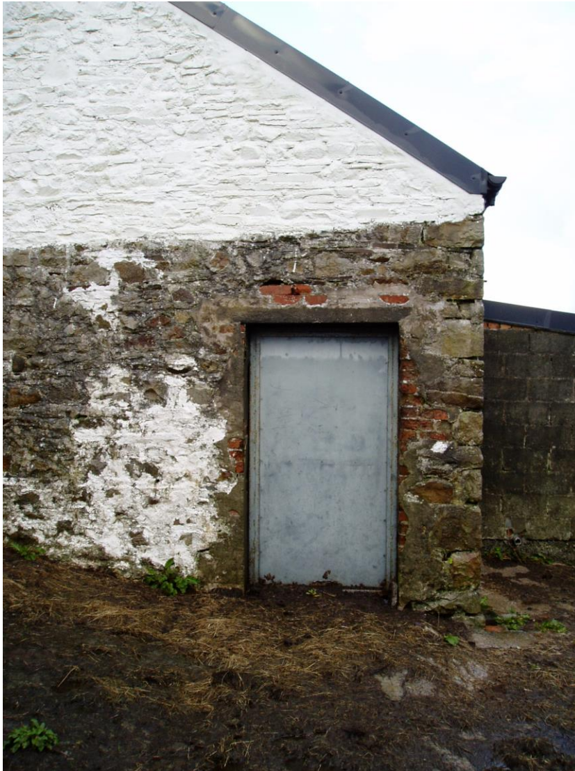
39) South West Elevation of Building F Showing Door
