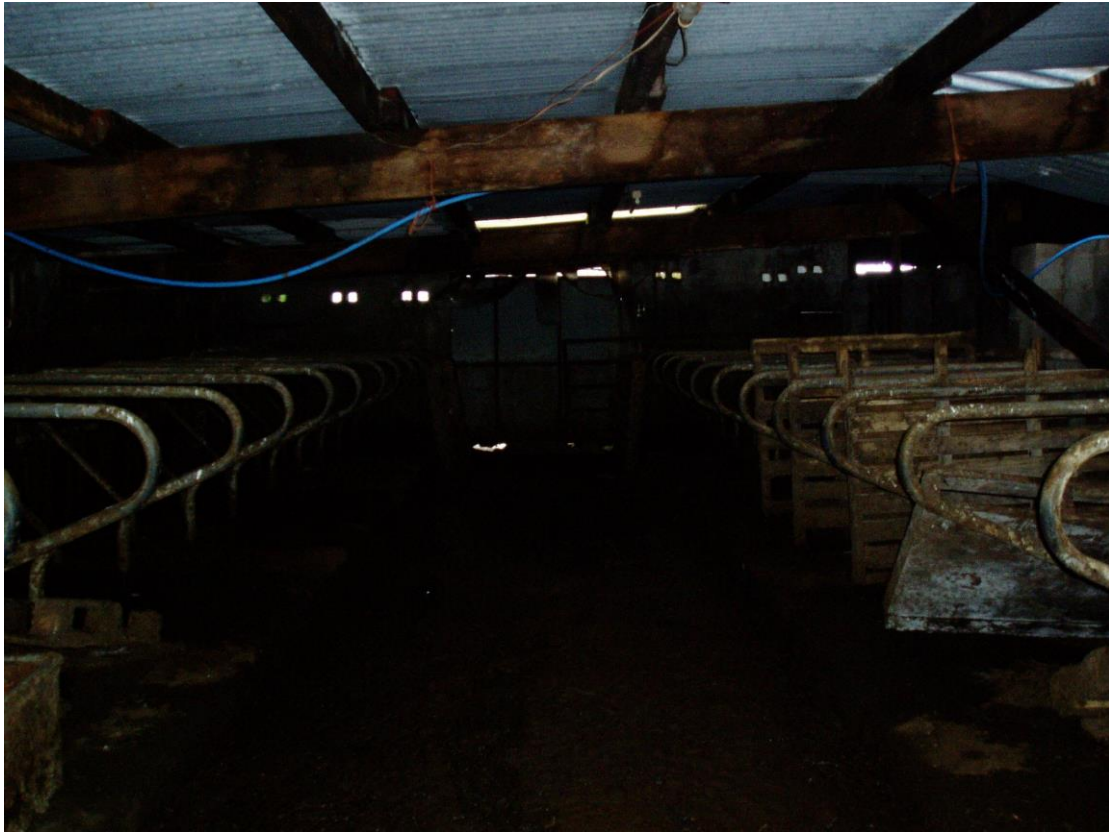
52) Interior of Building C from J
