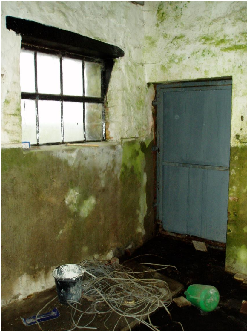
16) Interior of Milking Parlour Extension G – Door and Window
