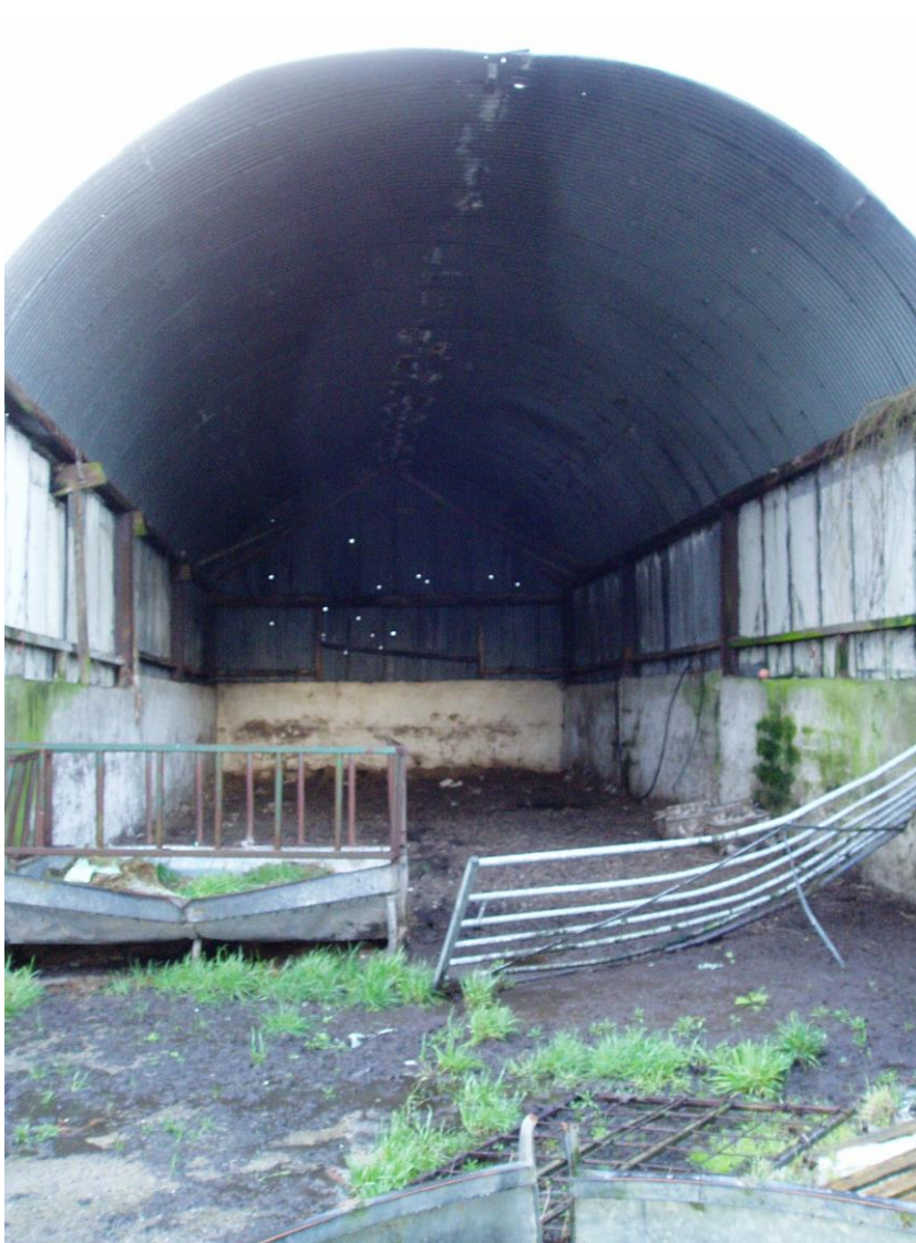
25) North East Elevation of Building A
