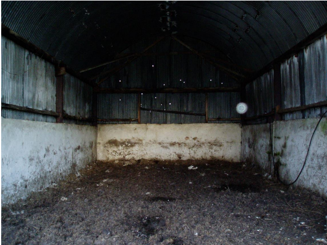
26) Interior of Building A Looking South West
