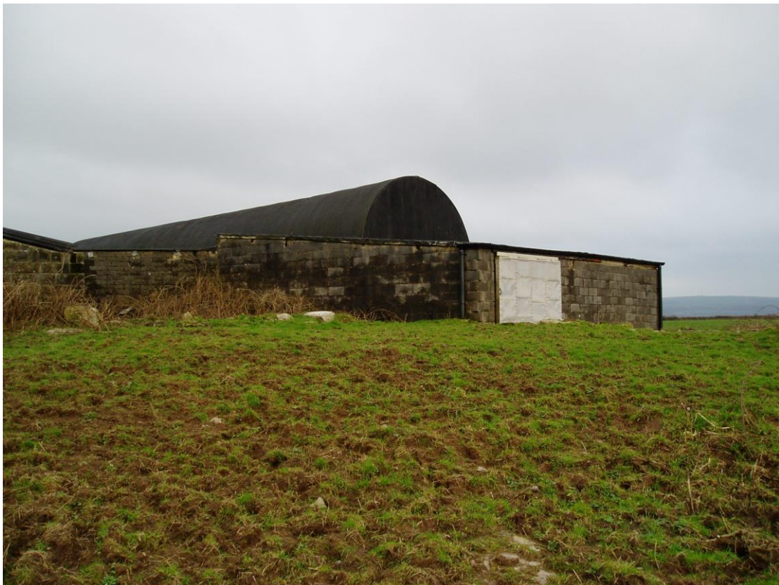
53) General View of Buildings C, D, E and J From The West
