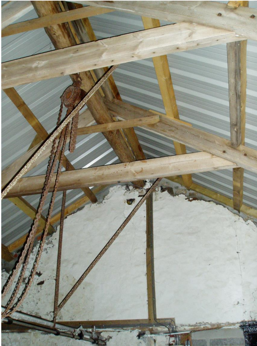
13) Interior of Milking Parlour Extension G - Roof Detail
