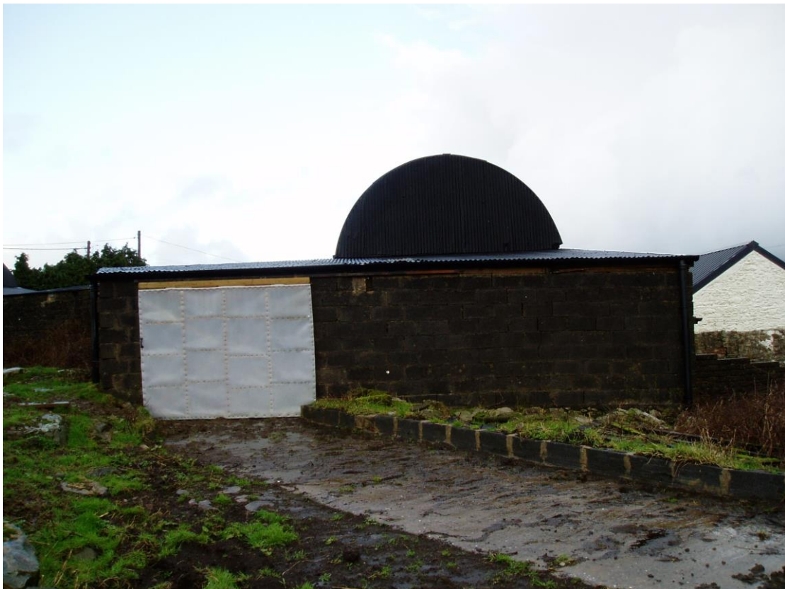
37) South West Elevation of Building J
