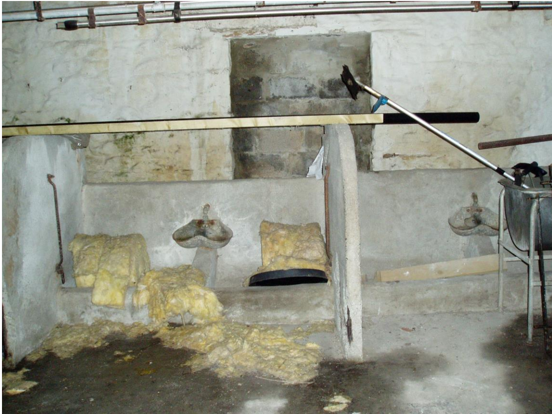
9) Interior of Milking Parlour Looking to Blocked Up Door to E
