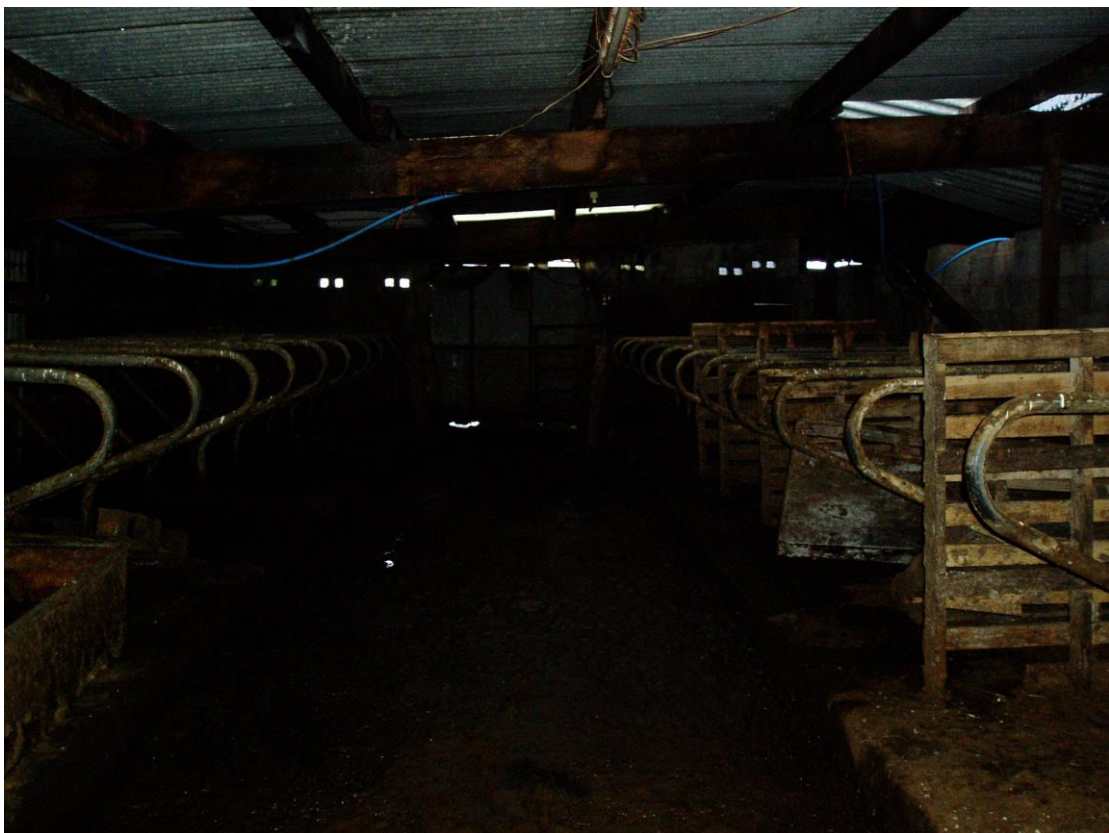
35) Interior of Building C From Building J
