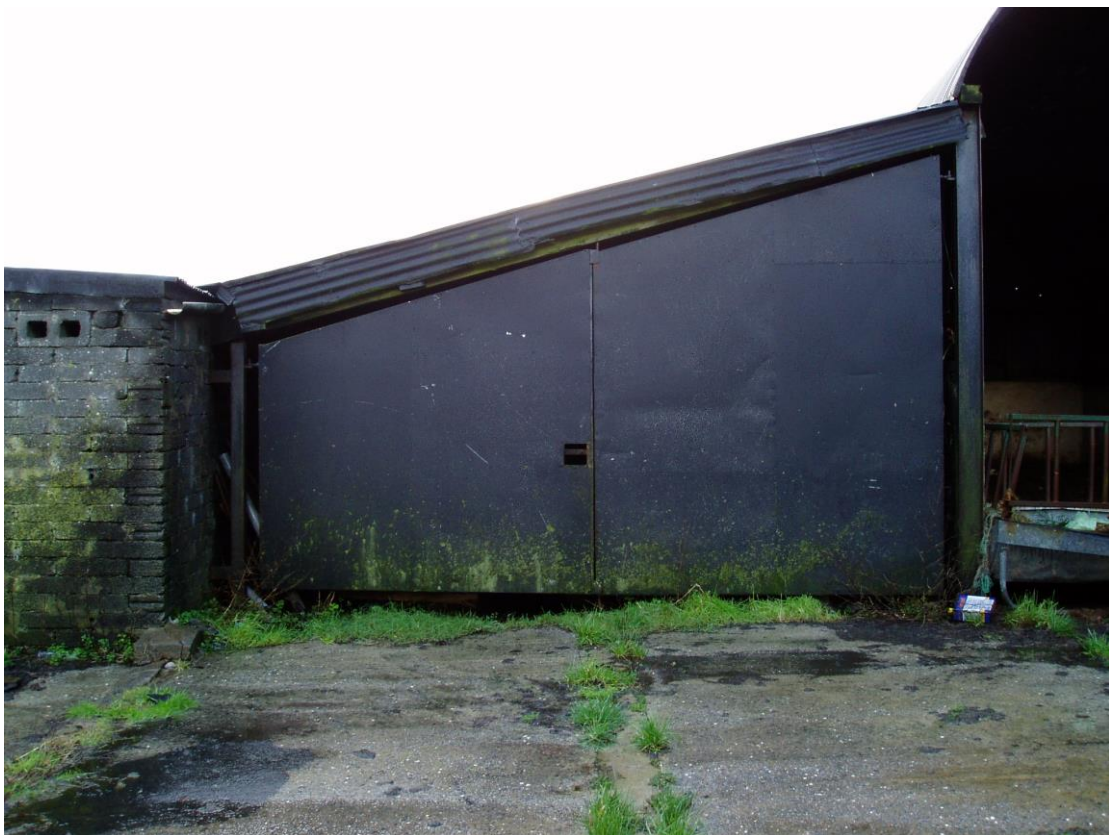
24) North East Elevation of Building B – Doors
