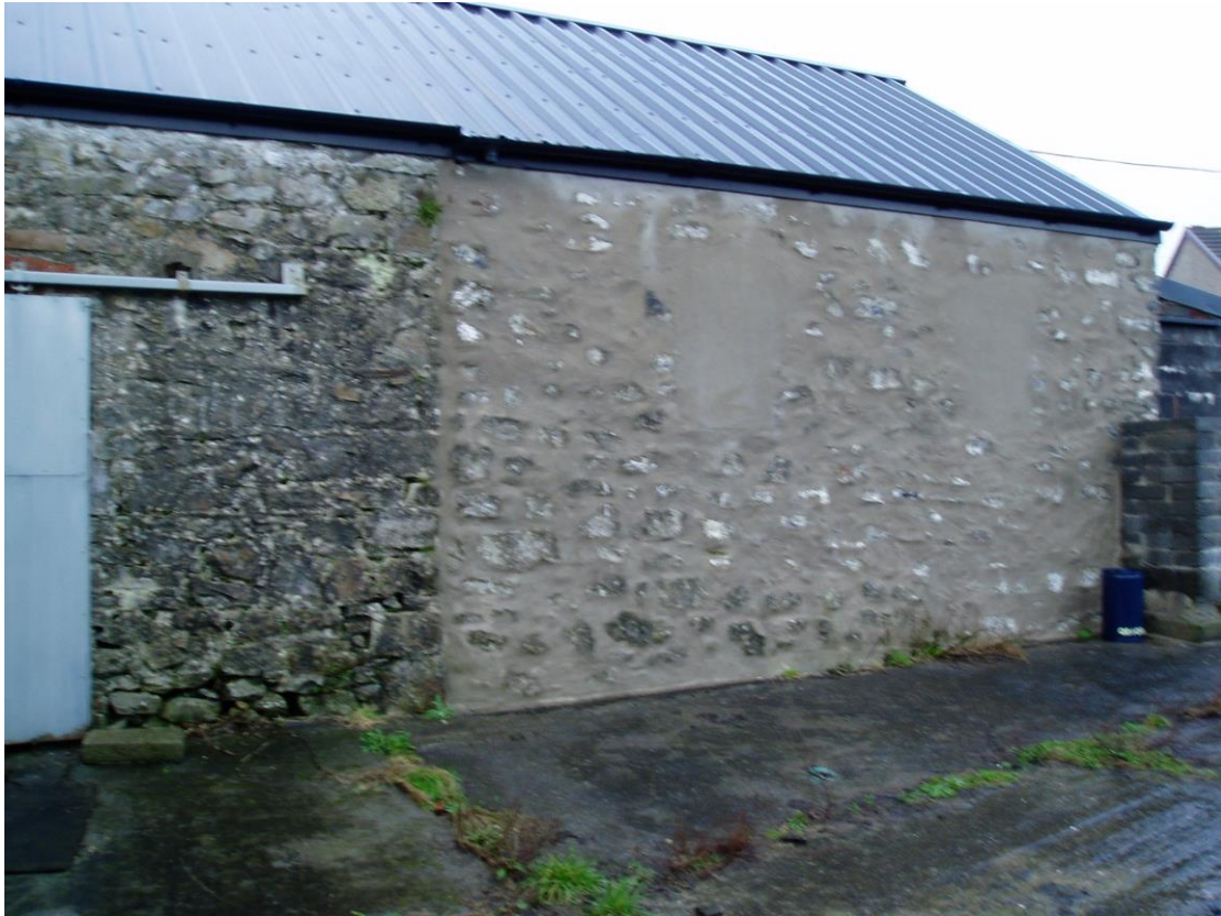
44) South East Elevation of Buildings F and G
