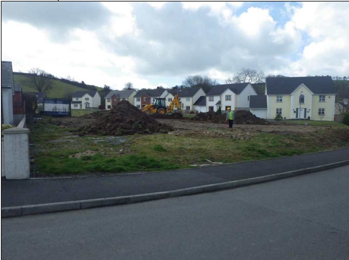
*Plate 4: LLL2013\_104, Starting clearance of topsoil in plots 1 and 2 down to subsoil looking south.*
