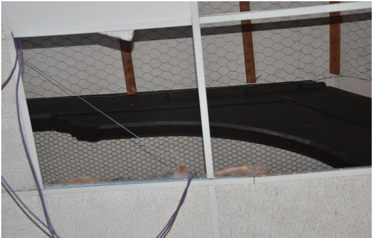
Plate 16. Central hall, original roof structure visible above later inserted dropped ceiling.
