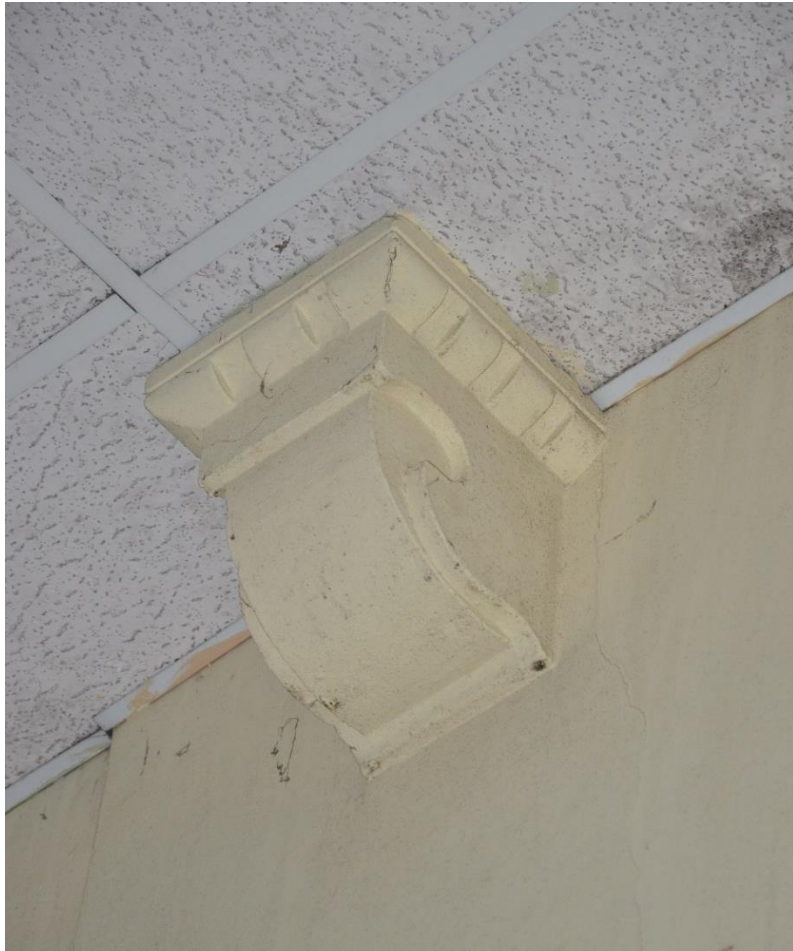
Plate 15. Central hall, surviving corbel beneath later inserted dropped ceiling.
