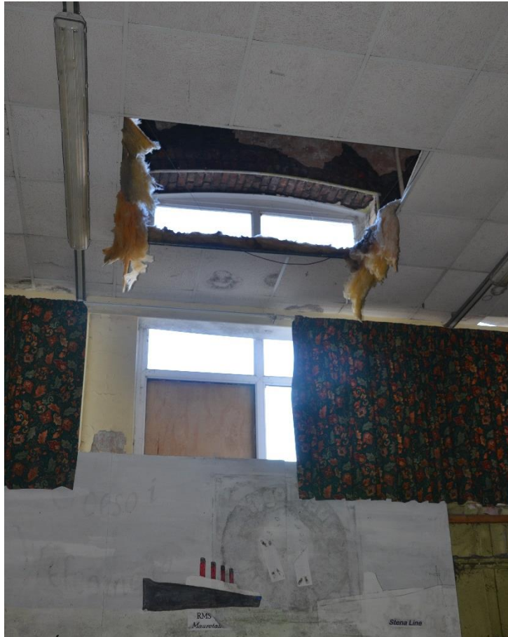
Plate 17. Classroom, showing original window truncated by later inserted dropped ceiling.
