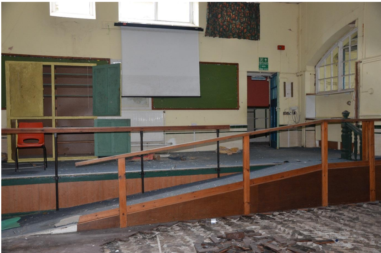
Plate 18. Central hall, west end showing addition of stage/dais and access ramp.
