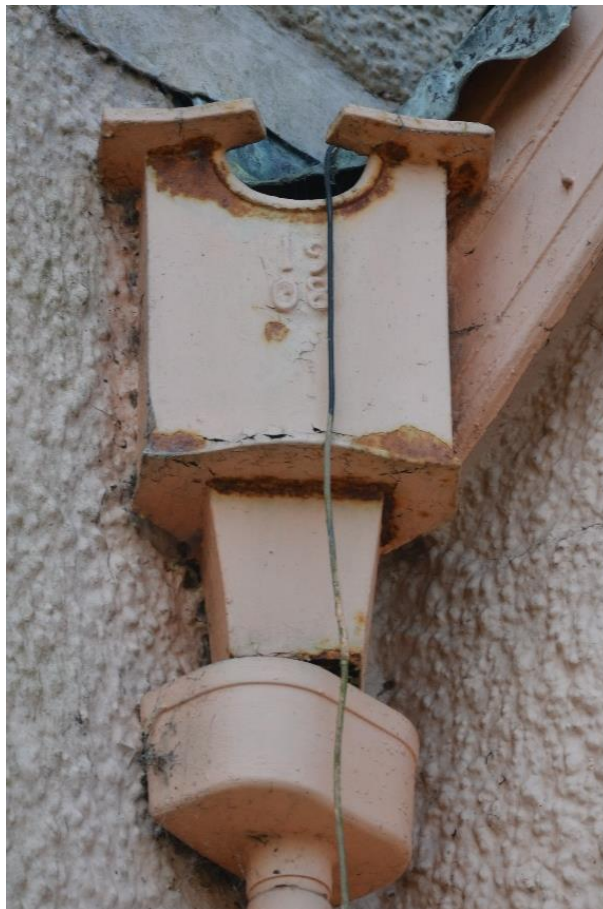
Plate 8. Detail of downpipe rainwater hopper, showing decorative date imprint
