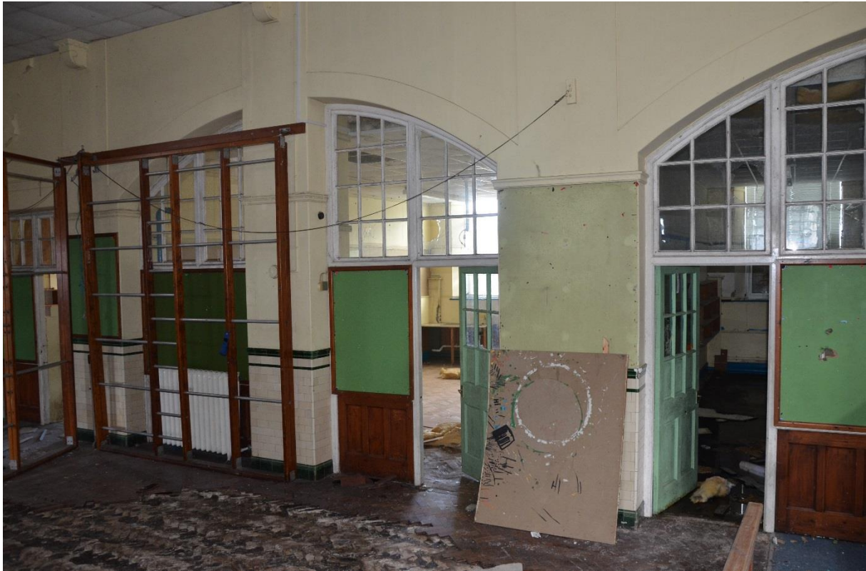
Plate 13. Central hall, showing arched windows and original timber doorframes to classrooms. Note the survival in parts of the original parquet flooring.
