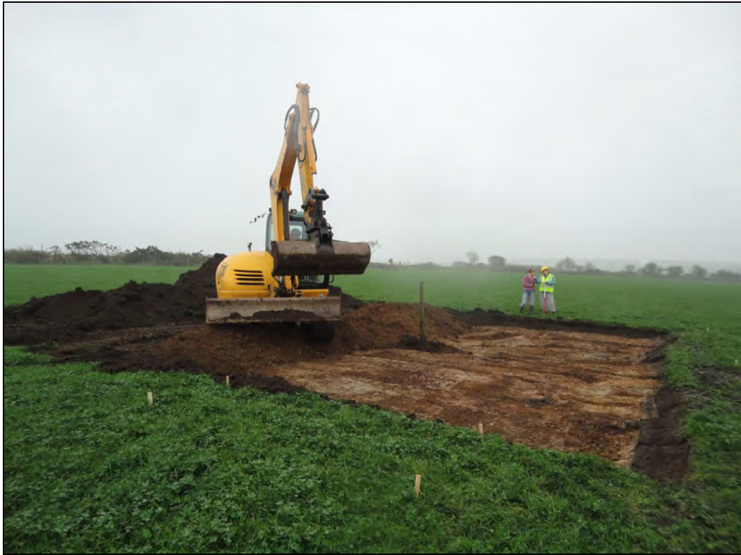
Plate 1: PGB_001, topsoil strip of western side of turbine foundation, looking southeast.
