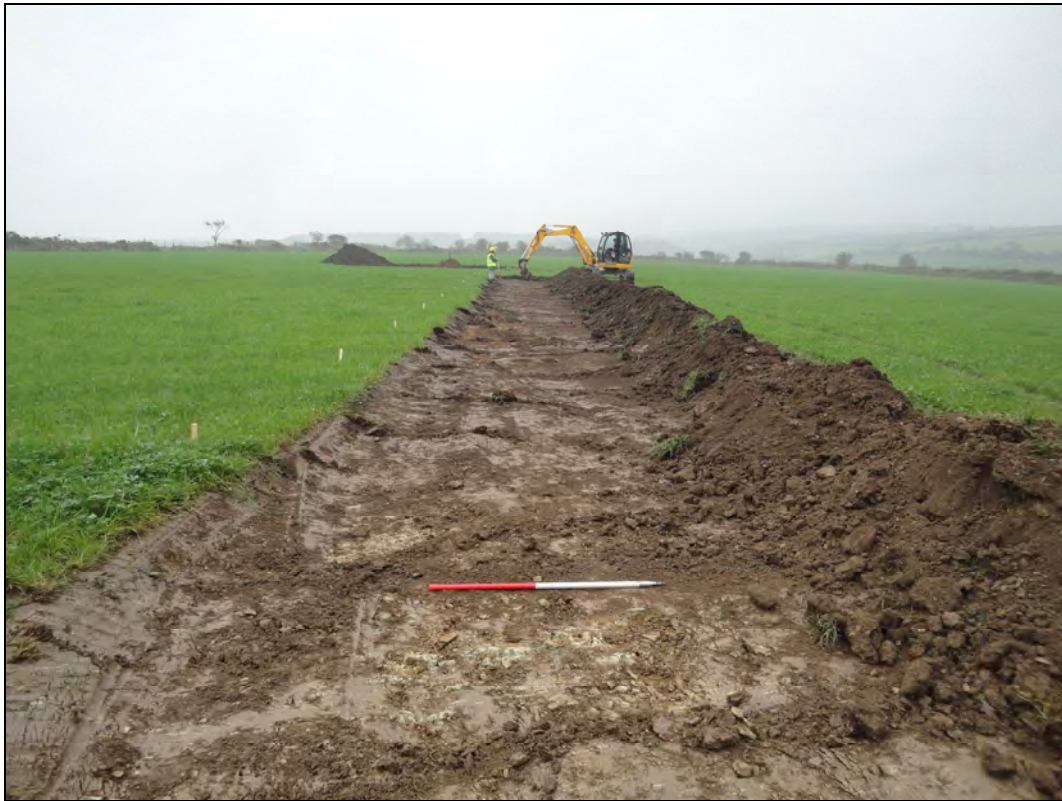
Plate 3: Partial topsoil strip along cable trench, looking south
