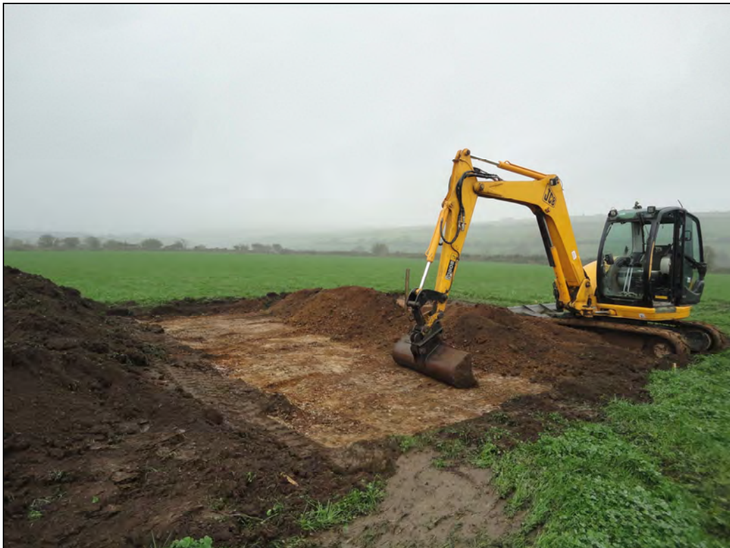
Plate 2: PGB_002, topsoil strip of eastern side of turbine foundation, looking southwest.
