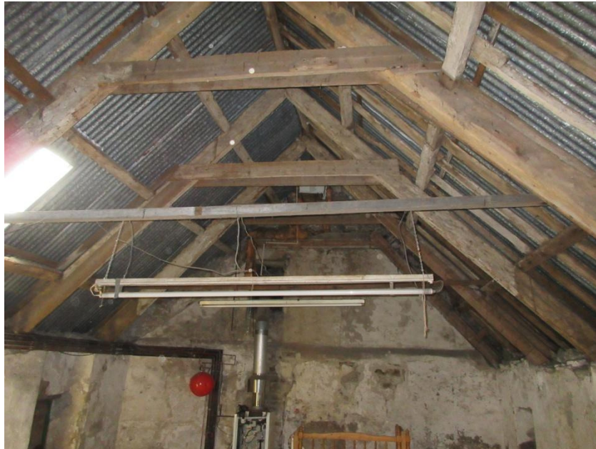
Figure 6 - early C18 roof trusses to Building 1
