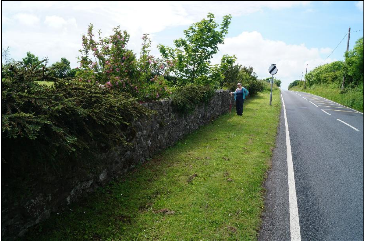
Plate 15: GGJ2016_115, stone wall, GGJ2016_015, along roadside, looking west. It appears to have been rebuilt in later 20 th century as a former gateway is not visible and concrete below part of wall.
