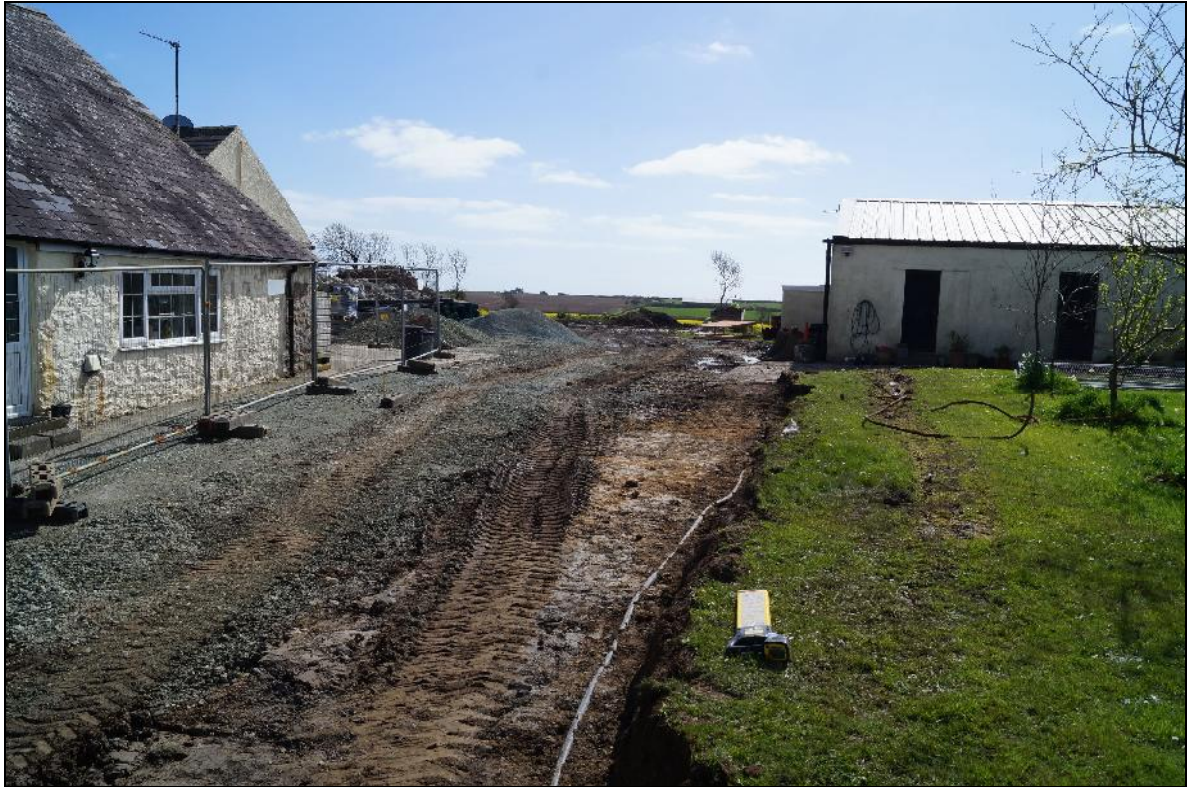
Plate 13: GGJ2016_129, Southern part of stripped area for the new roadway, showing alkathene water pipe, looking south southeast.
