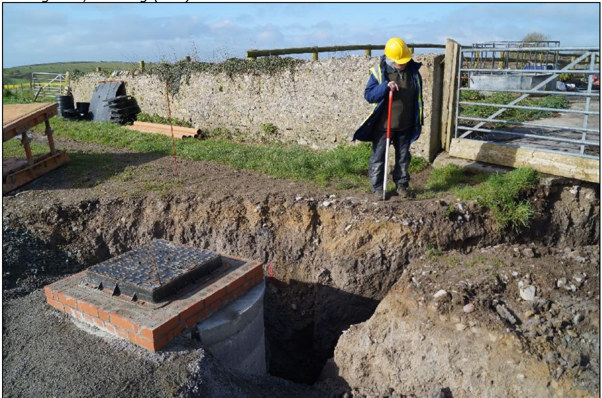
Plate 18: GGJ2016_134, Excavation for part of drainage system, showing layers of made up ground, looking southwest.
