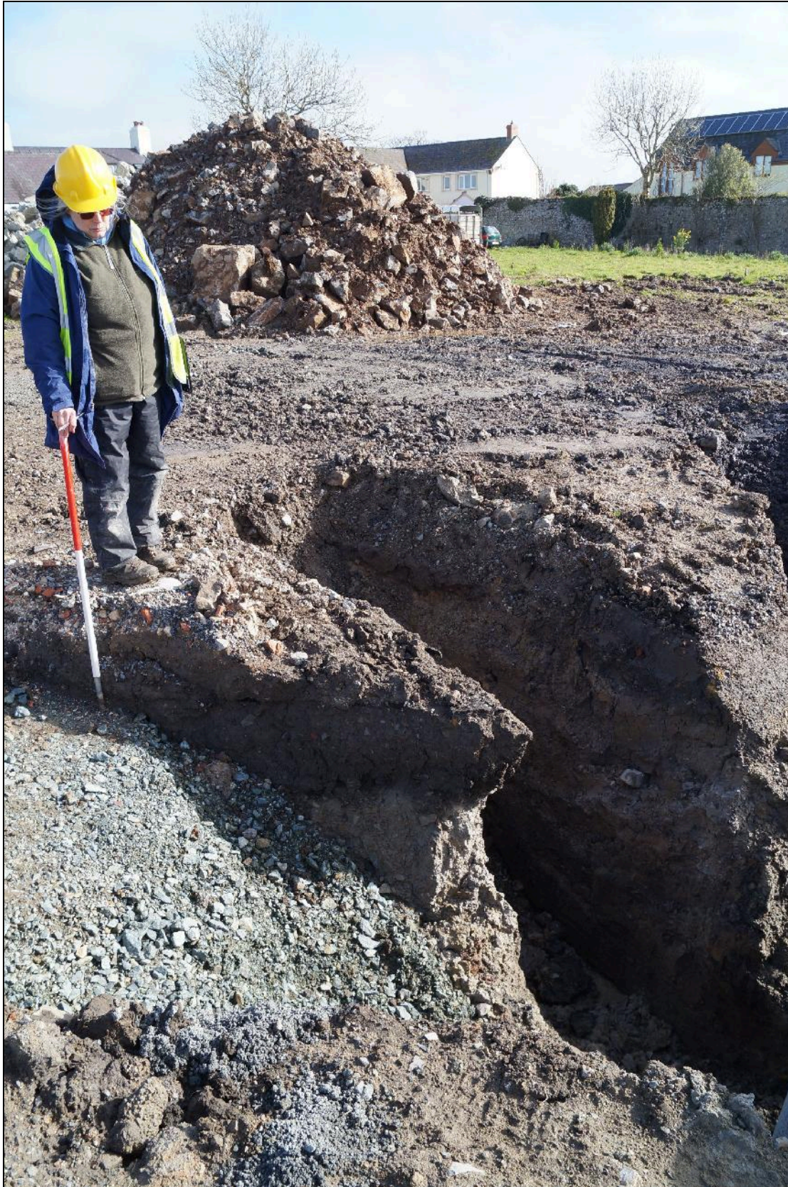
Plate 19: GGJ2016_135, Excavation for part of drainage system, showing layers of made up ground, looking northeast.
