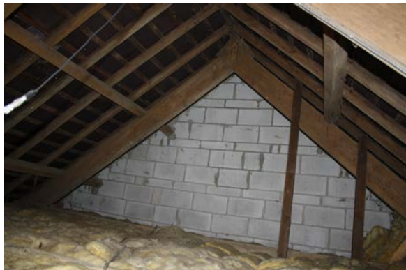
Cottage 2 Roof Space a
