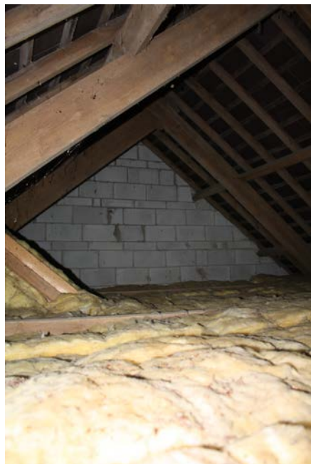
Cottage 1 Roof Space b
