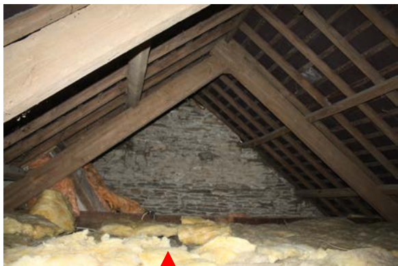
Cottage 2 Roof Space b
