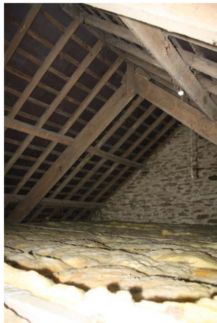
Cottage 1 Roof Space a
