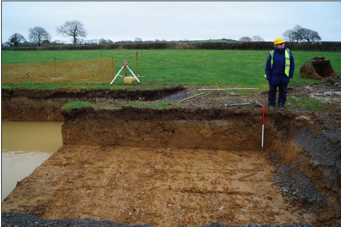
Plate 11: CCL2015_111, excavation of additional footing area to the south of the turbine foundation, with contexts 001, 005 and 007 visible in the section, looking east
