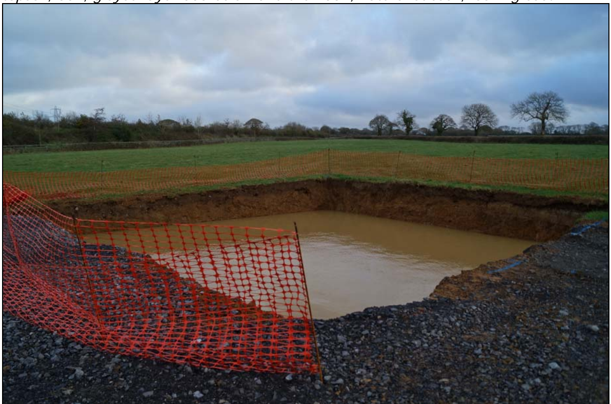
Plate10: CCL2015_110, fully excavated turbine foundation trench filled with water after heavy rain, looking northeast
