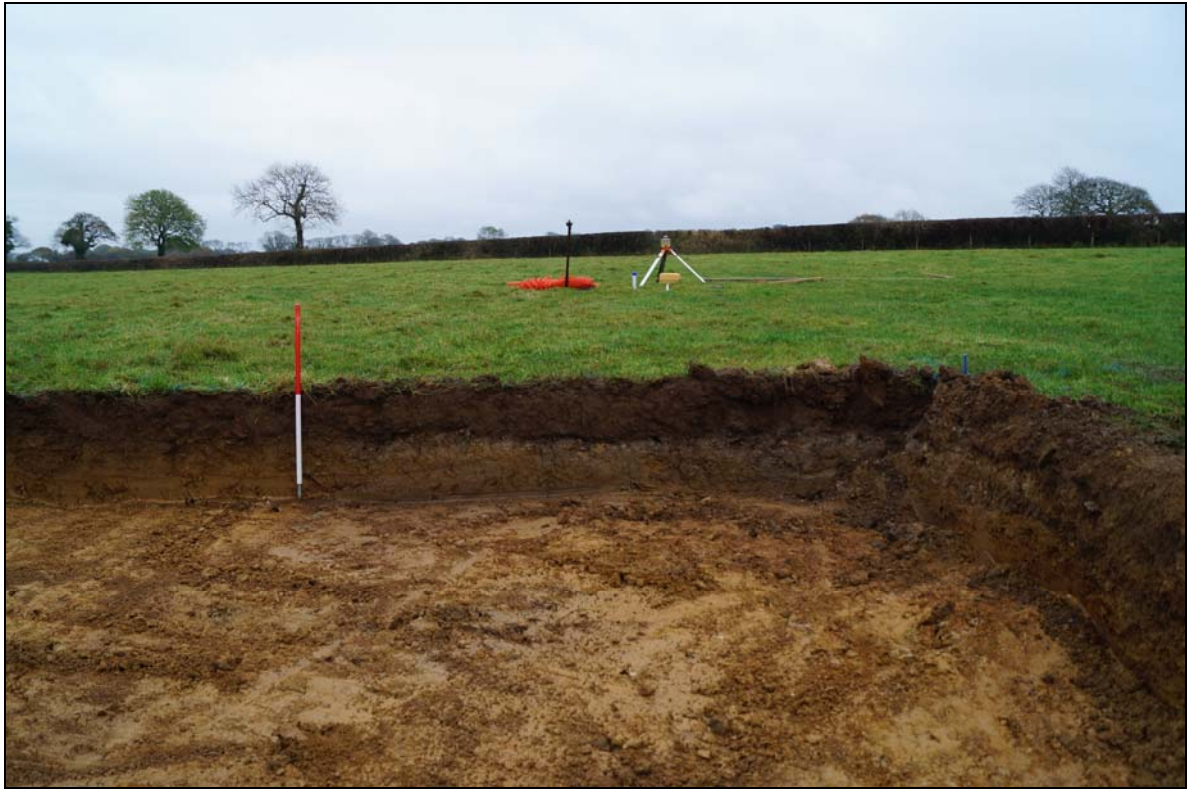
Plate 9: CCL2015_109, Southeastern corner of the turbine foundation trench showing topsoil, 001, gleyed layer 005 below and then 007, natural subsoil, looking east
