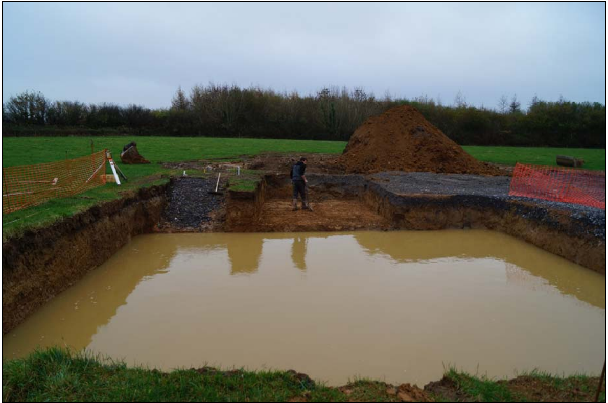
Plate 13: CCL2015_113, excavated turbine foundation and ramp and additional footing to the south, looking south.
