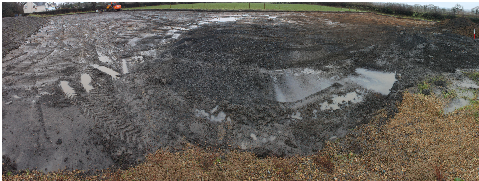
Plate 1 - Overview of stripped area.
