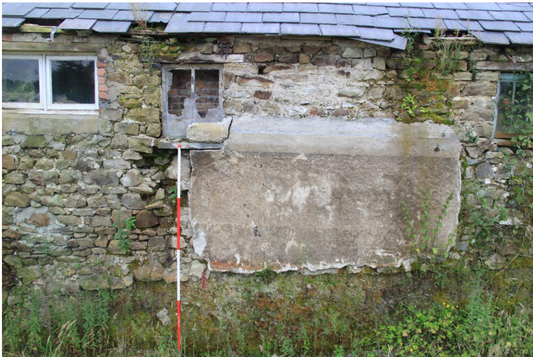
AD025_022 - Farmhouse - Patch of Plasterwork Demonstrating Existence Former Lean-to - North Elevation
