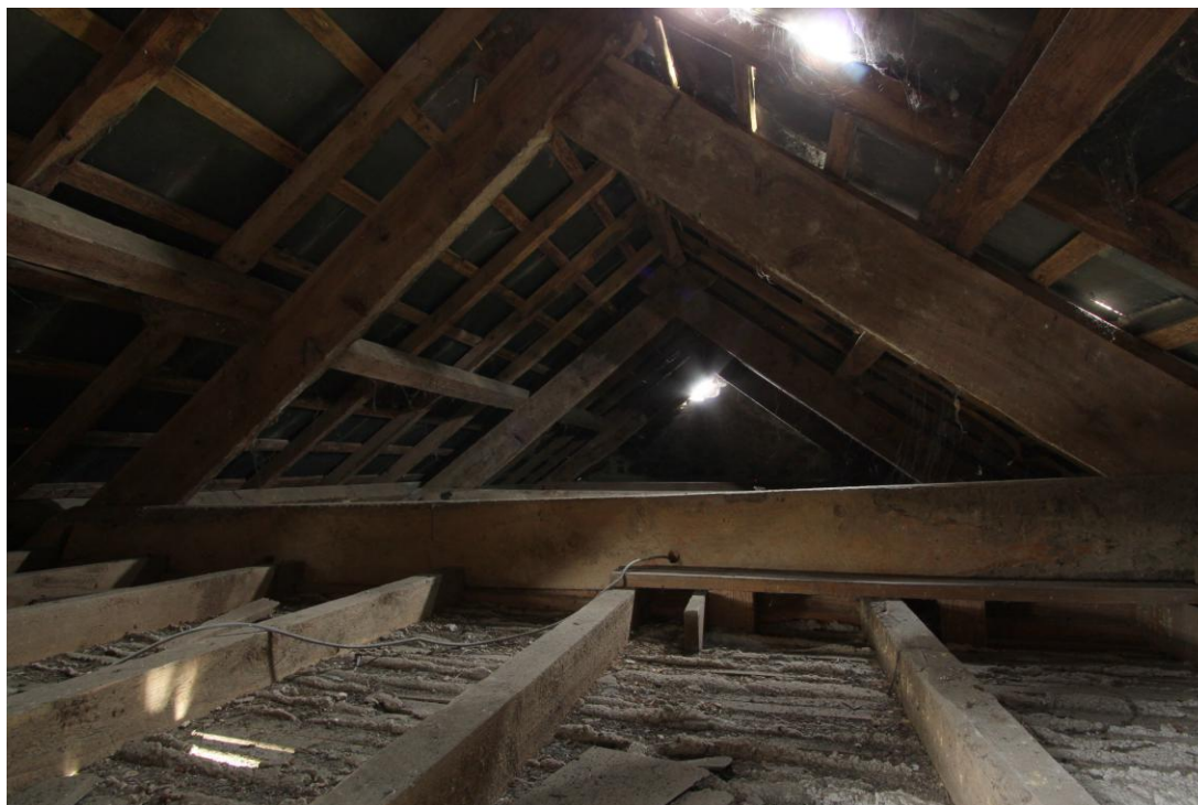
AD025_062 - Farmhouse - Truss , Purlins & Common Rafters - Loft Space
