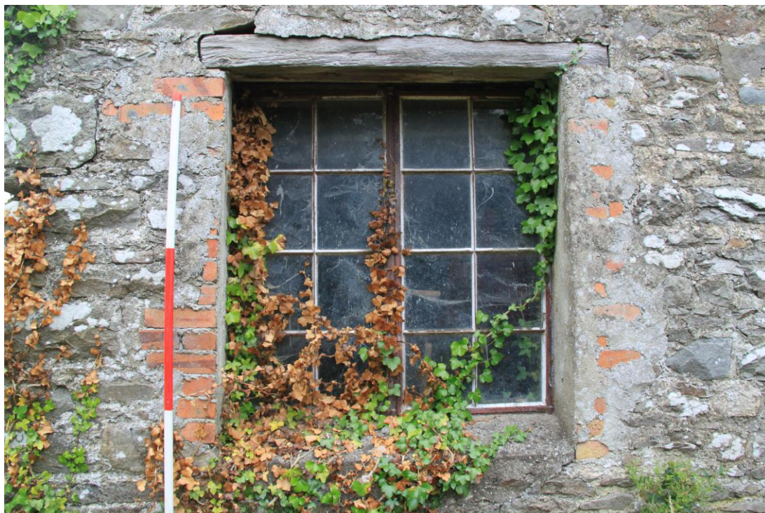
AD025_028 - Cowshed - Inserted Crittall Window - East Elevation
