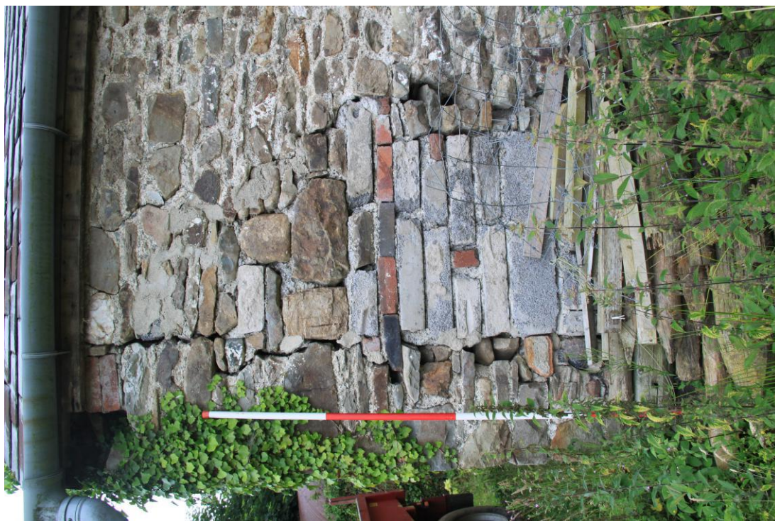
AD025_027 - Cowshed - Repair Infill - North Elevation
