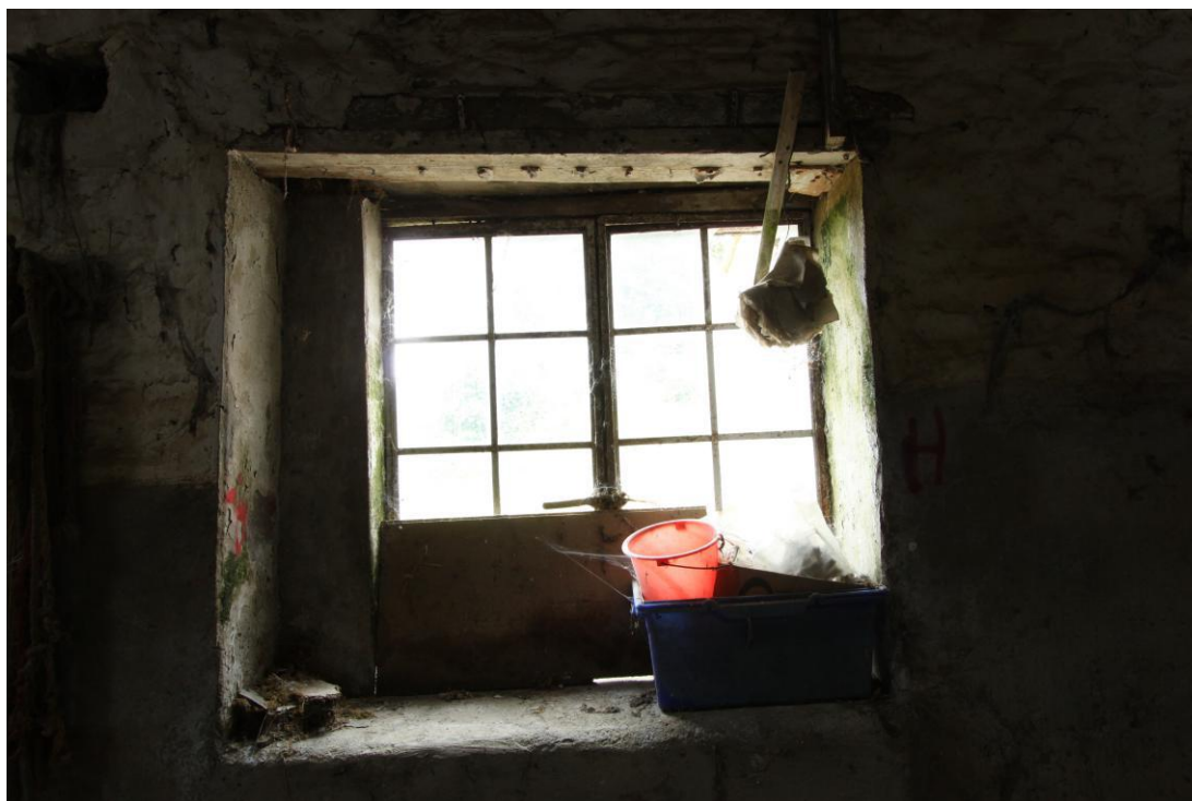
AD025_079 - Cowshed - Internal View of Crittall Window
