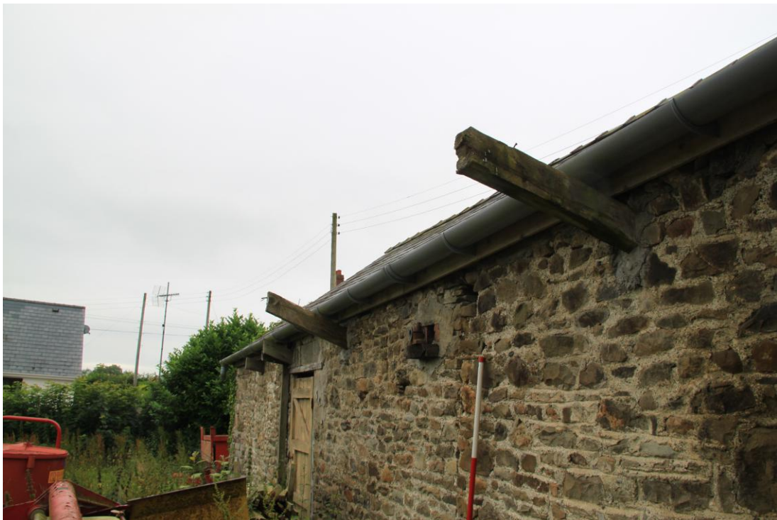
AD025_026 - Cowshed - Remains of Principle Rafters - North Elevation
