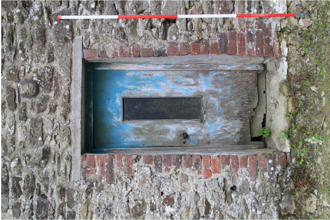
AD025_021 - Farmhouse - Inserted Door to Rear Room - West Elevation
