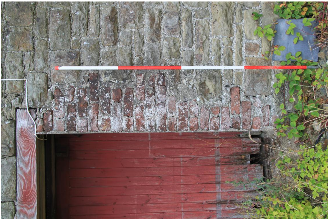
AD025_020 - Farmhouse - Inserted Red Brick Door Reveal - South Elevation
