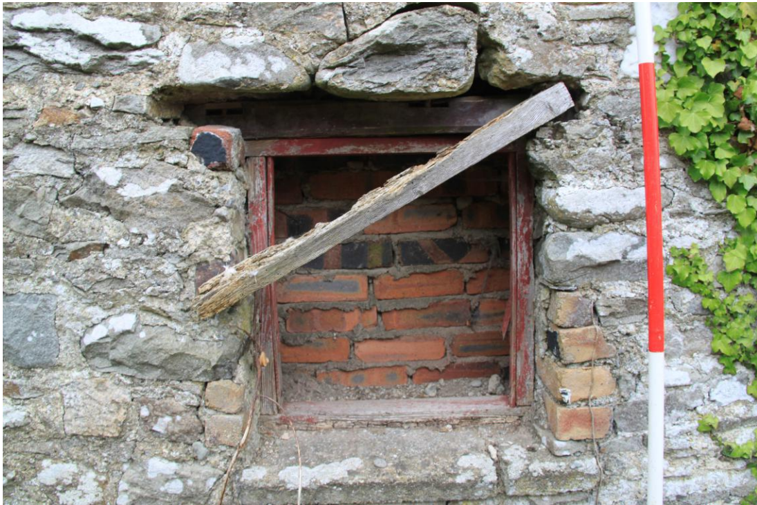
AD025_029 - Cowshed - Repaired & Filled Window - East Elevation
