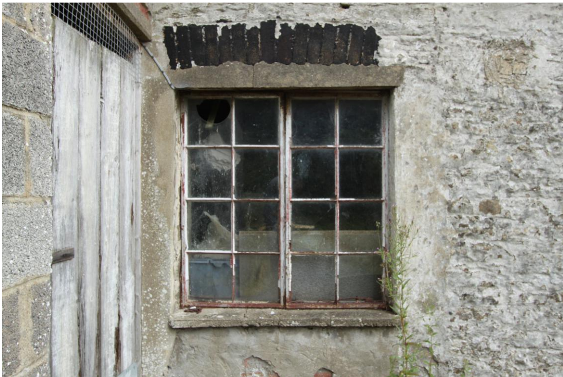
AD025_030 - Cowshed - Inserted Crittall Window - South Elevation
