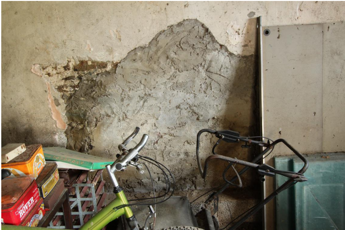
AD025_044 - Farmhouse - Blocked Fireplace - Bay III - Ground Floor
