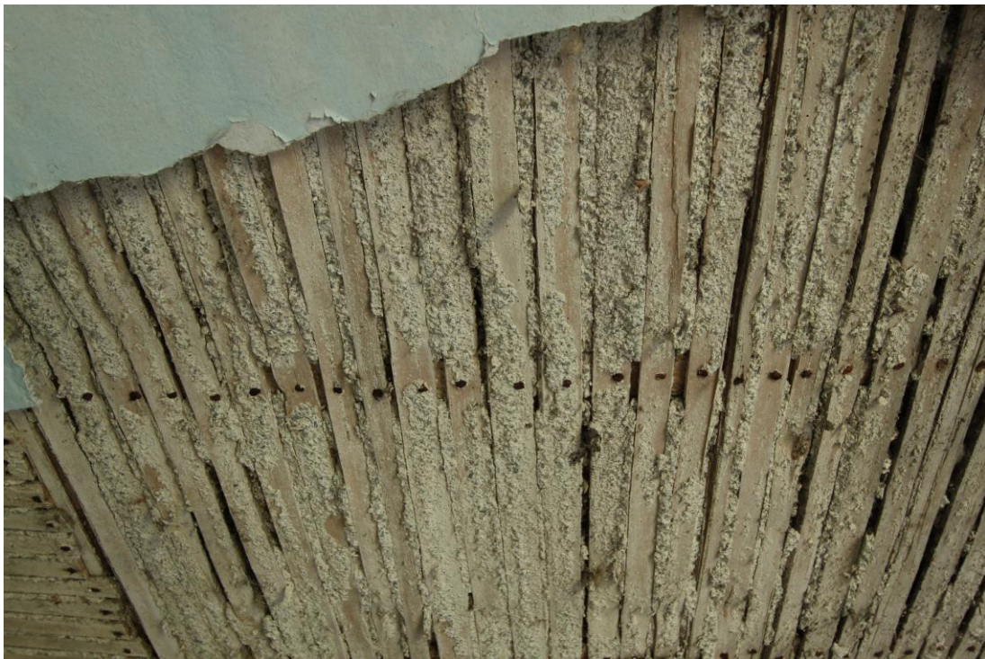
AD025_054 - Farmhouse - Lathe & Plaster - Bay I - First Floor
