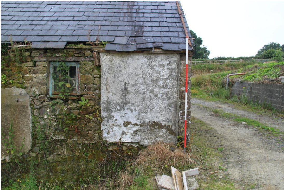
AD025_023 - AD025_022 - Farmhouse - Patch of Plasterwork Demonstrating Existence Former Lean-to - North Elevation
