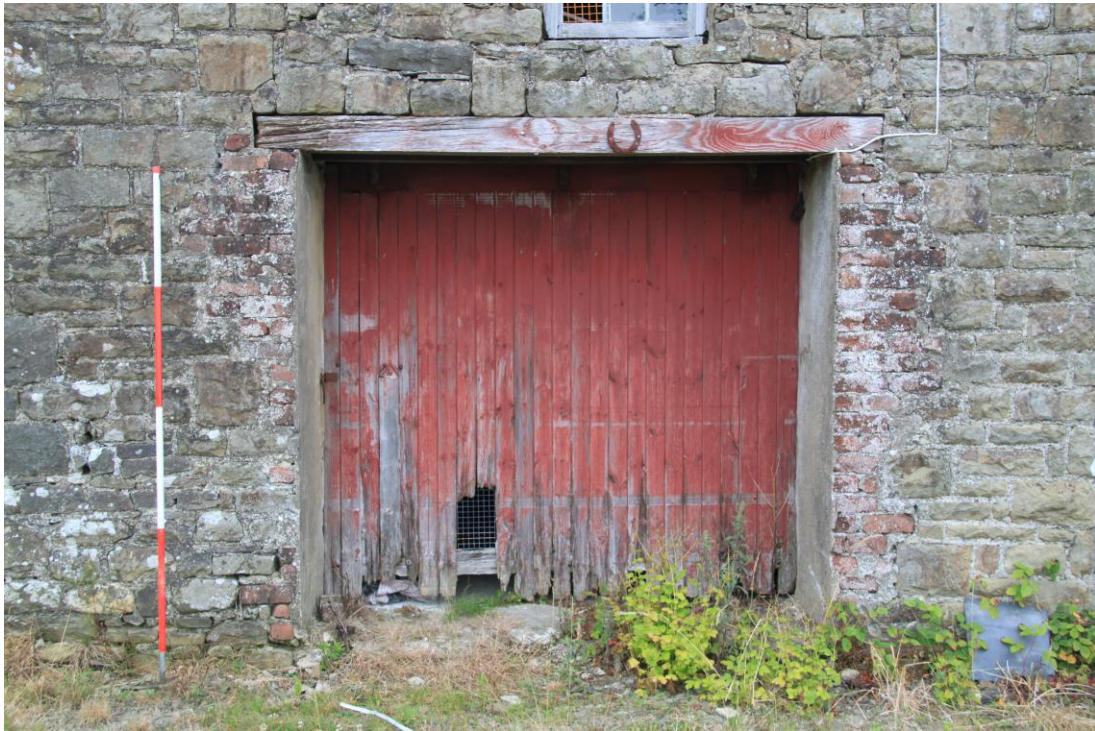
AD025_019 - Farmhouse - Inserted Garage Door - South Elevation
