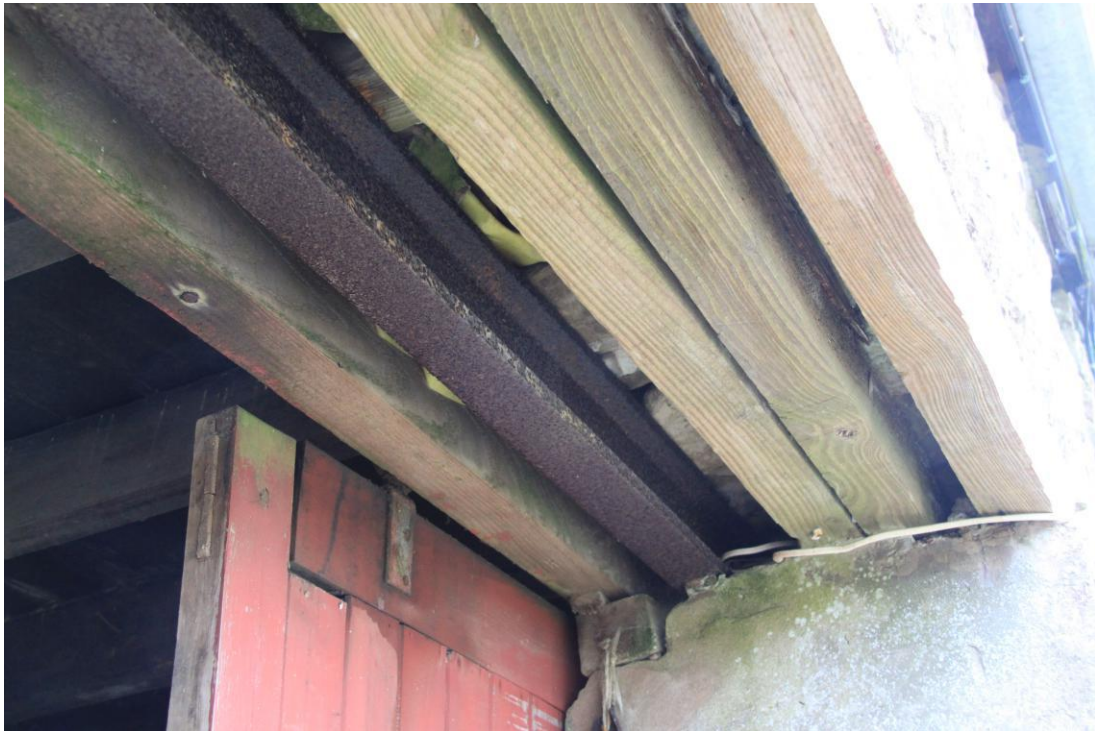
AD025_035 - Farmhouse - Garage Door Lintels, inc. Railway Track
