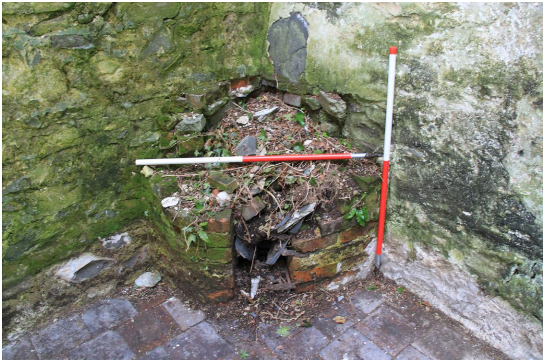
Plate 38 - AD010-BR-038 - Remains of small boiler/copper.
