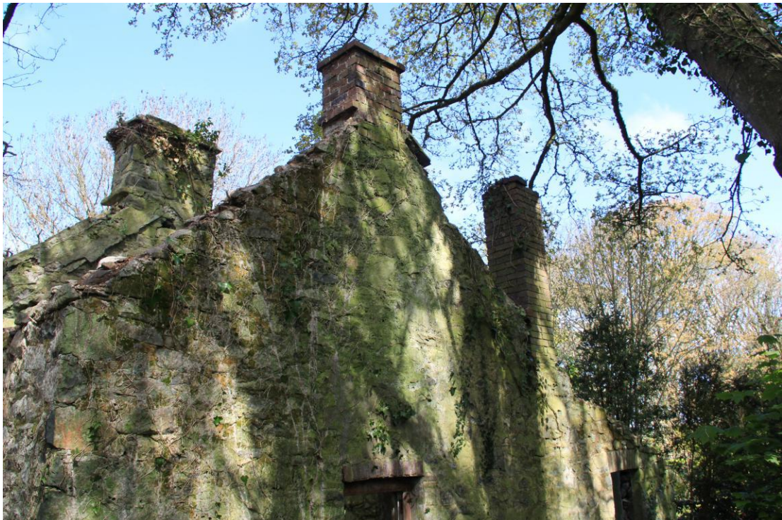
Plate 6 - AD010-BR-006 - East elevation, upper section.
