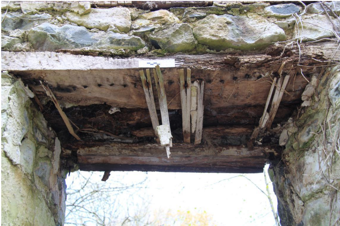
Plate 17 - AD010-BR-017 - Oak window lintel, internal, north wall.
