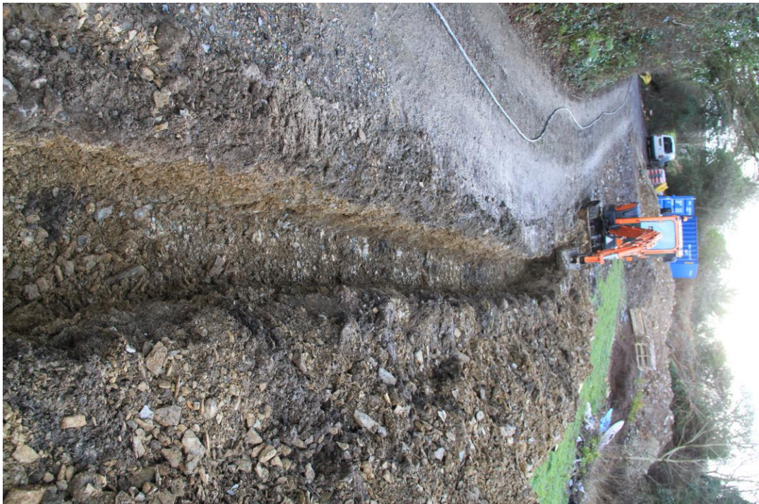
Plate 59 - AD010-D2-012 - Service trench 1 extending along track.
