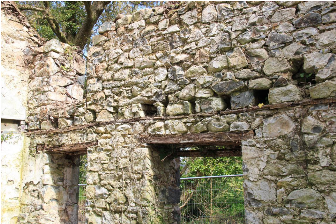
Plate 18 - AD010-BR-018 - Joist sockets, internal, north wall.
