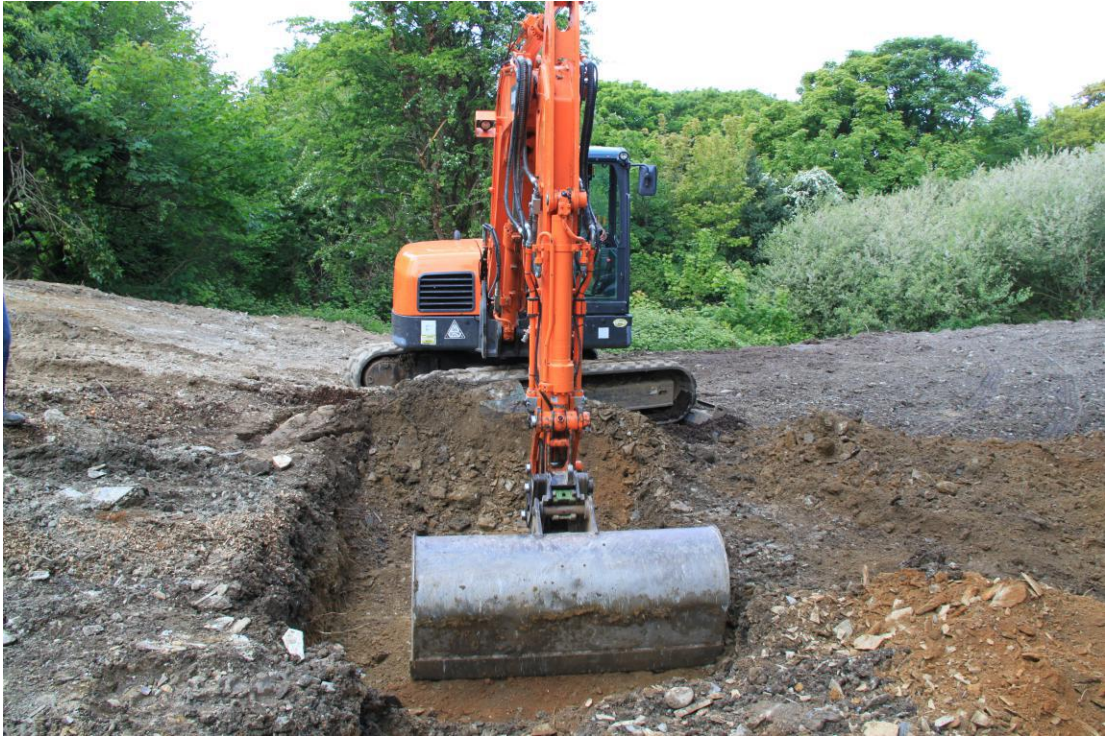
Plate 66 - AD010-D3-019 - Excavation of septic tank pit.
