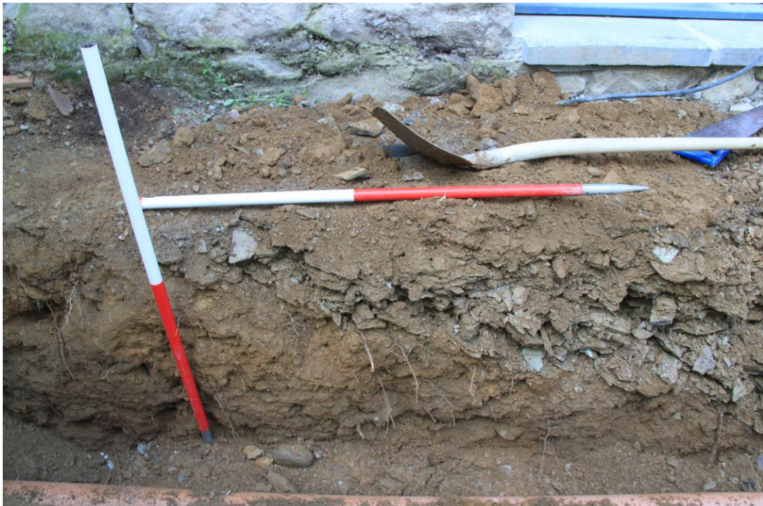
Plate 65 - AD010-D3-018 - Service trench 2 in front of the Former Coach House showing layers of levelling - shale over clayey-loam.
