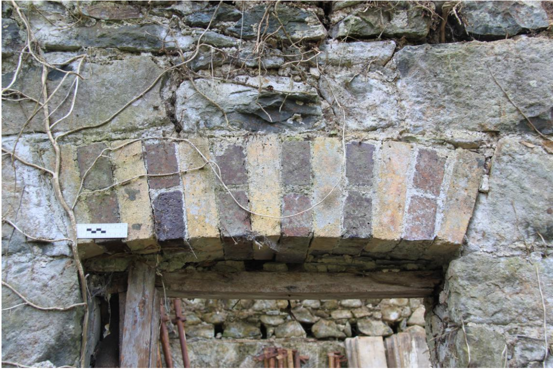
Plate 13 - AD010-BR-013 - Yellow and red brick flat segmental arch to window head, north elevation.
