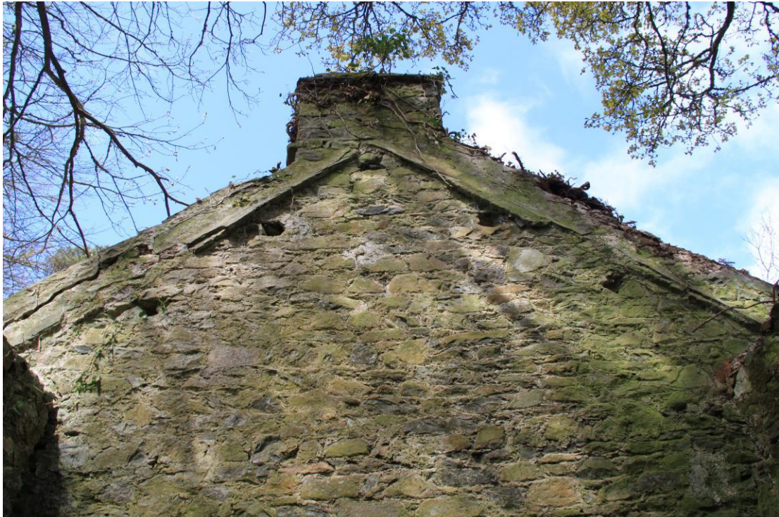
Plate 44 - AD010-BR-044 - Gable wall between Former Coach House and Extension A, showing two purlin and one ridge sockets.
