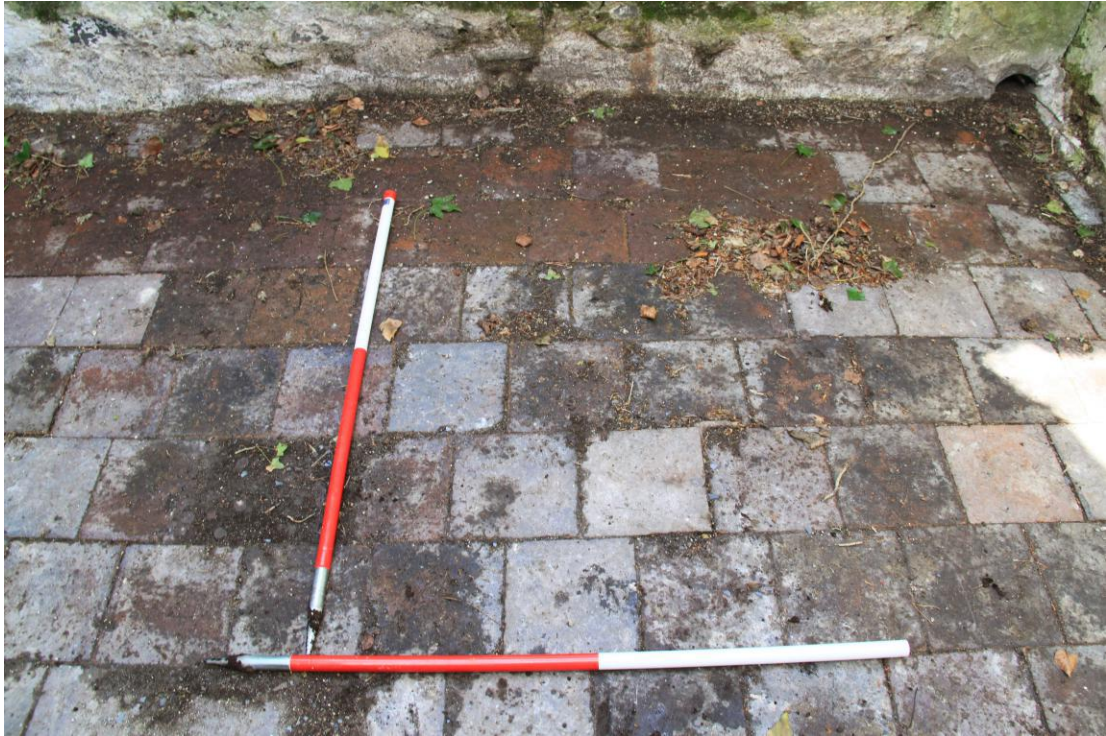
Plate 37 - AD010-BR-037 - Quarry tile floor to Extension A.
