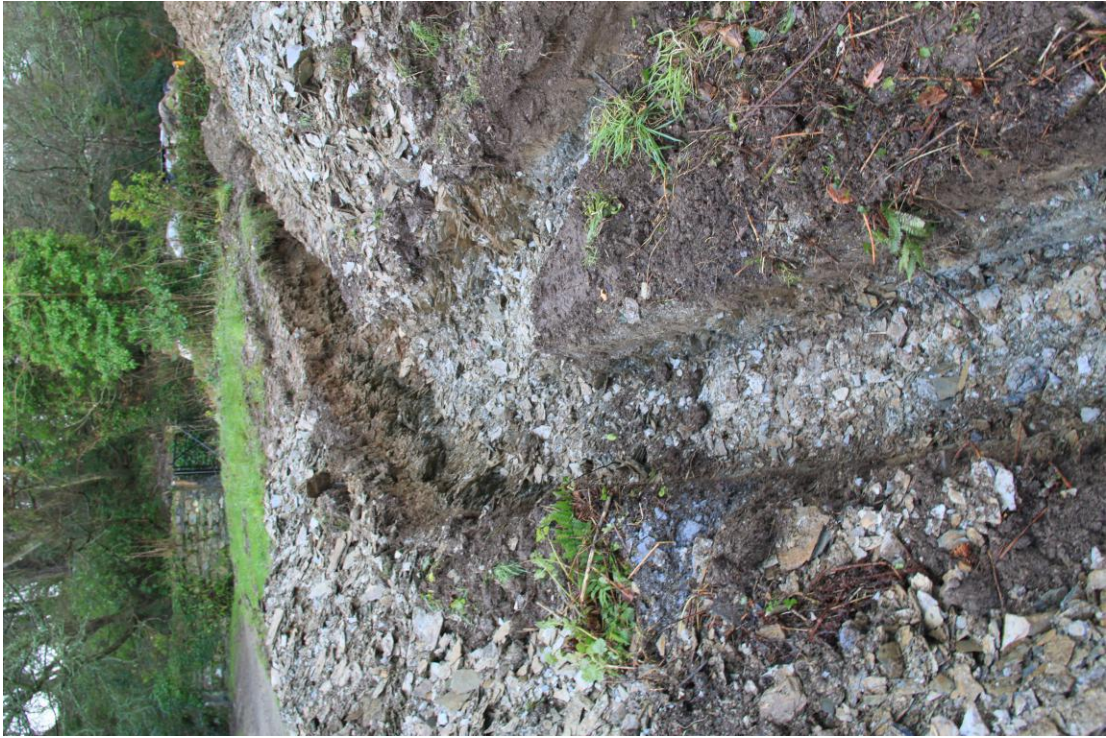
Plate 52 - AD010-D1-005 - Service trench 1 passing Castle Mill.
