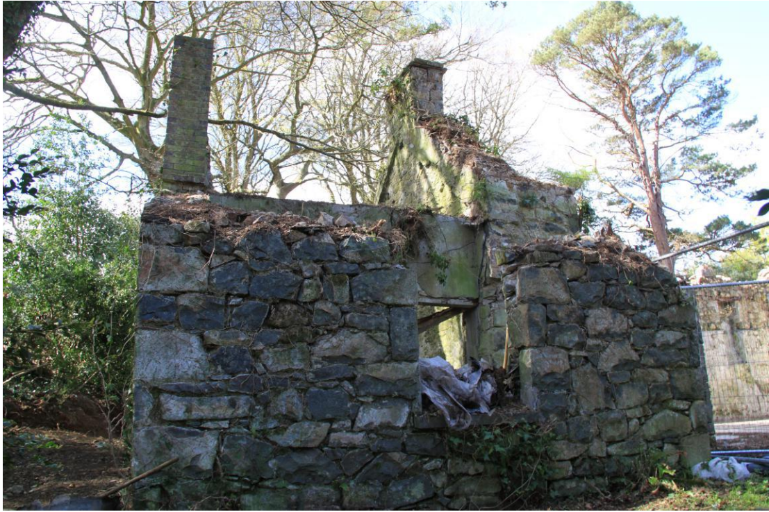
Plate 9 - AD010-BR-009 - North elevation, east end.
