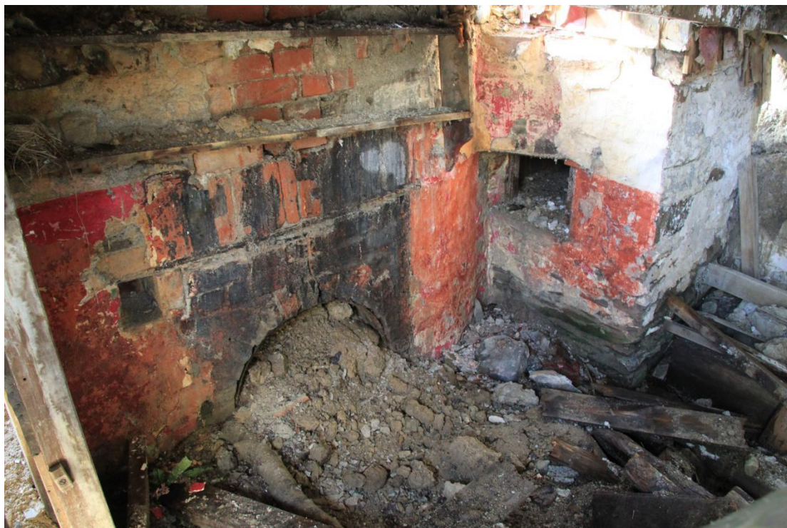
Plate 30 - AD004-BR-030 - Brick fireplace and bread oven.
