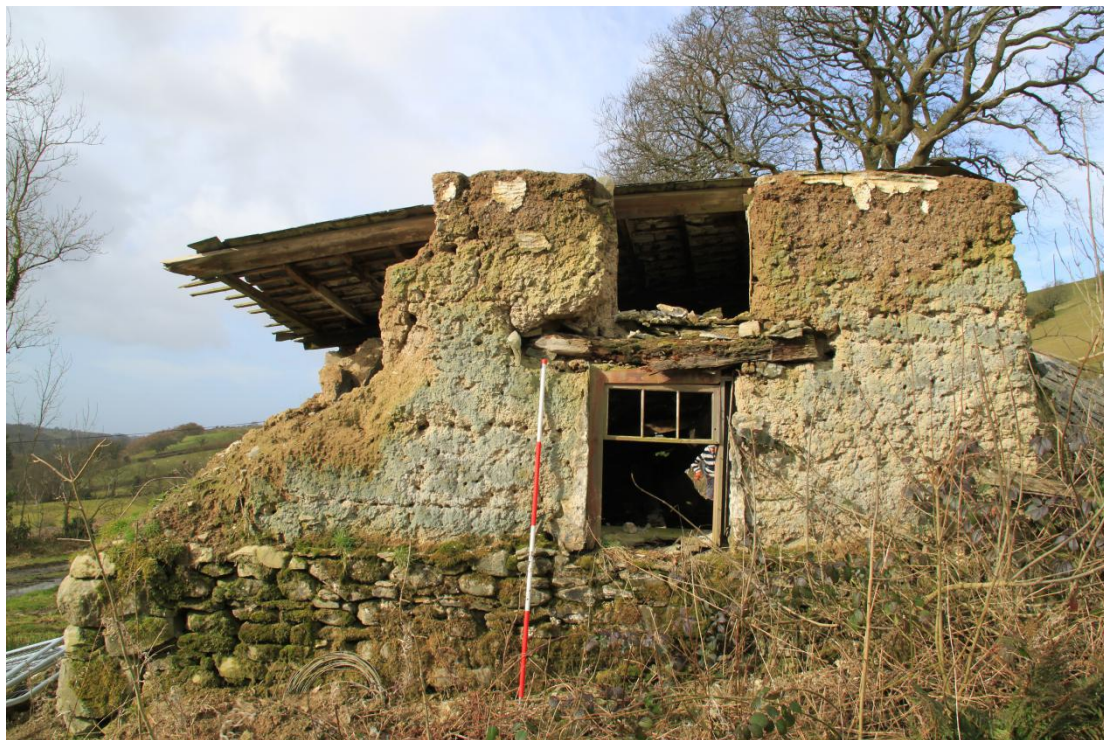
Plate 3 - AD004-BR-003 - View of west elevation. N.B. the change in clom colour to top of wall.
