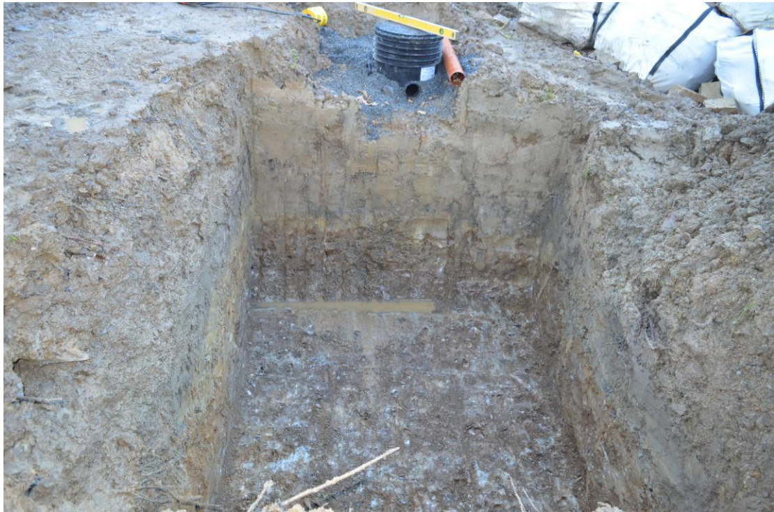
Plate 97 - AD004-D5-097 - Excavation of septic tank trench, looking east.
