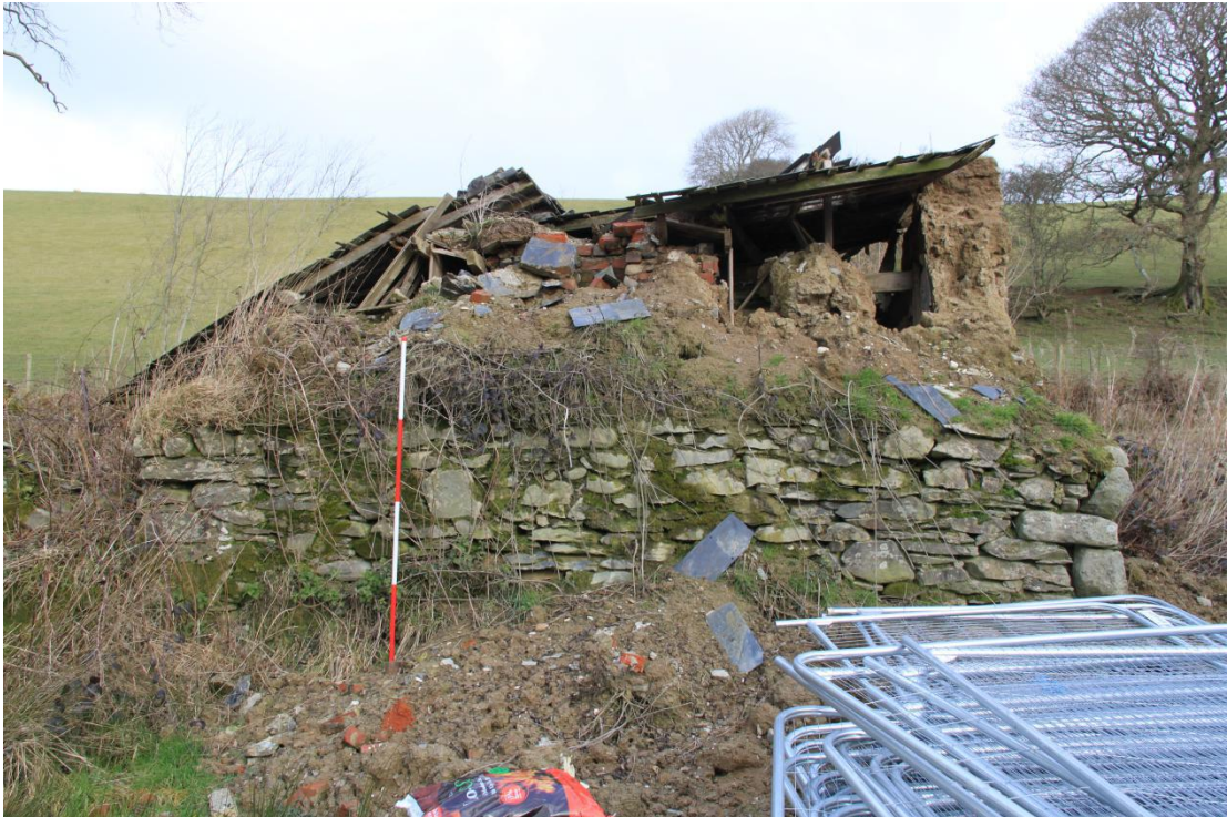
Plate 10 - AD004-BR-010 - South elevation, showing stone platform and decayed clom gable.
