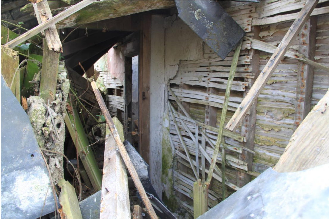
Plate 35 - AD004-BR-035 - Passage side of kitchen partition, in lathe and plaster.
