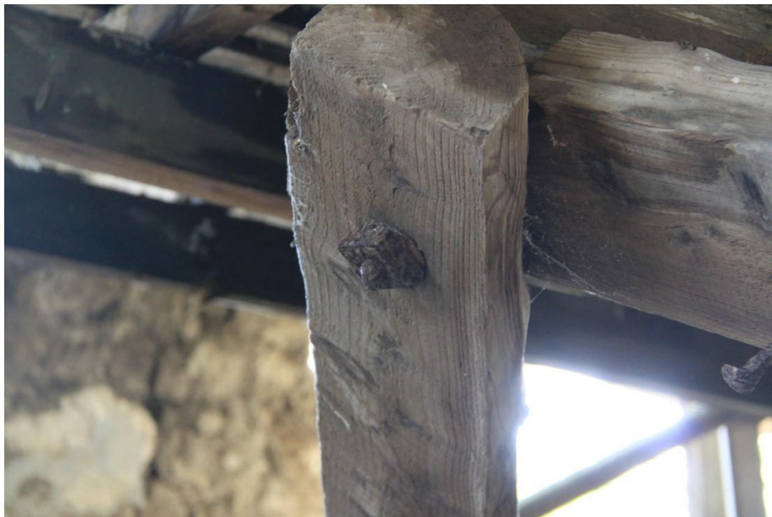
Plate 39 - AD004-BR-039 - Nut and bolt fixing to apex of principle rafters.
