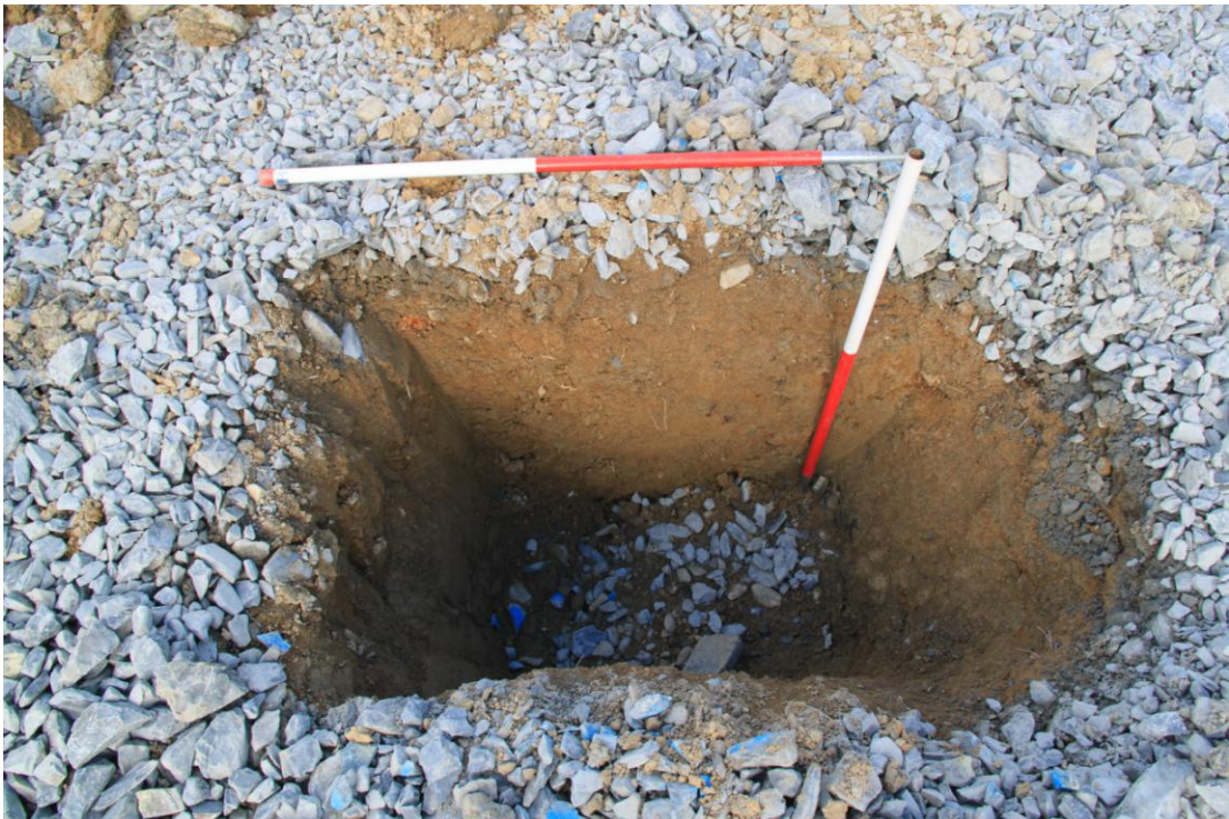
Plate 79 - AD004-D3-079 - Foundation pit, for steel post.
