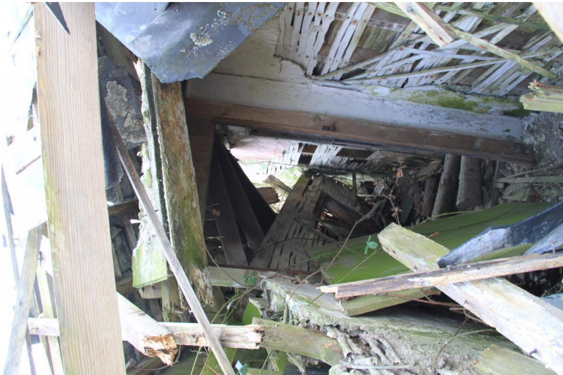
Plate 36 - AD004-BR-036 - Passage side of kitchen partition, in lathe and plaster, also showing parlour partition in woven hazel and clom.
