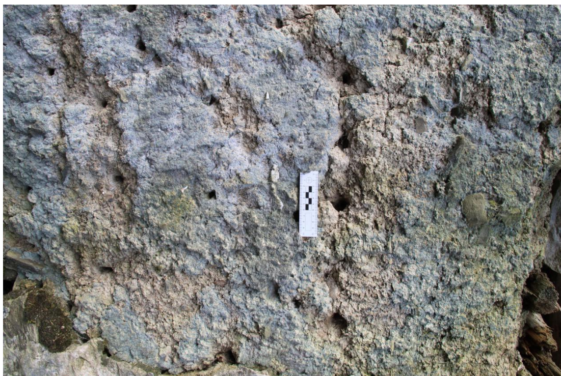
Plate 24 - AD004-BR-024 - Detail of 'pug holes' to support the adherence of render, east elevation.
