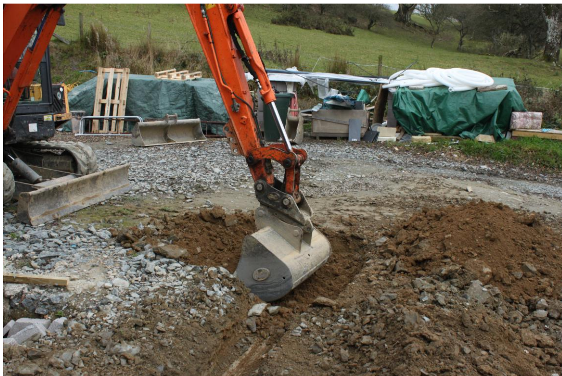
Plate 82 - AD005-D4-082 - Excavation of waste service trench, east end of site.
