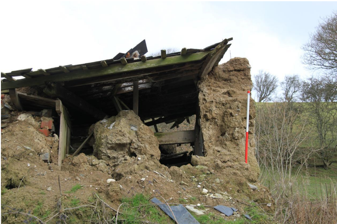
Plate 22 - AD004-BR-022 - Section of east lateral wall, showing difference in upper clom composition and lower.
