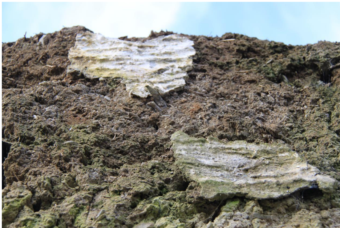
Plate 25 - AD004-BR-025 - Remains of thin lime render.
