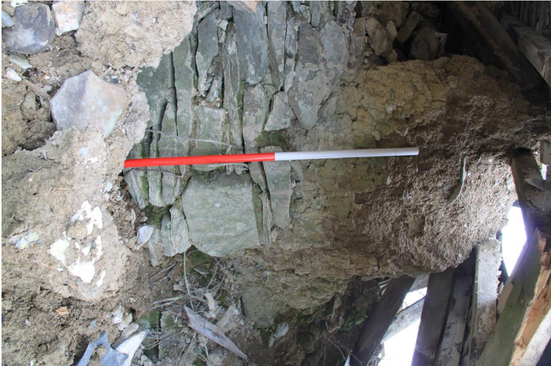
Plate 15 - AD004-BR-015 - Joint between later stone infill and clom wall to former kitchen doorway.
