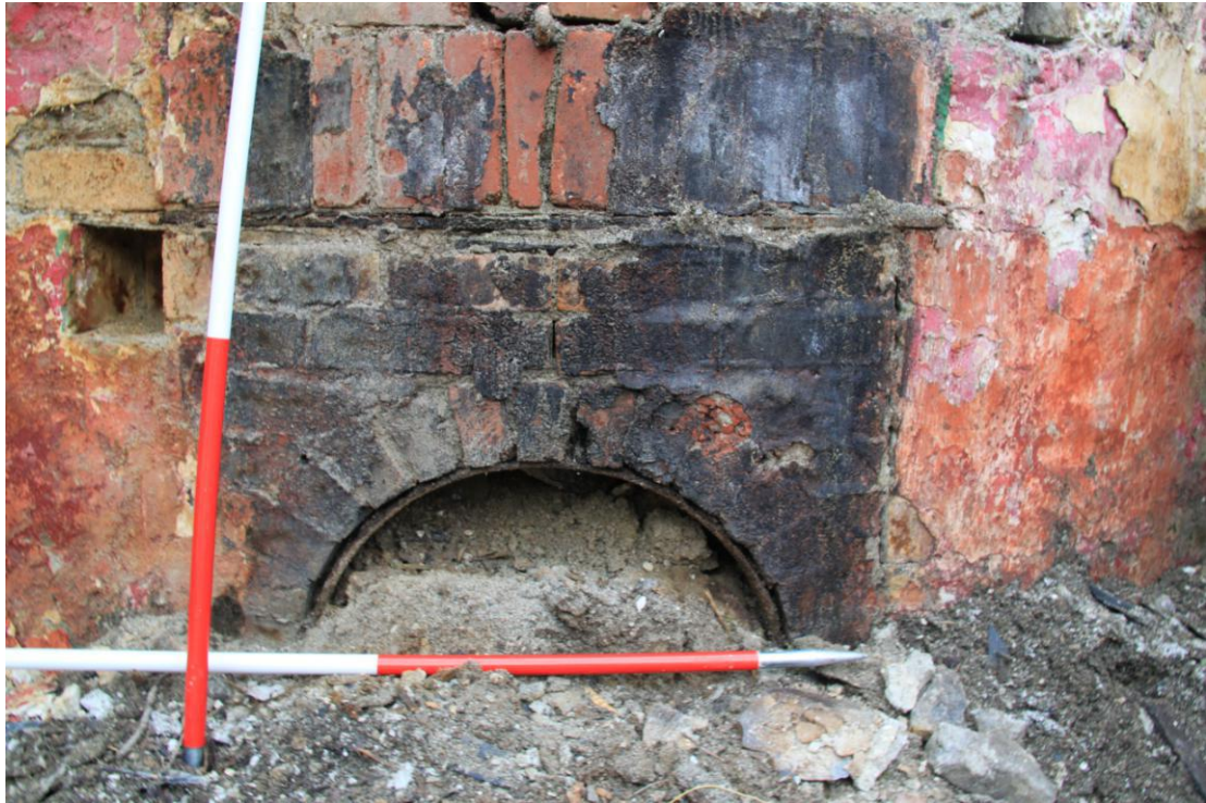
Plate 46 - AD004-D1-046 - Fireplace; black painted bricks a later infill.
