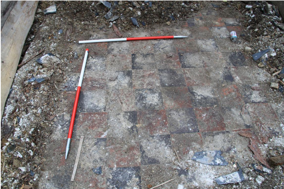
Plate 45 - AD004-D1-045 - Black and red quarry tile floor to kitchen.
