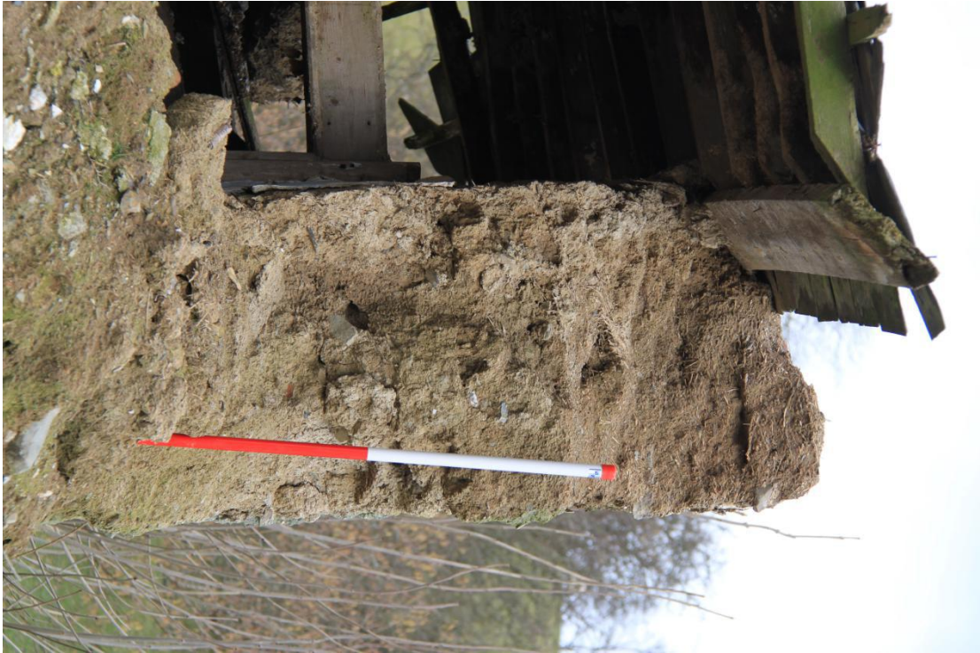
Plate 21 - AD004-BR-021 - Section of east lateral wall, showing difference in upper clom composition and lower.
