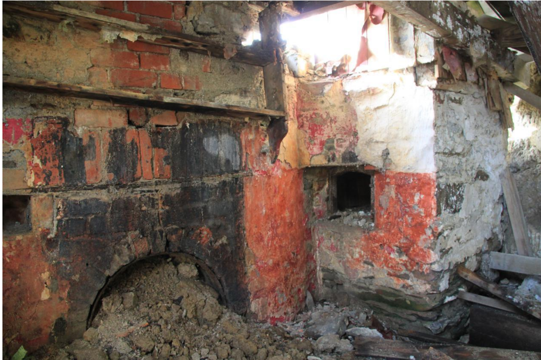
Plate 31 - AD004-BR-031 - Brick fireplace and bread oven. N.B. the later brick infill to fireplace.
