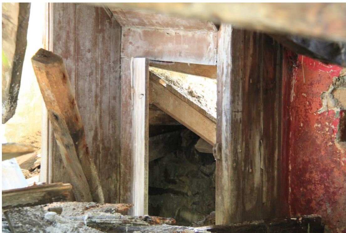
Plate 33 - AD004-BR-033 - Underside of stair, clad with bead-and-butt boards.
