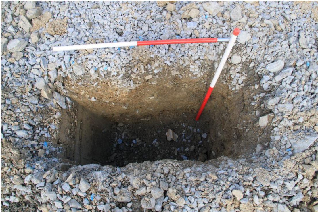
Plate 78 - AD004-D3-078 - Foundation pit, for steel post.
