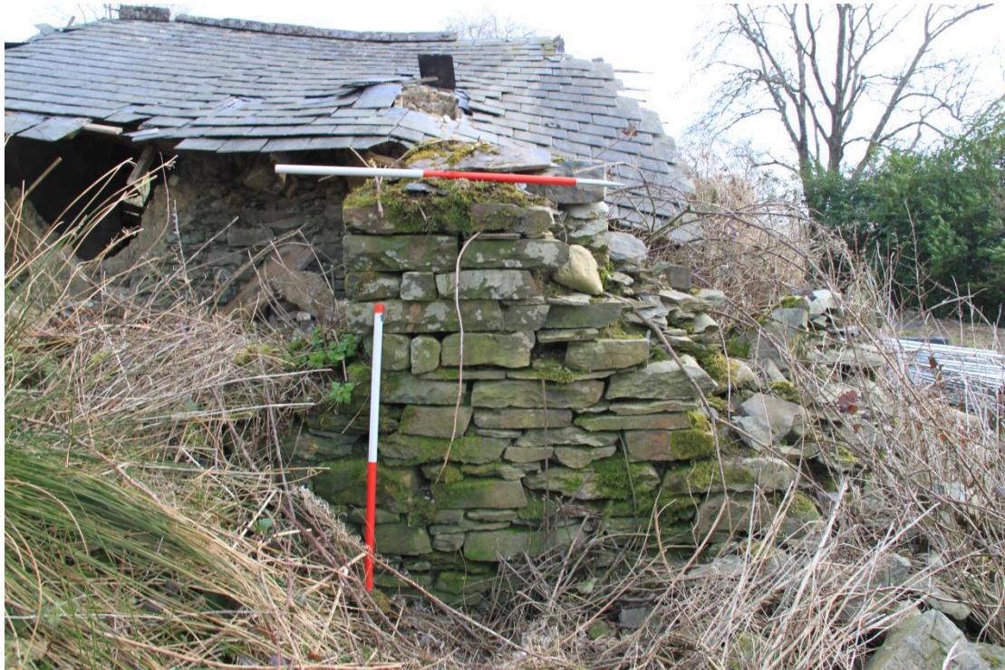
Plate 17 - AD004-BR-017 - West elevation of stone extension, showing window reveal.
