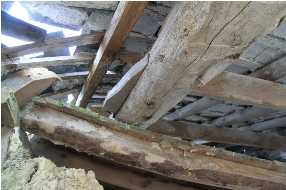
Plate 38 - AD004-BR-038 - Purlin cleat remaining on principle rafter.
