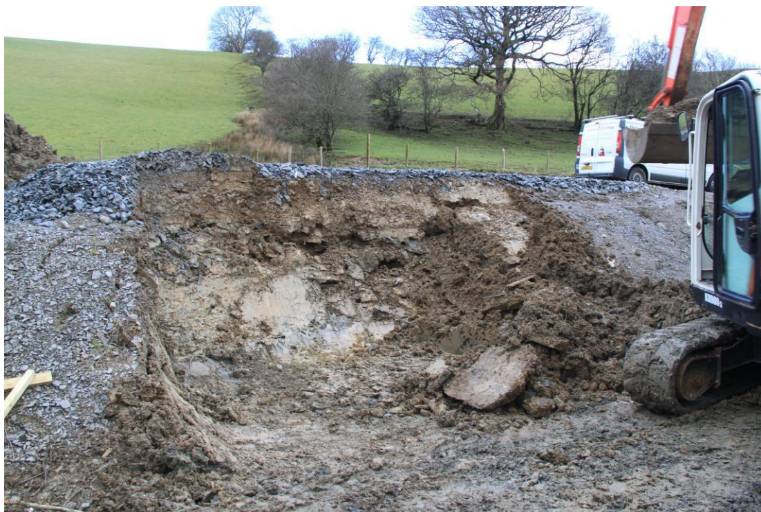
Plate 59 - AD004-D2-059 - Excavation of for retaining wall foundation slab.
