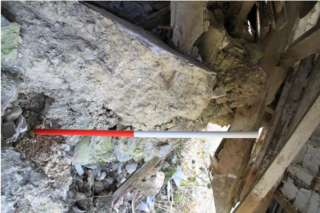
Plate 12 - AD004-BR-012 - Clom wall in section, west lateral wall. N.B. the 'break' where the later layer of clom was added.
