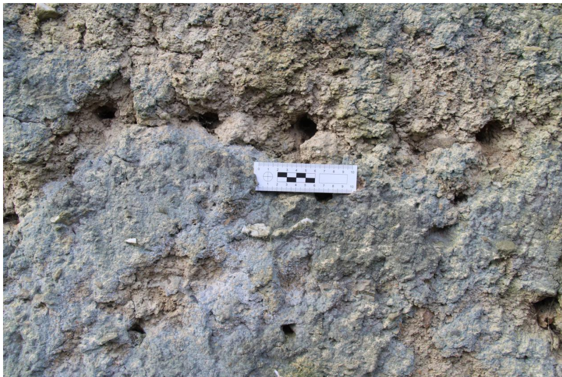
Plate 23 - AD004-BR-023 - Detail of 'pug holes' to support the adherence of render, east elevation.
