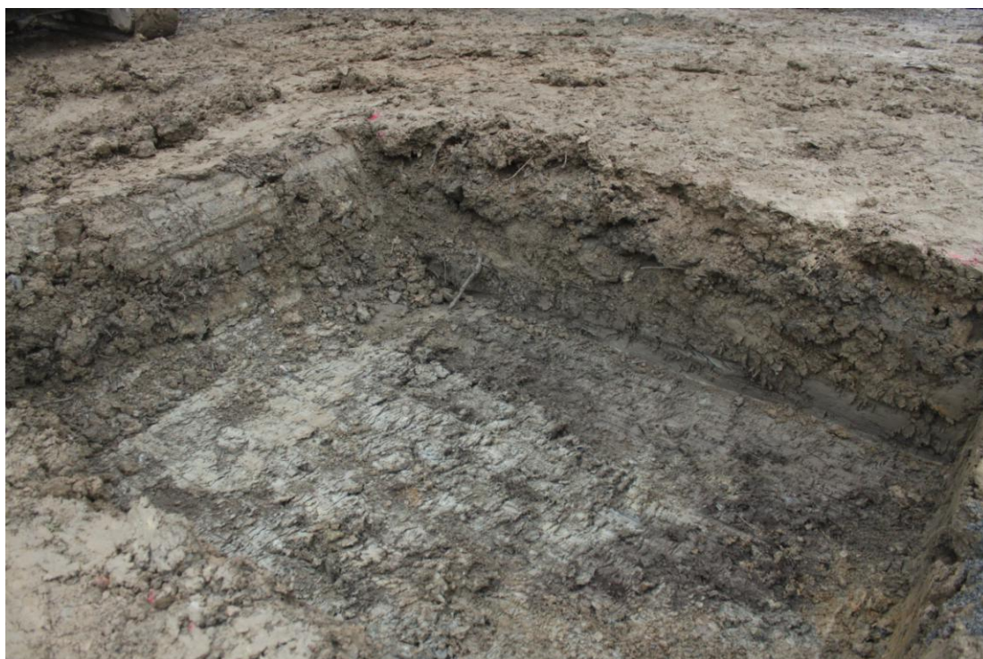
Plate 93 - AD005-D5-093 - Excavation of septic tank pit.
