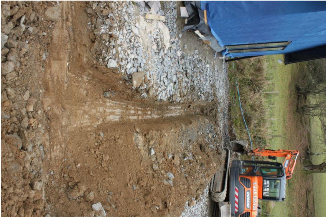
Plate 84 - AD005-D4-084 - Excavation of waste service trench, east end of site.
