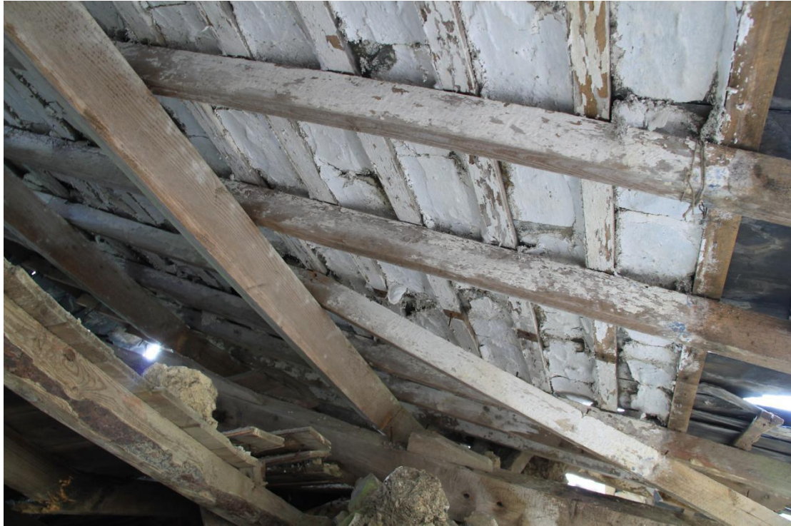
Plate 37 - AD004-BR-037 - Limed underside to slated roof.
