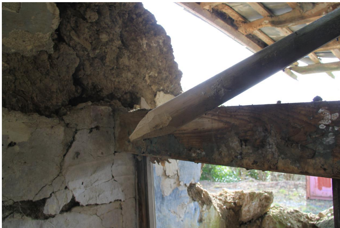
Plate 40 - AD004-BR-040 - Spiked end to later common rafter.
