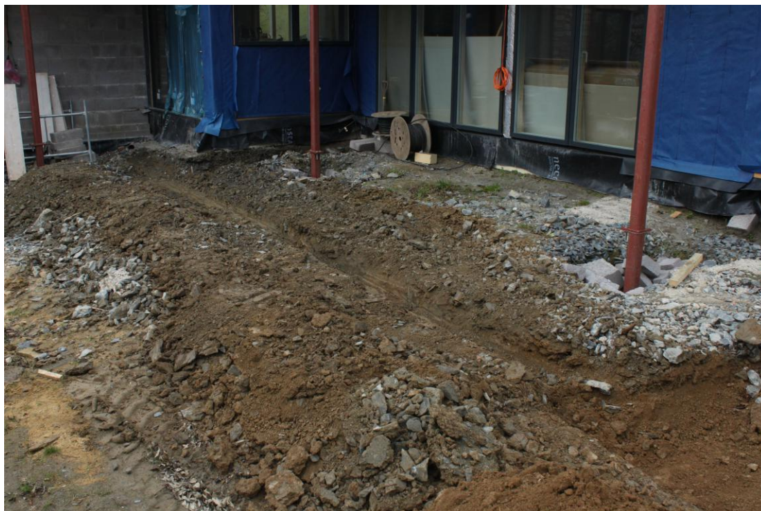
Plate 83 - AD005-D4-083 - Excavation of waste service trench, across south of site.
