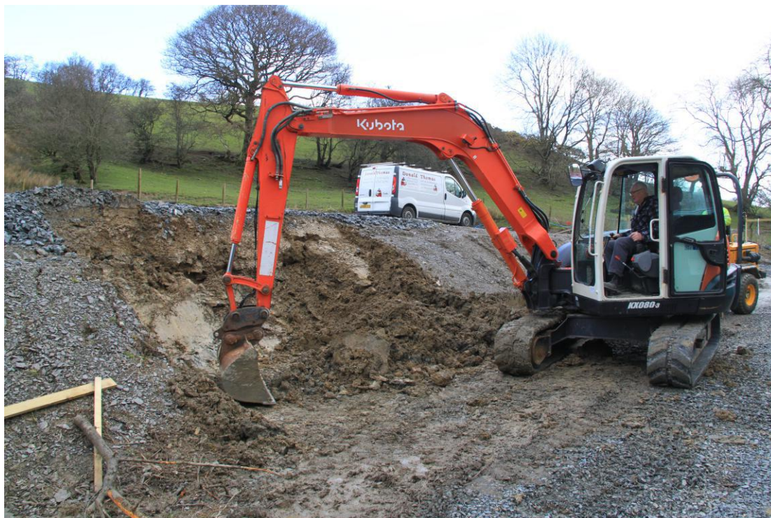
Plate 58 - AD004-D2-058 - Excavation of for retaining wall foundation slab.
