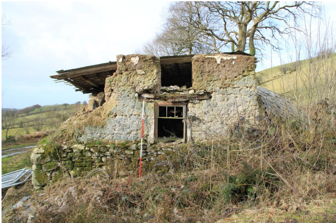
Plate 2 - AD004-BR-002 - View of east elevation. N.B. the change in clom colour to top of wall.
