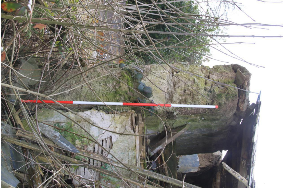
Plate 13 - AD004-BR-013 - Section of east lateral clom wall. N.B. the change in colour and texture to top circa 70cm of the wall.
