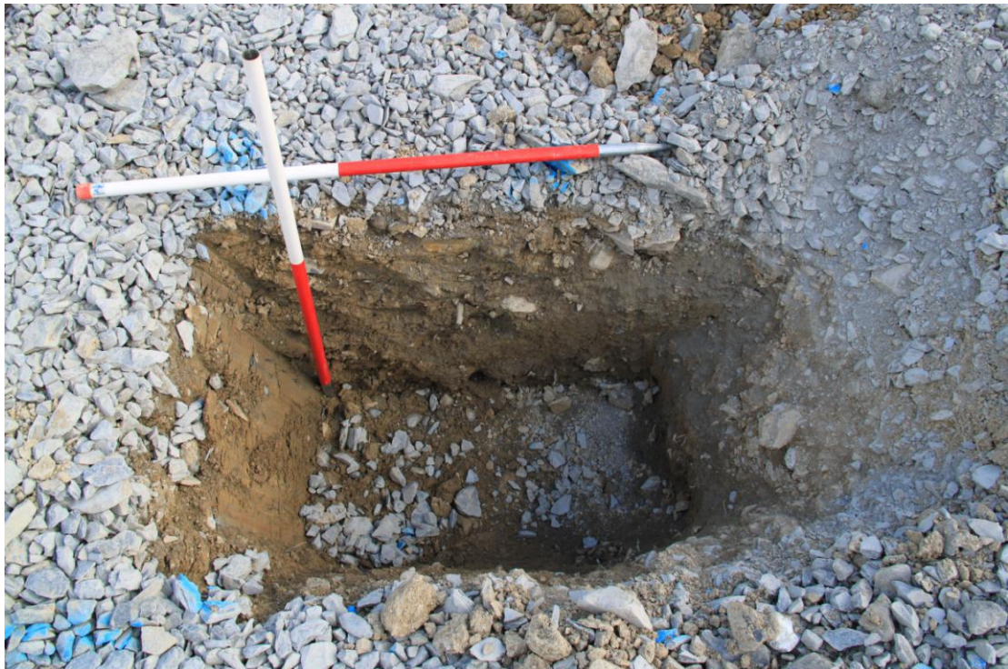
Plate 77 - AD004-D3-077 - Foundation pit, for steel post.
