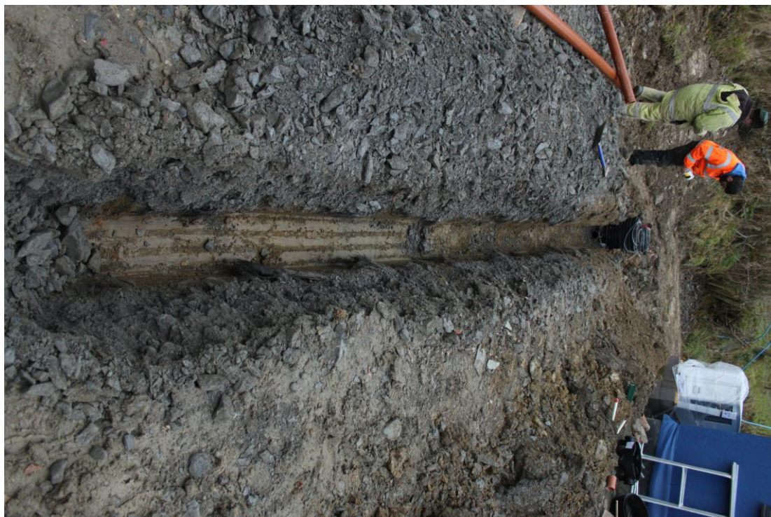
Plate 88 - AD005-D5-088 - Excavation of waste service trench, west end of site.
