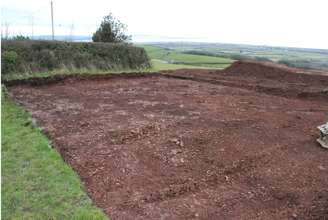
Plate 7 - AD003-D1-007 - Completion of excavations for foundation raft.
