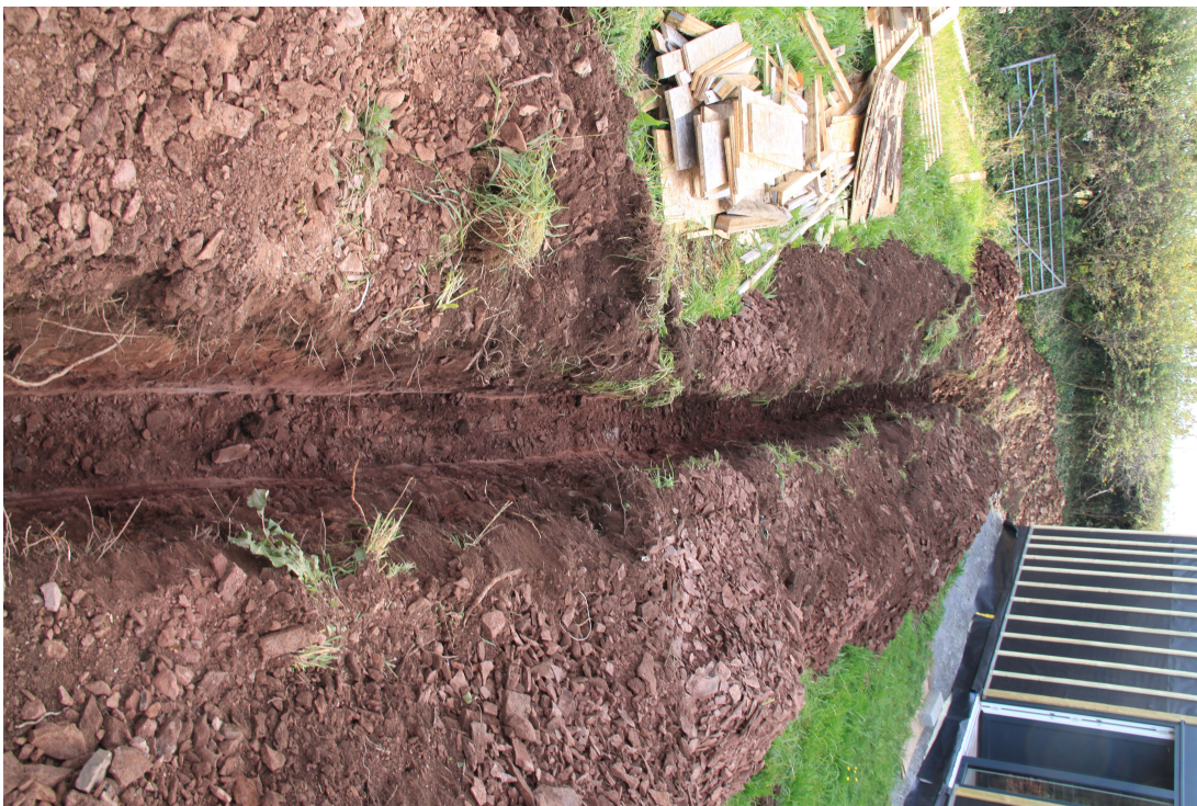
Plate 8 - AD003-D2-008 - Service trench across north of site.
