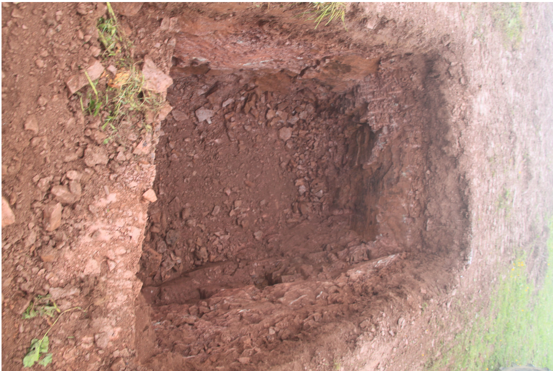
Plate 18 - AD003-D3-018 - Completed septic tank excavation.
