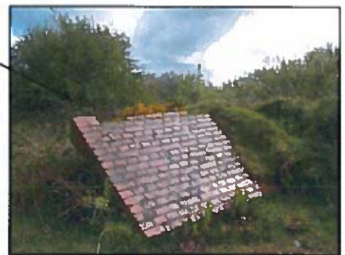
Figure 51 End wall collapsed
