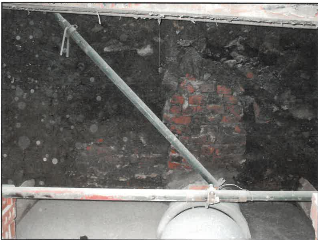
Plate 4: Connexion to the north-south Victorian sewer from the west
