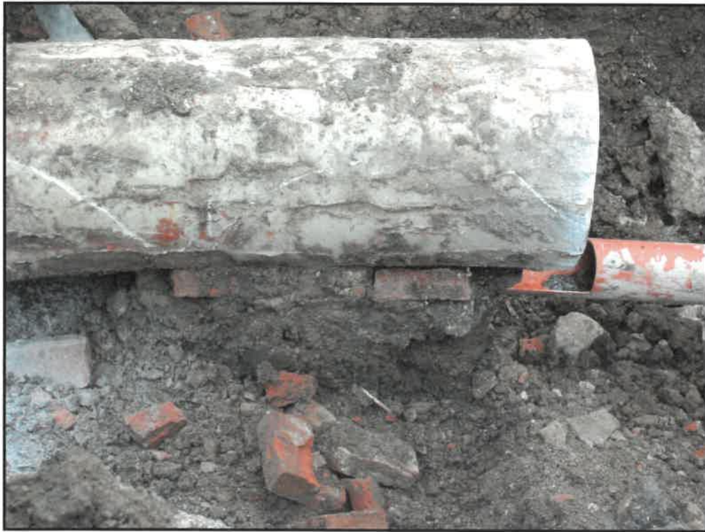
Plate 3: The Victorian sewer and its modern fibreglass lining from the north
