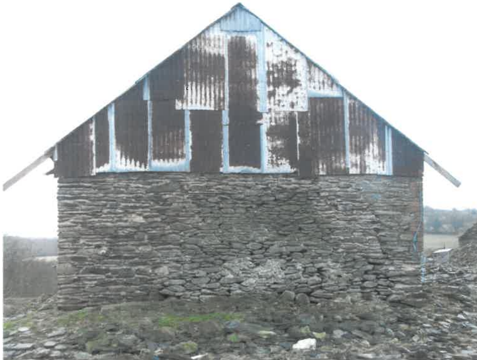
Figure 10 Cowshed (2) North gable of (15) showing repairs
