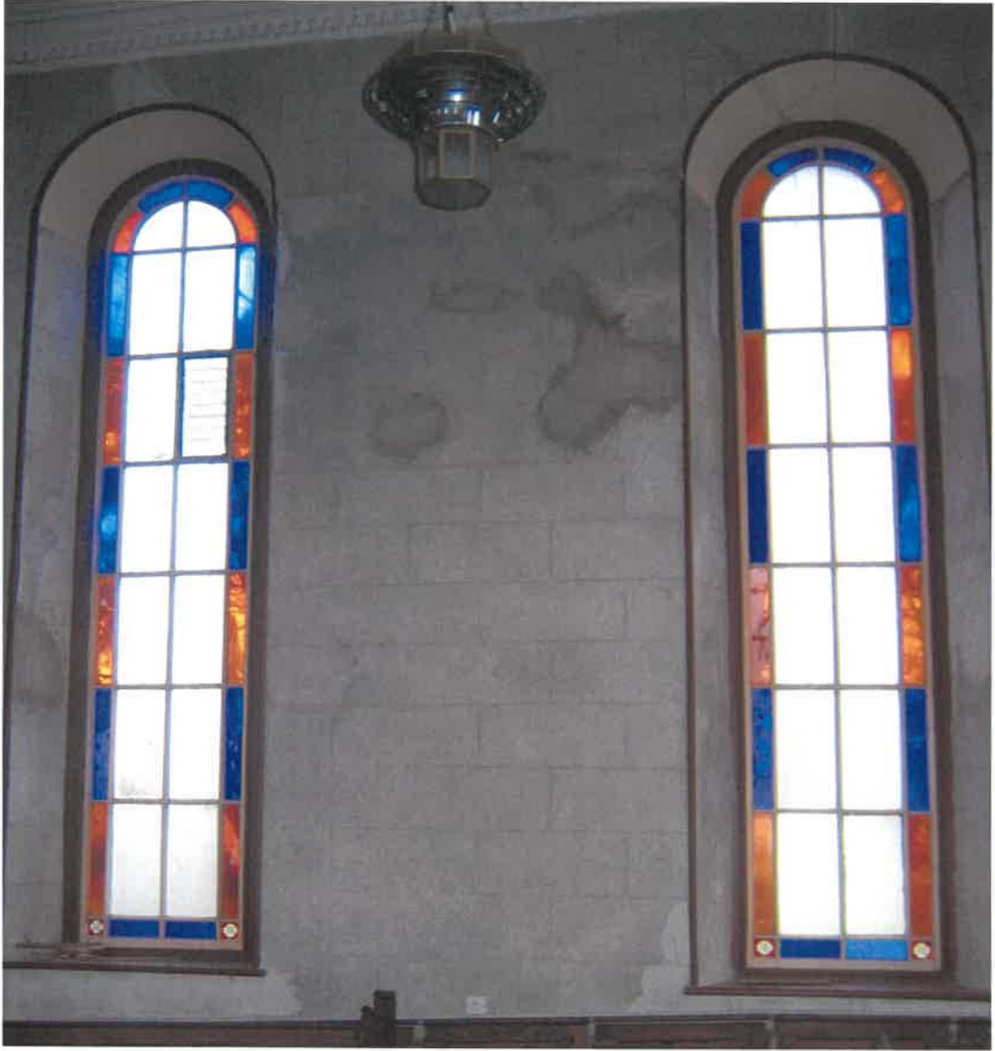
Window detail in main Chapel
