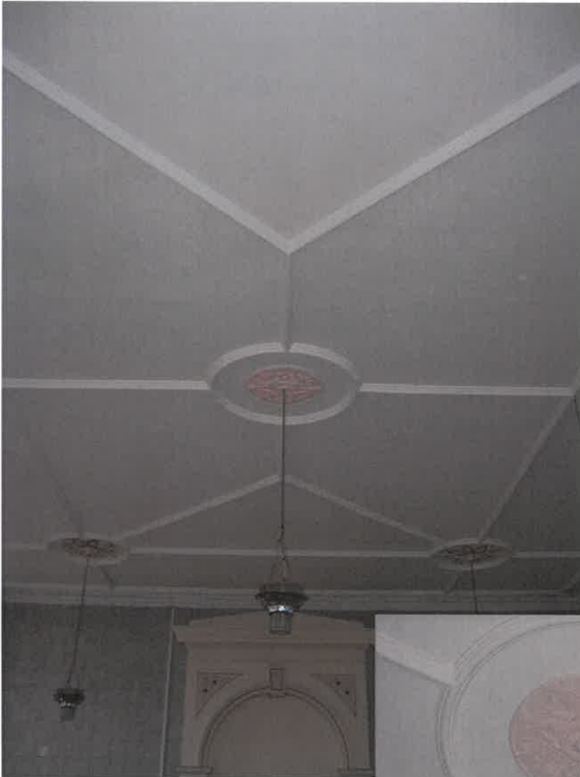
Detail of ceiling and roses
