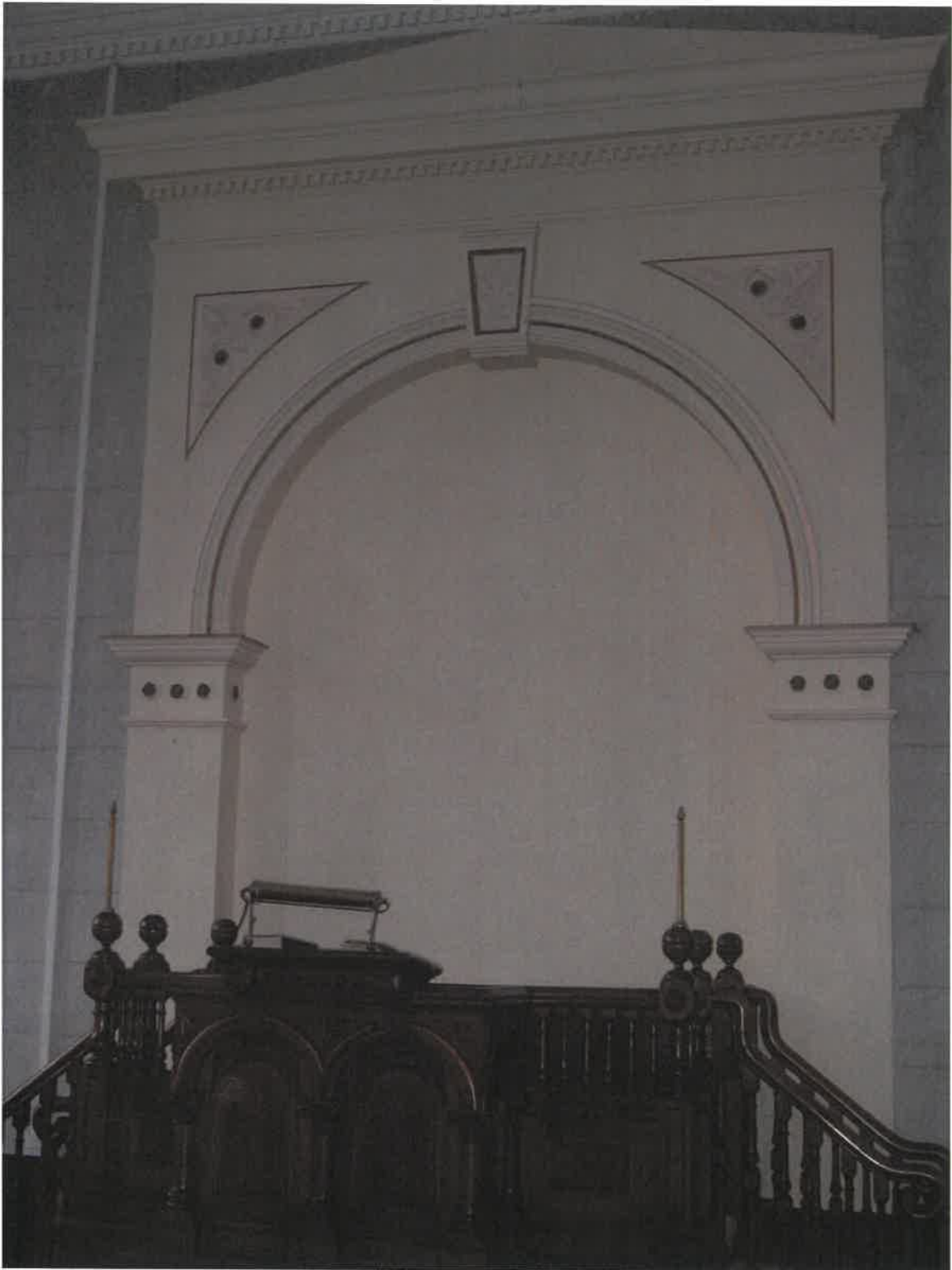
Plaster panel behind pulpit
