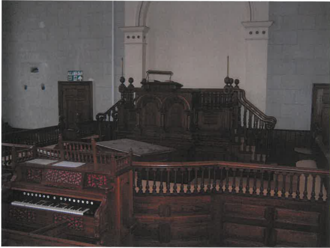
View towards pulpit Outer balustrading and panelling are to be removed
