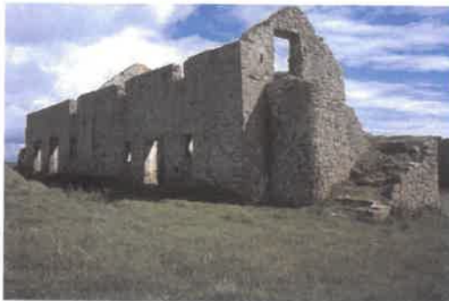
Plate 48. The large barn, its slit window blocked by the external stair
