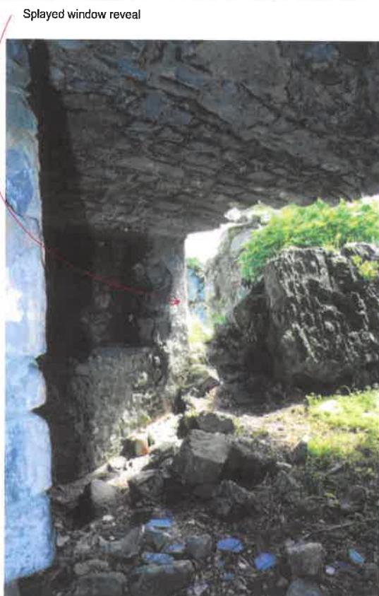
Plate 9. Collapsed vaulting in the south-east service room
