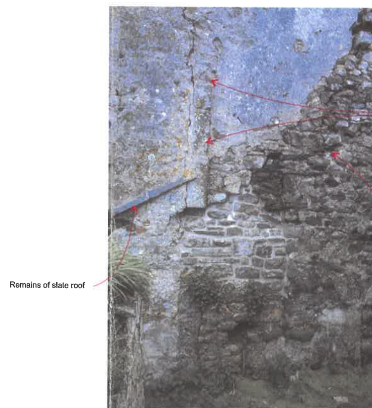
Plate 34. Detail of masonry surrounding inserted chimney
