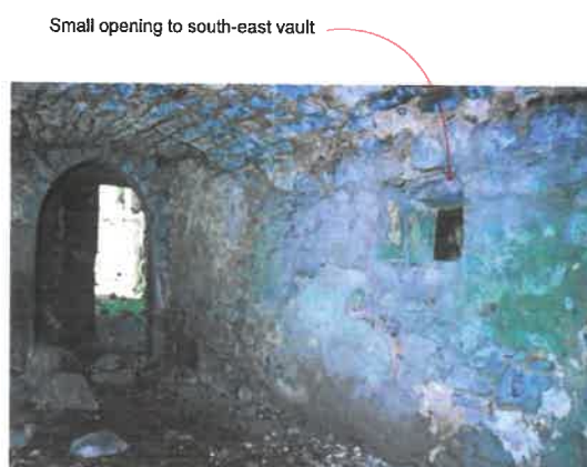
Plate 12. The north-west vault with a window for sharing light between the two service rooms
