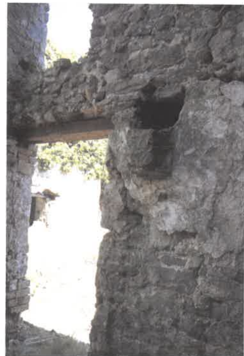
Plate 18. A rough corbel in the south-east wall of the hall
