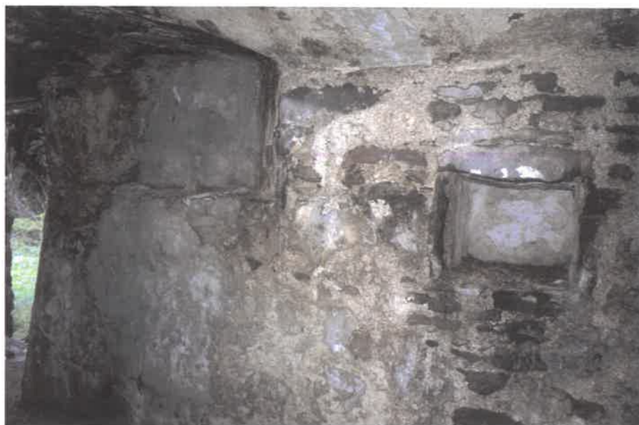
Plate 13. The blocked openings in the north-west service room
