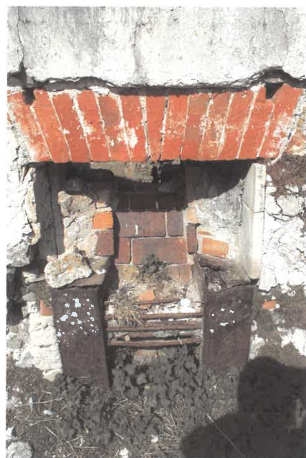
Plate 28. Cast iron fireplace in north-east wall of the Solar
