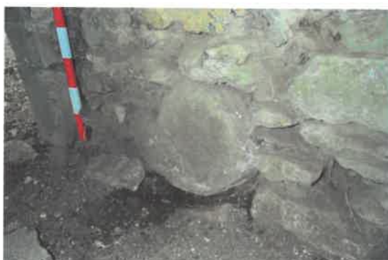
Plate 11. Padstone or column base used as infill
