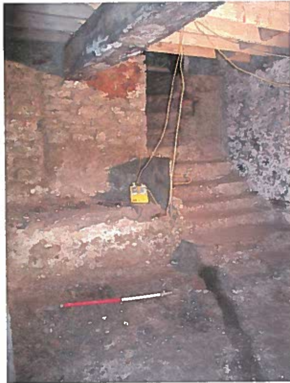
Plate 32; Area of basement at side of entrance steps. Showing blocked single culvert running west from beneath stone steps (looking east)
