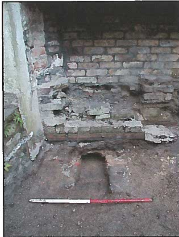
Plate 19: Remains of exposed air duct for brick oven in earlier hearth (looking south-west).
