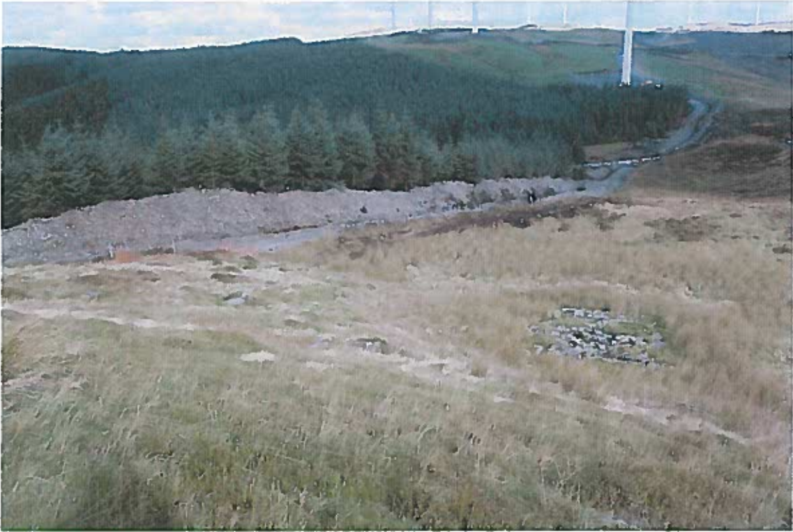
Plate 3 Groundworks on cable route between Turbines 11 and 12, passing PRN 33266. Photo CPAT CS04-56-20
