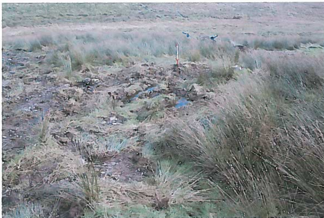
Plate 5 Surface damage to trial working PRN 33236 at grid connection pole 118. Photo CPAT CS04-56-23
