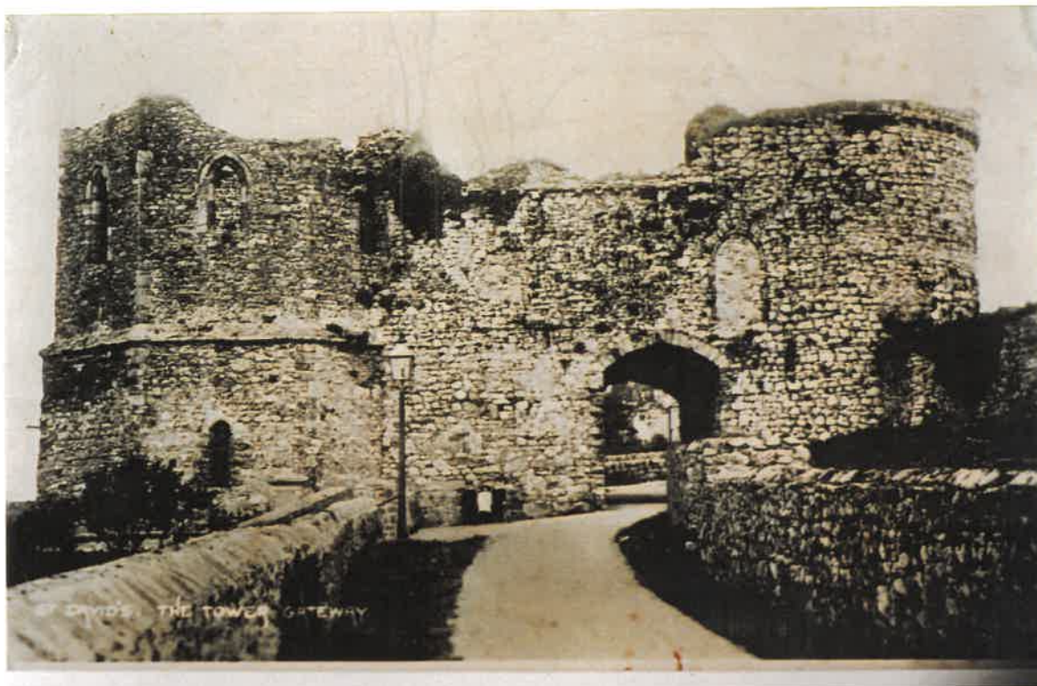
The western elevation of the gate around the turn of the century, showing the first floor openings blocked with masonry, but with considerably more masonry at the top of the north-north-western elevation of the belfry. By c.1925 the western window and first floor doorway had been reopened, but the belfry parapet had been reduced. [postcard from the collection of J.Viles and Sons]
