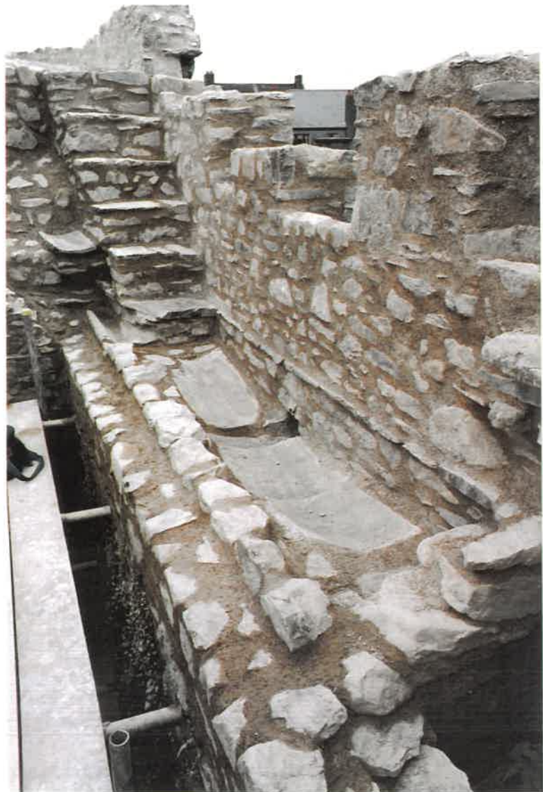
PT98/15/19: The south end of the parapet of the west elevation showing the gutter to carry off water from the chimney and parapet steps emptying through the exterior wall; the two gutter-slabs to the east of the steps which rose to the tower parapets; and the ledge and socket to accommodate the wall plate of the gatehouse chamber roof. [After repair]
