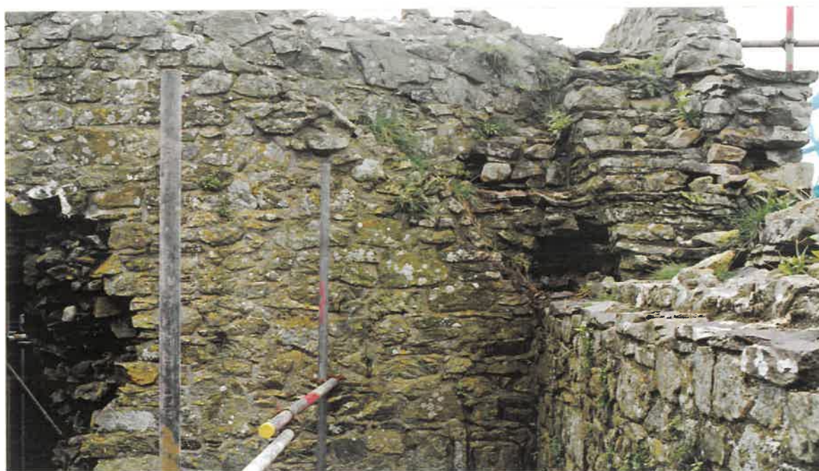
PT98/7/32A: The north-west corner of the gatehouse chamber showing the remains of the original roof-line, with the socket for the wall-plate beneath
