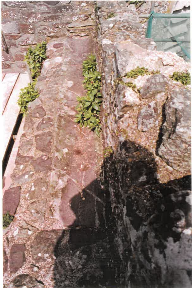
PT98/12/8: The remains of the gutter on the northern end of the east parapet, rebbed when the parapet was repaired under Alban Caroe in 1950-1. At this time the wall top was rebuilt removing any traces which may have survived of the slot along the inner margin of the wall to accommodate the wall plate of the medieval roof.
