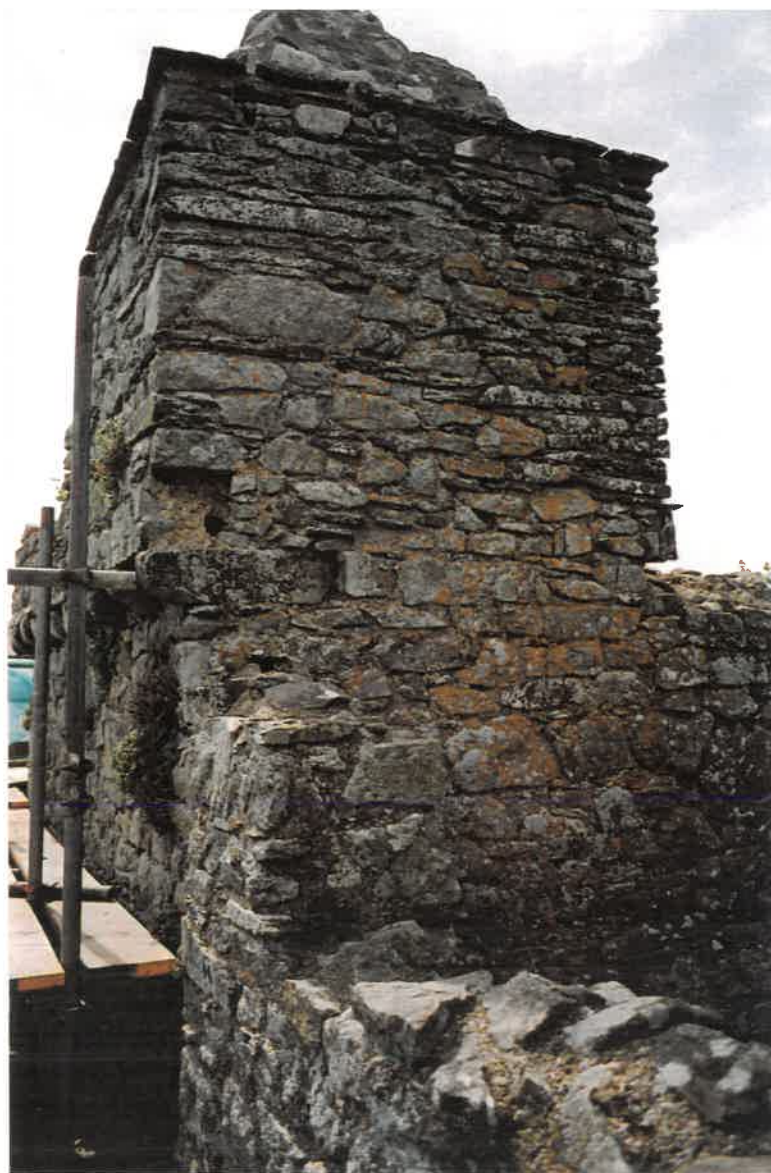
PT98/11/27: The northern elevation of the stair turret at the north-east angle of the south tower, showing the scar of the junction of the parapet occupying the course above the tower string-course. This provides evidence for the original height of the merlons over the gatehouse chamber. The cap of the stair turret was renewed by Caroe in c.1950-1.
