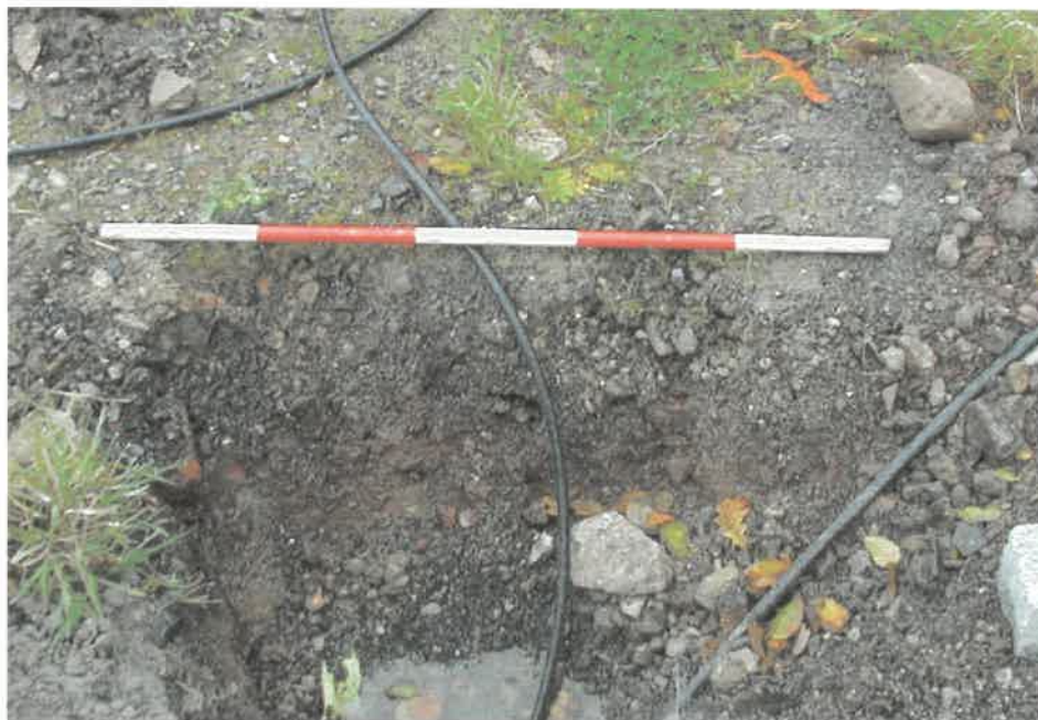
Plate 03: Detail of service trench containing crushed red sandstone pathway in section. (Scale 1m.)
