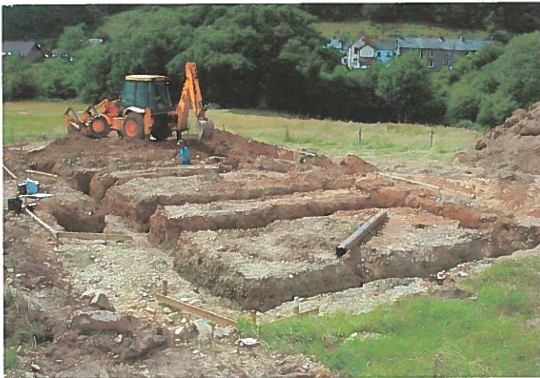
Plate 02: Shot of Plot 8 following excavation of footings, looking west.
