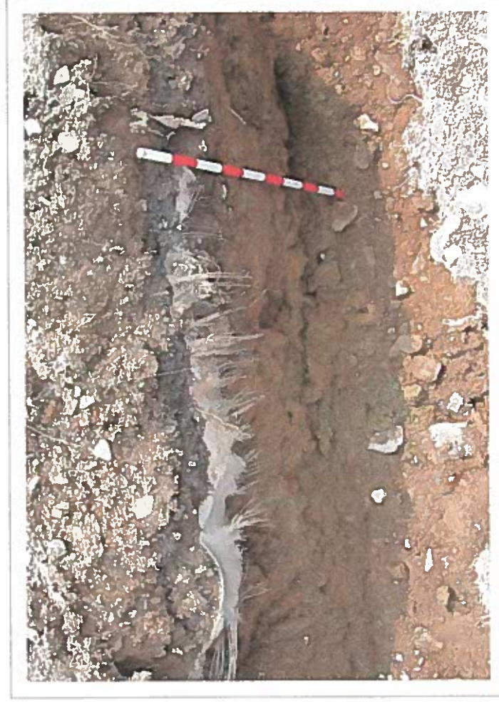
Plate 03: Shot of section showing gravel chippings and geotextile base, looking south-east.
