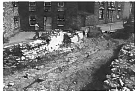
16. Foundation trench for new boundary wall
