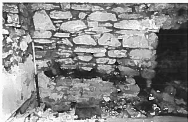
9. Repaired lower section of east wall in parlour, at floor level
