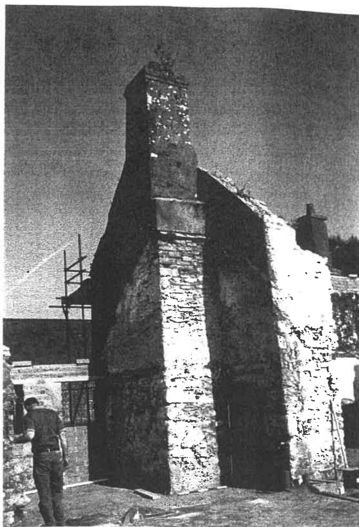
Plate 2 The large external chimney on the south wall - camera facing NW. Note:- a) external pink limewash to ground floor height b) top of 'Flemish' chimney to right.
