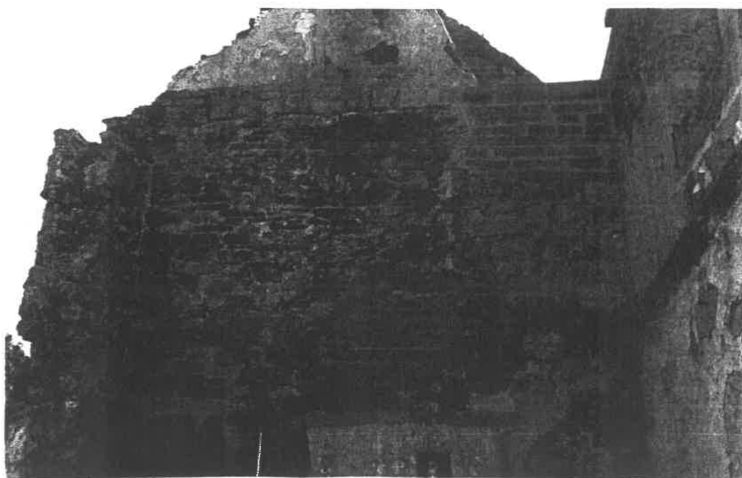
Plate 3 The upper part of interior of south wall (U) - camera facing south. Note:- a) change in masonry above ranging pole showing 'ghost' of chimney flue in wall b) blocked-in hearth and also old concrete filling old lintel position
