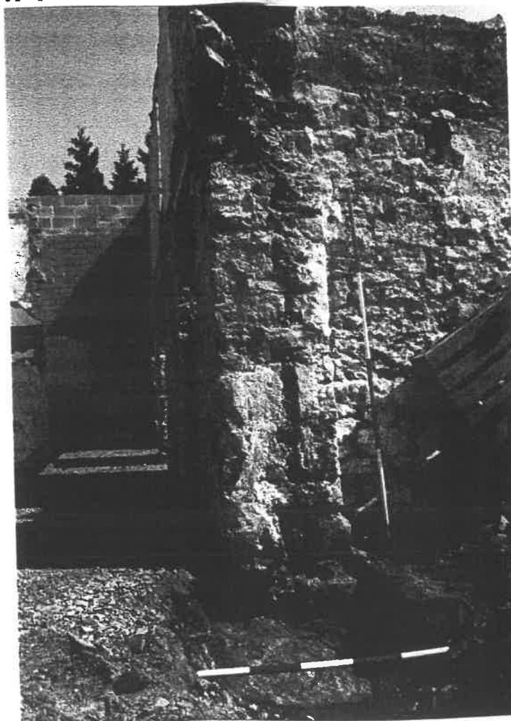
Plate 7 The southern end of wall (R) with wall (X) removed - camera facing north Note:- a) old lime plaster finish indicating that this was the north side of an opening b) yellow/orange bedrock in base of foundation cut (10).
