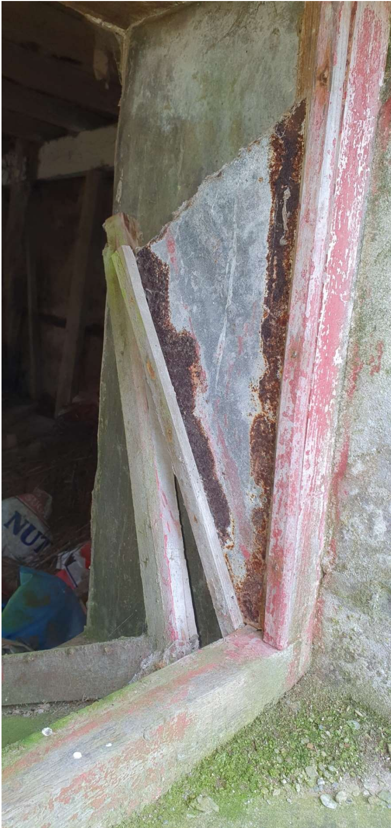
Glanrhyd Photographic Survey Covering Document 18/3/2021 Ref:1871 Llyr Evans Planning Ltd. PCC Ref: 20/0403/PA
