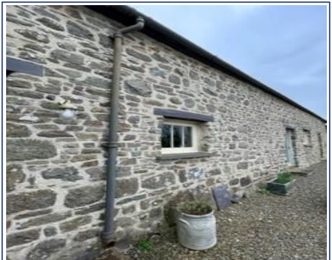
Figure 71: The Byre Rear (North Elevation) showing the painted metal rainwater goods.
