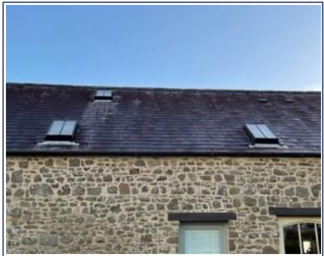
Figure 91: The Byre Rear (North Elevation) showing the conservation roof light windows.
