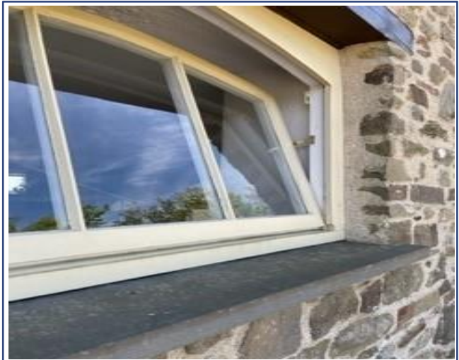
Figure 81: The Byre Rear (North Elevation) Lounge window slate windowsill.
