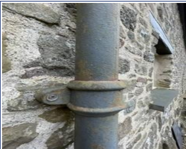
Figure 70: The Byre Rear (North Elevation) showing the painted metal rainwater goods.
