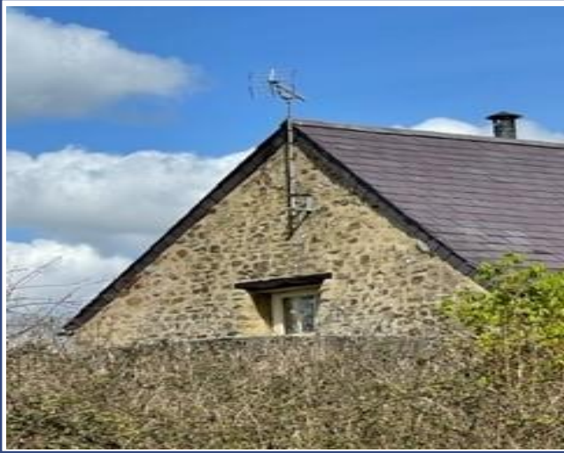
Figure 72: The Byre Side (West Elevation) showing the metal wood burner flue.
