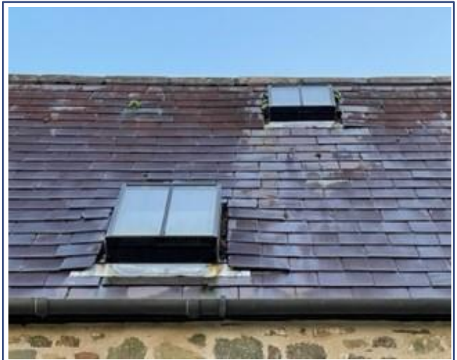
Figure 93: The Byre Rear (North Elevation) showing the conservation roof light window (Bedroom 3).
