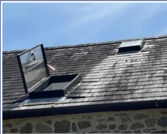
Figure 92: The Byre Rear (North Elevation) showing the conservation roof light window (Bedroom 3).
