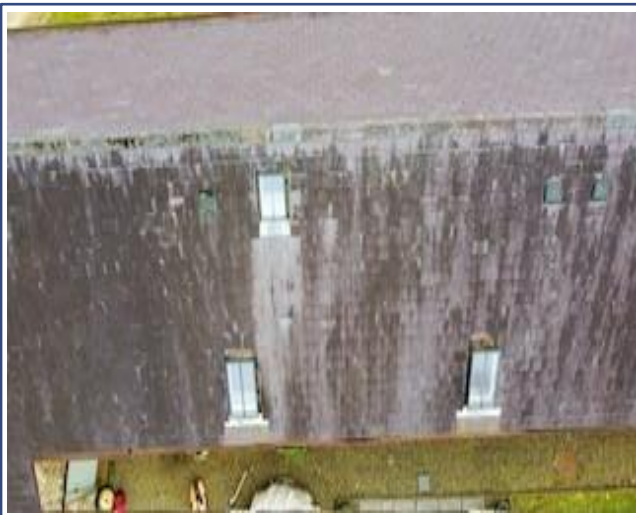
Figure 90: The Byre Rear (North Elevation) aerial view showing the conservation roof light windows.
