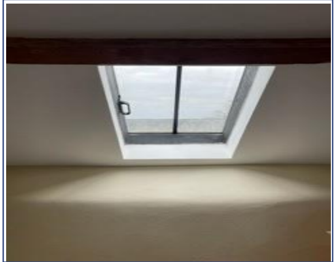
Figure 150: The Byre Bedroom 3 conservation roof light window and oak beam on the north elevation.
