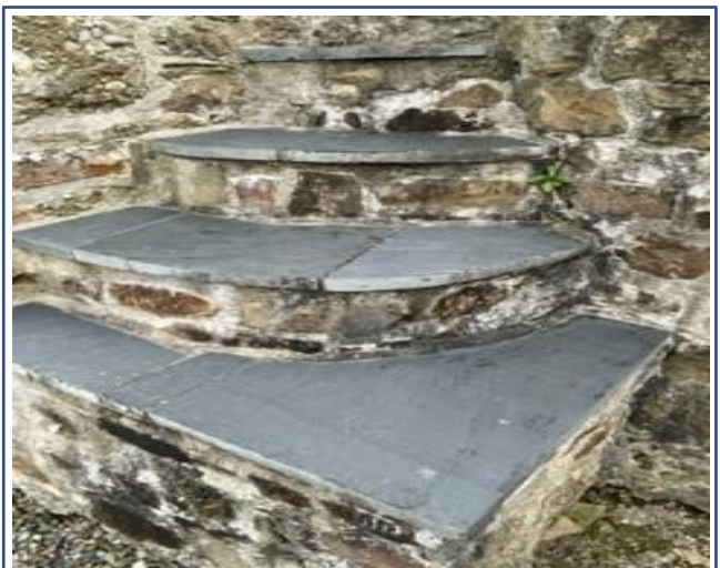
Figure 67: The Byre Front (South Elevation) milking steps showing the Welsh slate.
