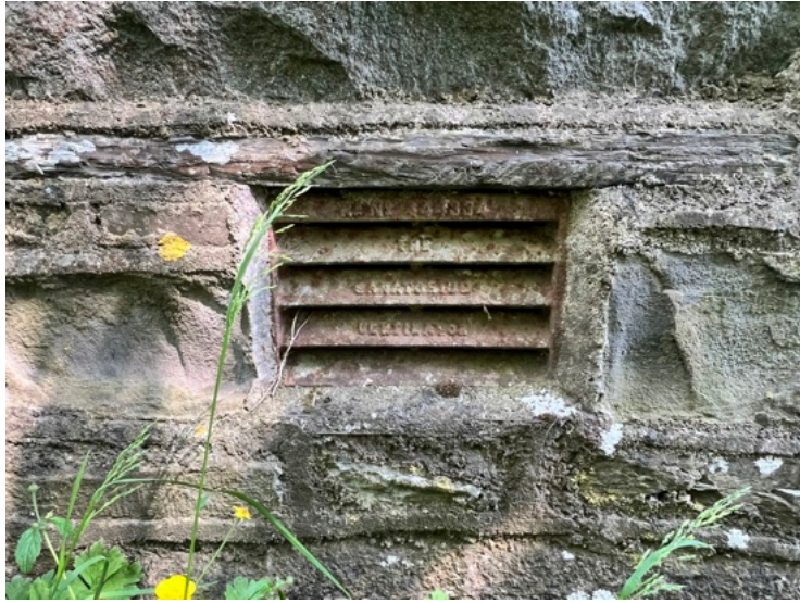
Cast air brick detail South facing elevation
