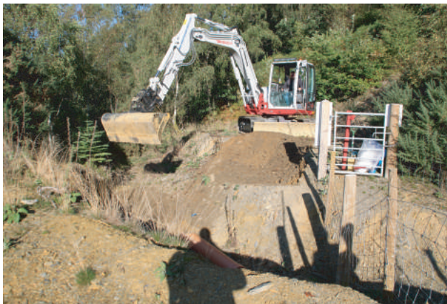
Plate 15. Working shot during creation of temporary access track across drainage channel from Adit No.9. Looking west.
