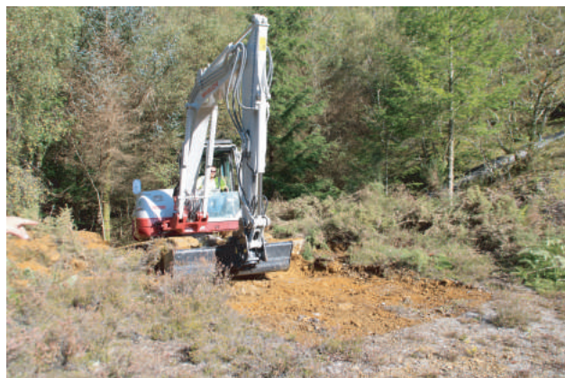
Plate 06. Working shot through area of spoil and scree for proposed temporary access track leading to lagoon area. Looking northwest..
