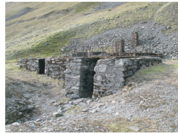
Plate 27. Wall foundations and mounting plates for compressor and turbines (PRN: 98045).
