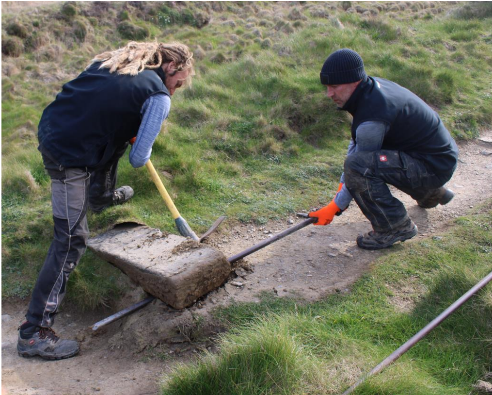
Figure 9. Photo showing approach to remove steps, including pickaxe and then crowbar to help lift steps from the ground.
