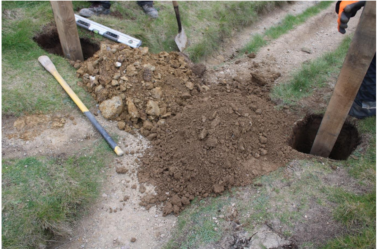
Figure 13. Photo showing pits created to house the wooden posts of physical barrier. Note the colour and composition difference between the material from the two different pits.
