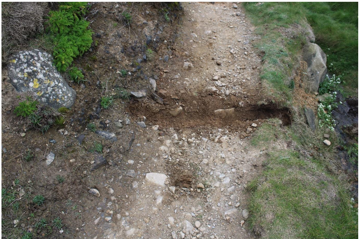
Figure 12. Photo showing shallow drainage ditch created directly above the bottom group of steps that were removed.
