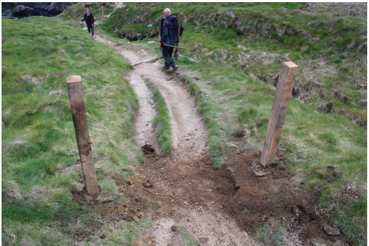
Figure 14. Photo showing posts in place packed with the material dug out to create the pits.
