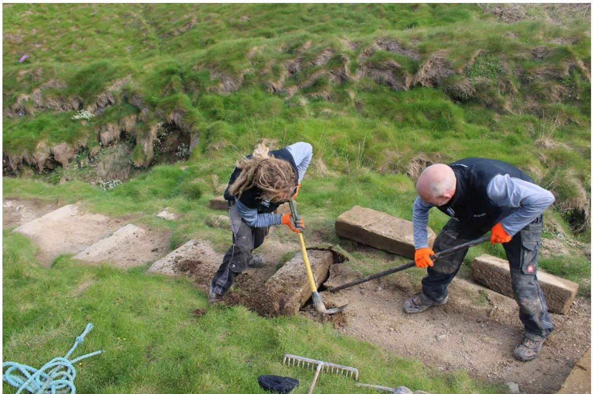
Figure 10. Photo showing removal of steps using hand tools.
