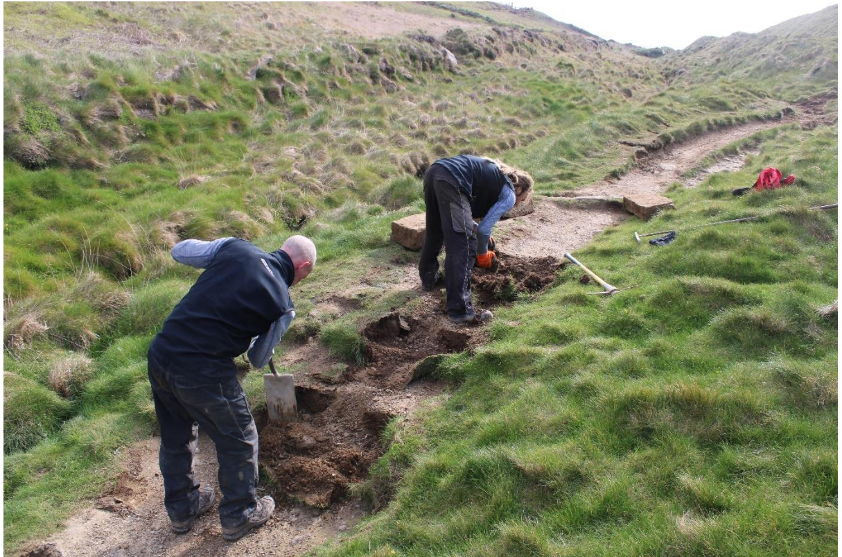
Figure 11. Photo showing use of hand tools to re-profile the surface after removing the steps.
