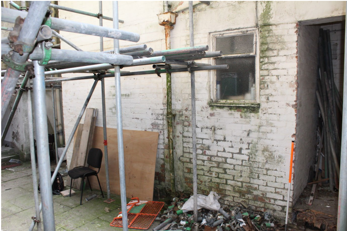
Image EDP 6.7: The ground floor of the Estates Offices features a bricked-up window and a single casement with hopper window above, and metal glazing bars. To the right of the image is the dogleg access route from the courtyard towards the Estates Offices main entrance and King Street.
