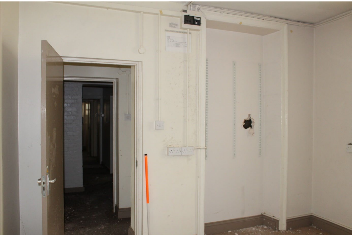
Image EDP 6.18: The western wall of room G4 in the cottage, which features a blocked-up doorway (right) and a modern doorway from which the Estates Offices is accessible via a dogleg.
