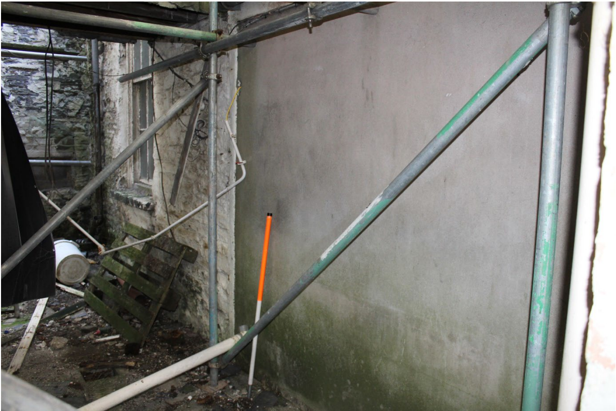
Image EDP 6.6: Just seen is the rear elevation of the Cottage, formed of a mixture of stone rubble. The rear ground floor contains an original six-over-six sash, which was not updated when the front windows were converted to plate glass in the late 19 th century.
