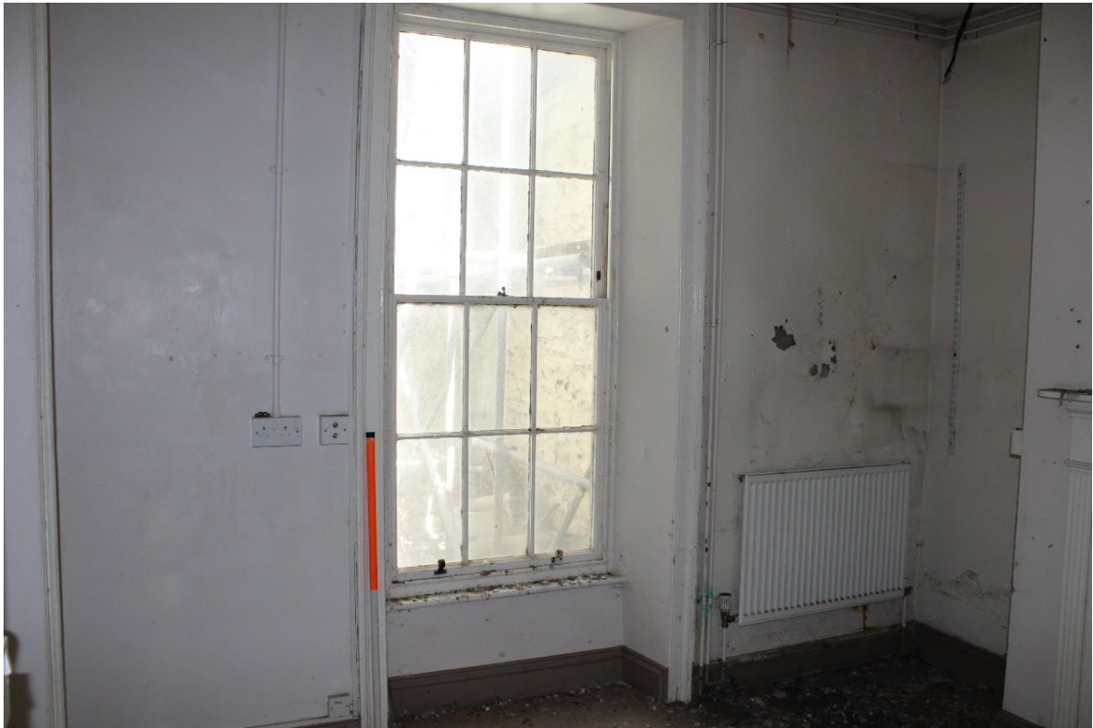
Image EDP 6.19: The original (pre-1860) sash window with thin glazing bars and no horns.
