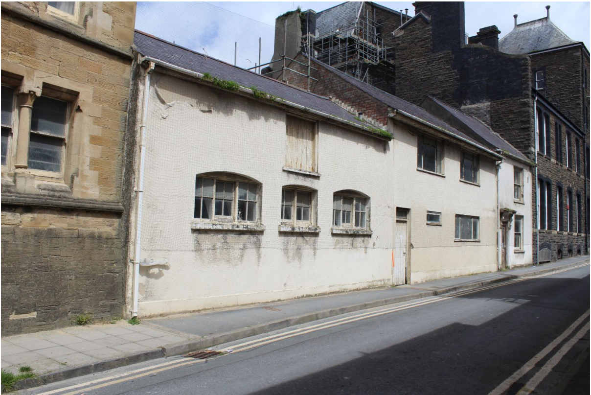
Image EDP 6.4: The King Street elevation is finished with painted render, which tries to present the three buildings as a block, however each building unit has different roof heights, with the Old College Extension having the lowest, Estates Offices the middle, and the Cottage, the highest.
