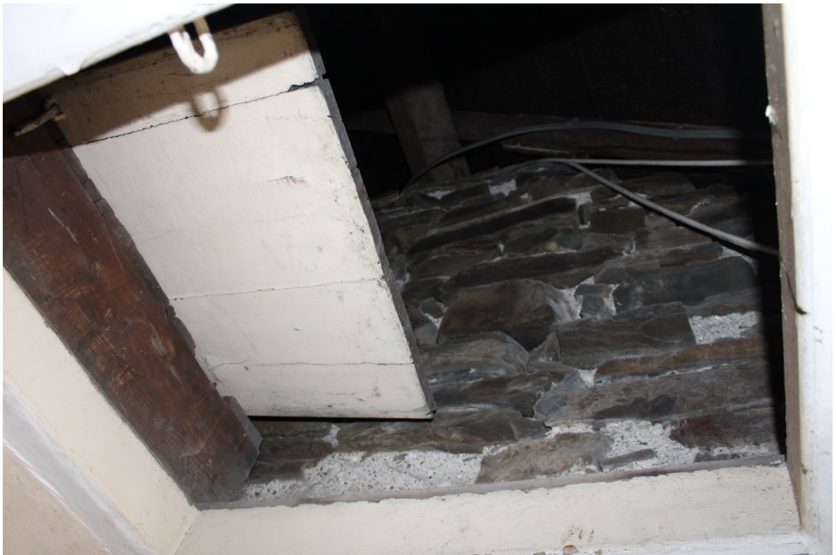
Image EDP 6.22: The ceiling of F4 contains an attic space which shows the dressed stone internal gable end of the cottage.
