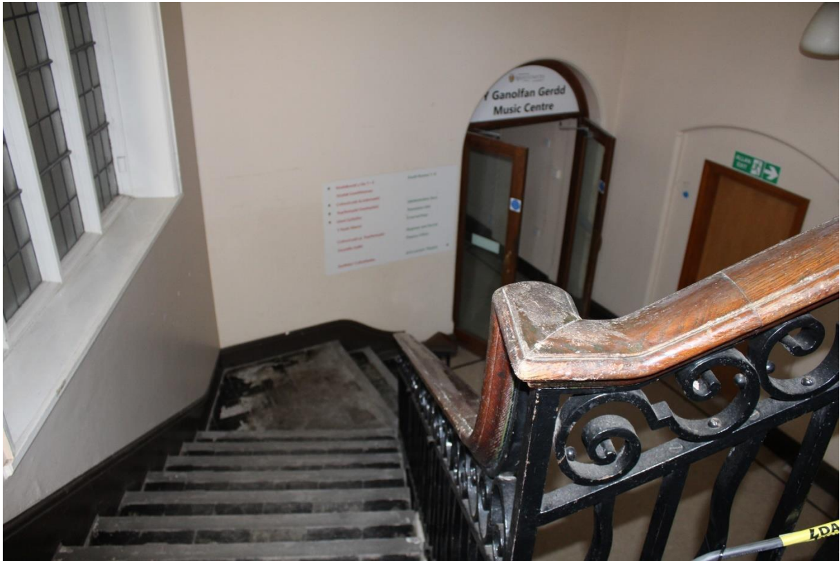
Image EDP 12: The stairwell in the Ferguson Range with its three-sided cantilever staircase
