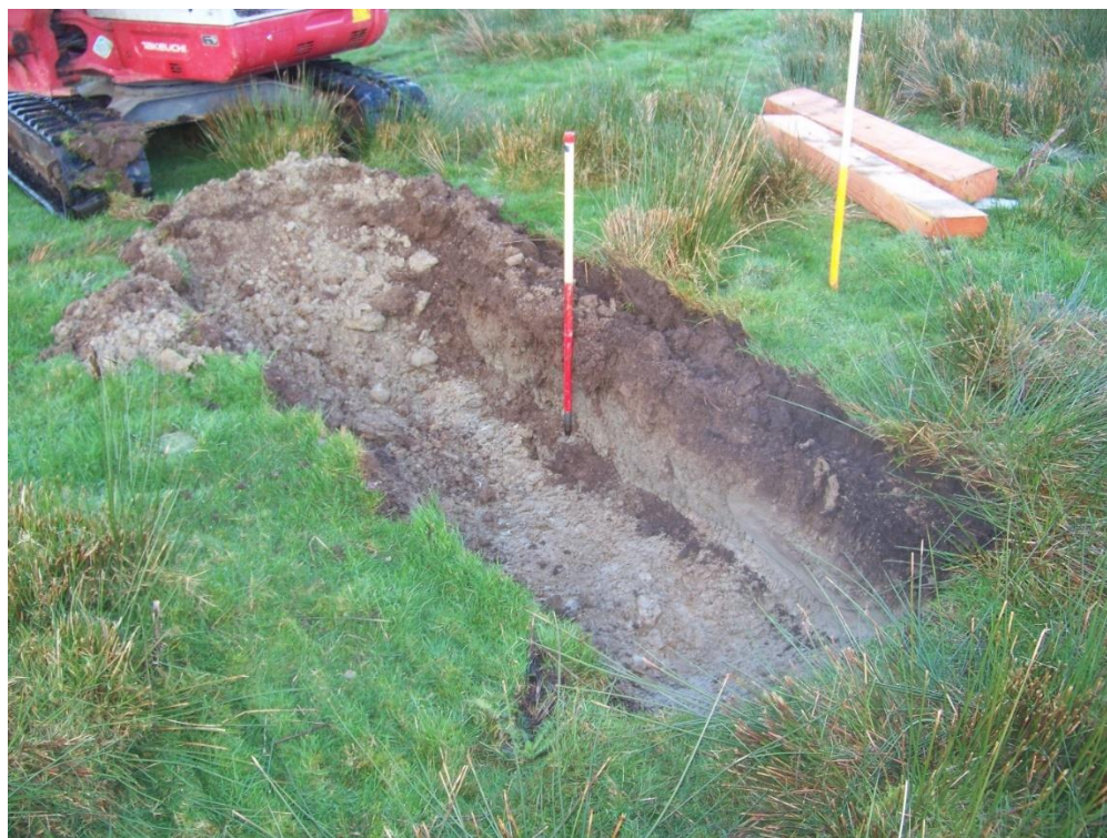
Figure 14 South outer anchor pit. The peaty topsoil around 0.10m deep is clearly visible as is the shale beneath that
