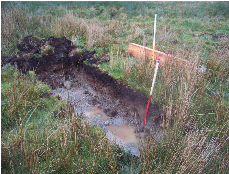
Figure 7 North outer anchor pit. The peaty topsoil around 0.10m deep is clearly visible as is the yellowy grey clay beneath that and the shale 0.30m below the surface.
