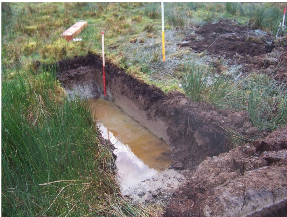
Figure 15 West Outer anchor pit. The peaty topsoil around 0.10m deep is clearly visible as is the yellowy grey soil clay beneath that
