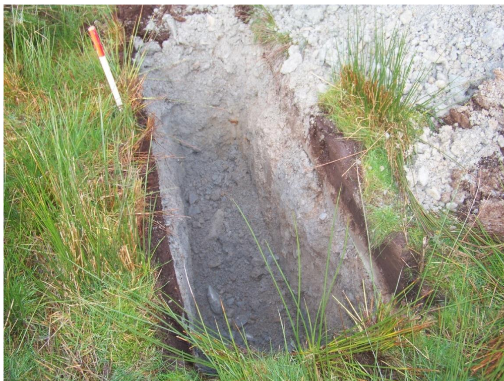
Figure 12 South Inner anchor pit at full depth. The peaty topsoil around 0.10m deep is clearly visible with a band of clay beneath just above the shale
