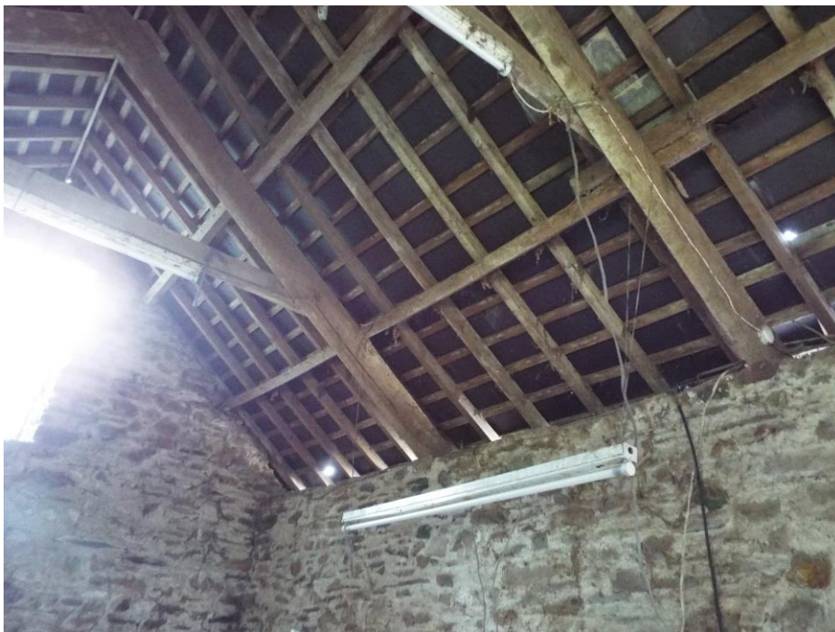
General view of roof showing rafters, purlins and A frames
