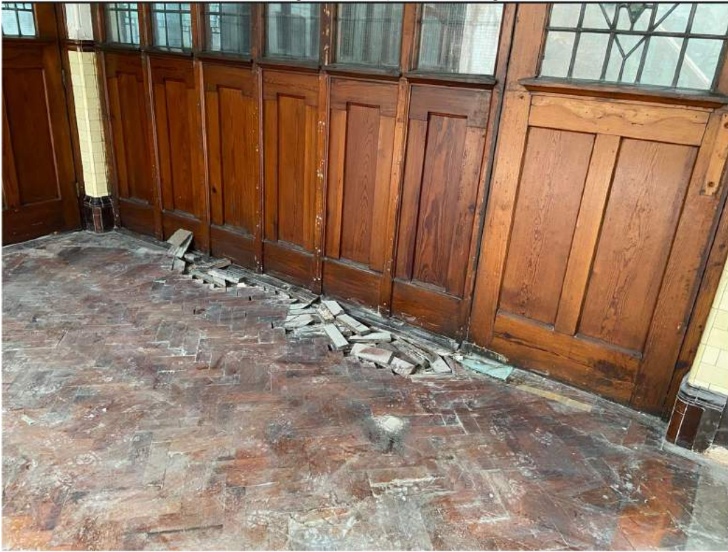
Photo 19 Ground Floor Damage to Parquet Flooring
