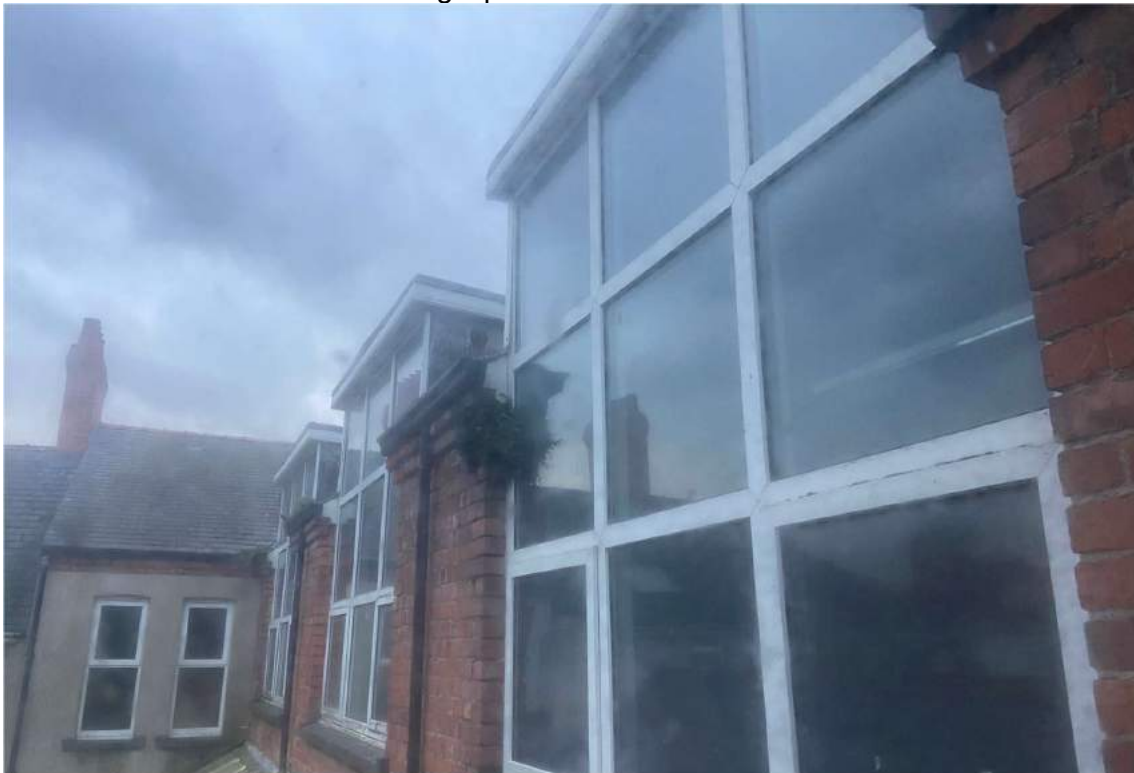
Photo 7 North Elevation Existing Upvc Windows
