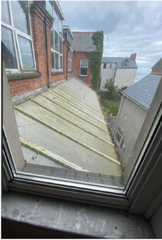
Photo 8 North Elevation Showing Polycarbonate Roofing.
