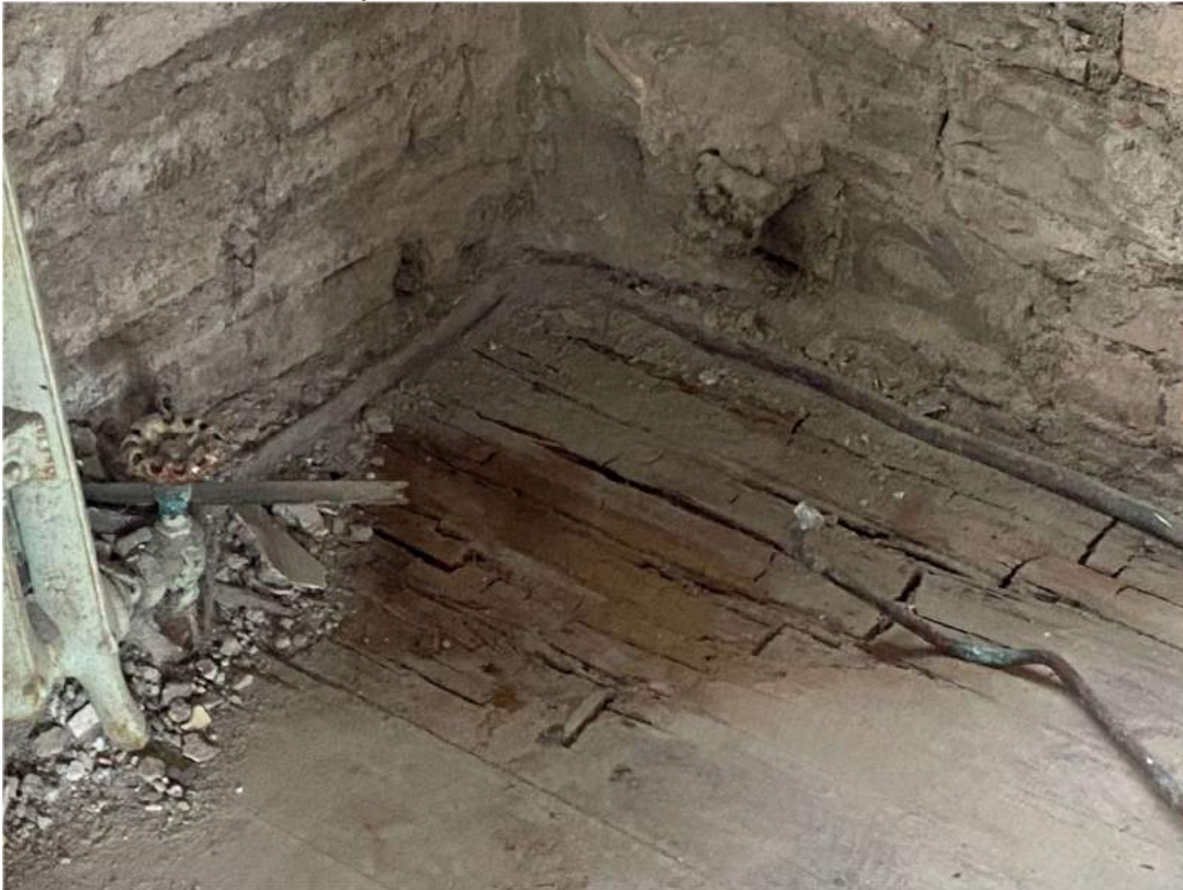
Photo 31 First Floor Dry Rot in Floor Boards
