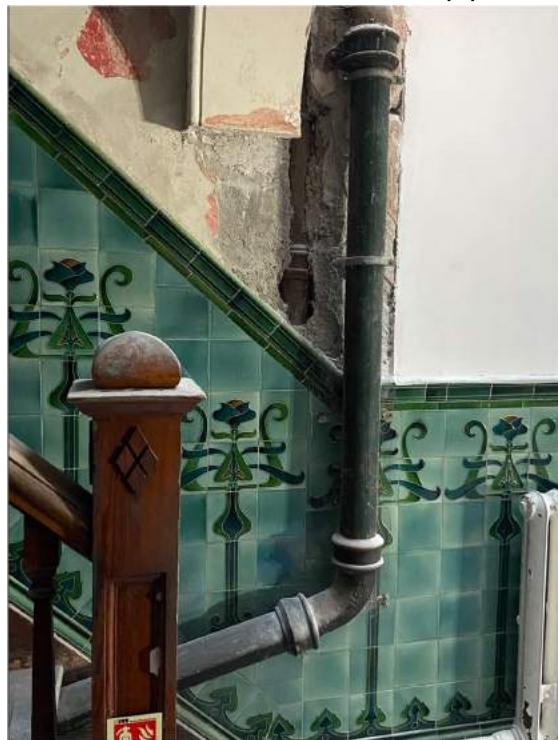
Photo 16 Rear Stair rain water pipe.
