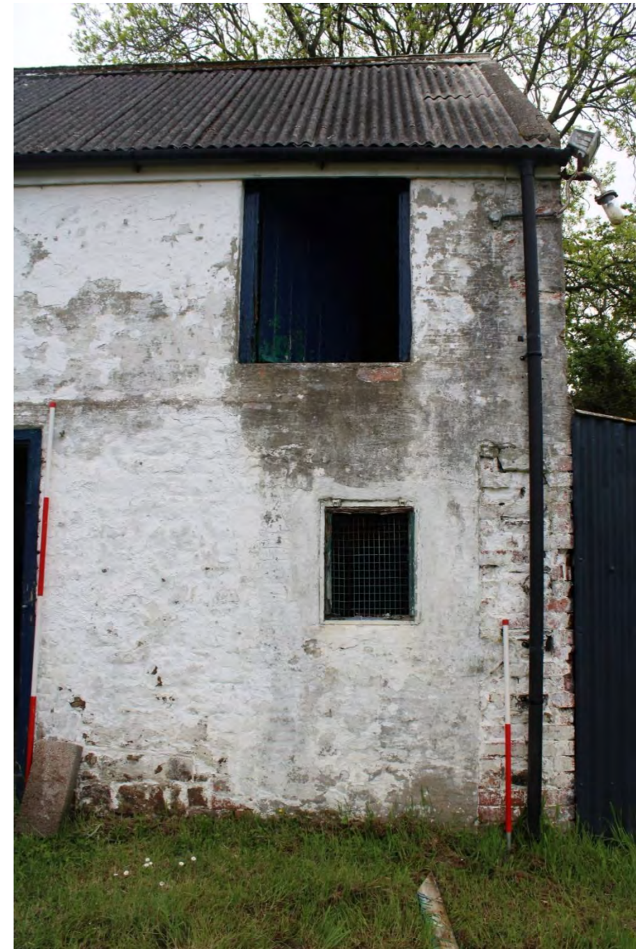
Photo 40: Detail of southern end of western façade of Building D showing the doorway to the first floor, brick repairs on southwestern corner, brick blocked doorway with later window at ground floor
