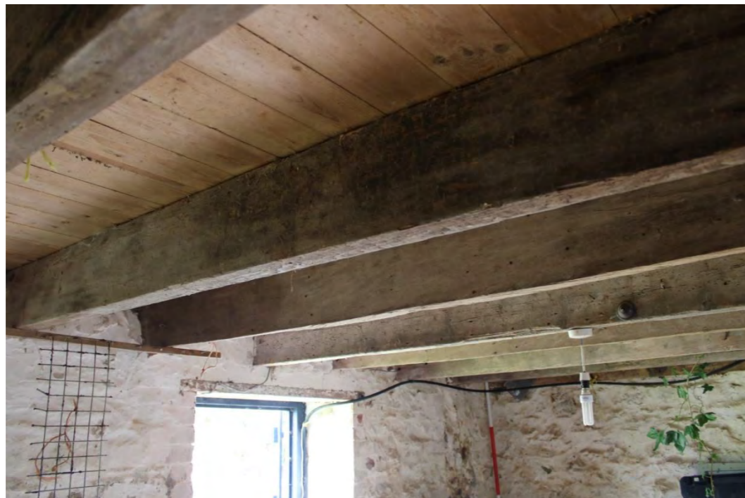
Photo 55: View northwest showing later added ceiling of ground floor level, with rafters and boarding for the first floor of Building D
