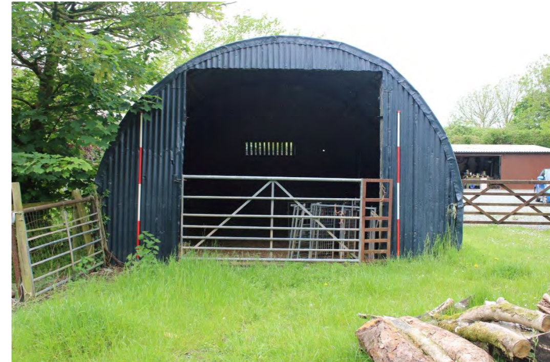
Photo 62: Eastern elevation of Building F, showing entrance and classic Nissen Hut shape
