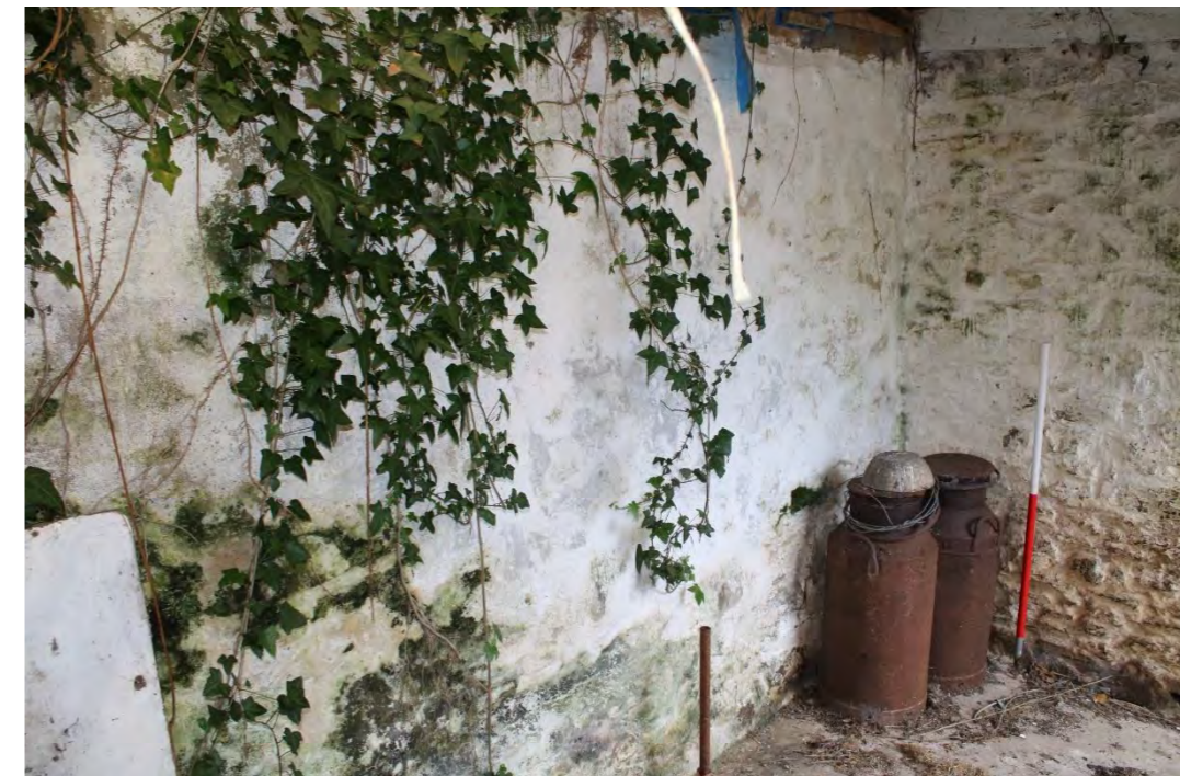
Photo 30: View southeast of eastern interior wall of Building C, which is probably a former revetment wall holding up the bank material to the east
