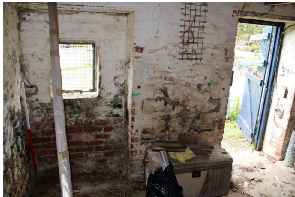
Photo 51: View of doorway and southern window in western interior wall at ground floor level within Building D, with brick blocked doorway to left
