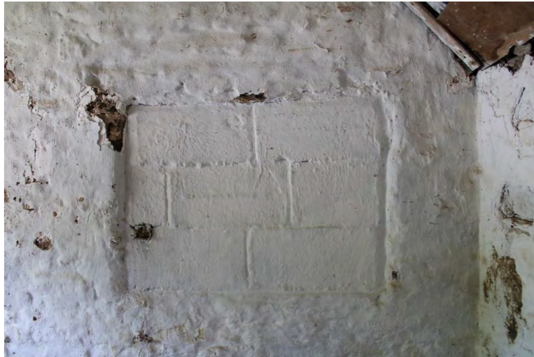
Photo 85: Detail of blocked window in northern gable end wall of Building G
