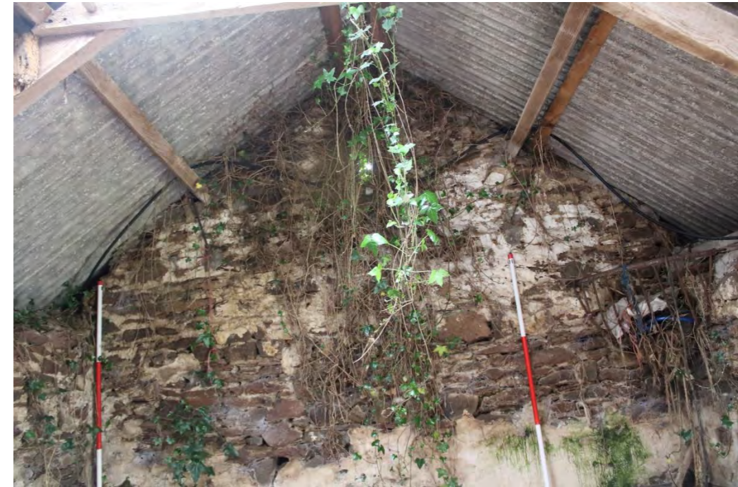
Photo 15: Eastern gable end wall of Building B showing roof structure with window light near apex of roof and feeder to right
