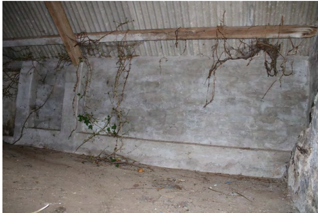
Photo 45: Northern end of western interior wall of Building D showing modern brick wall heightening
