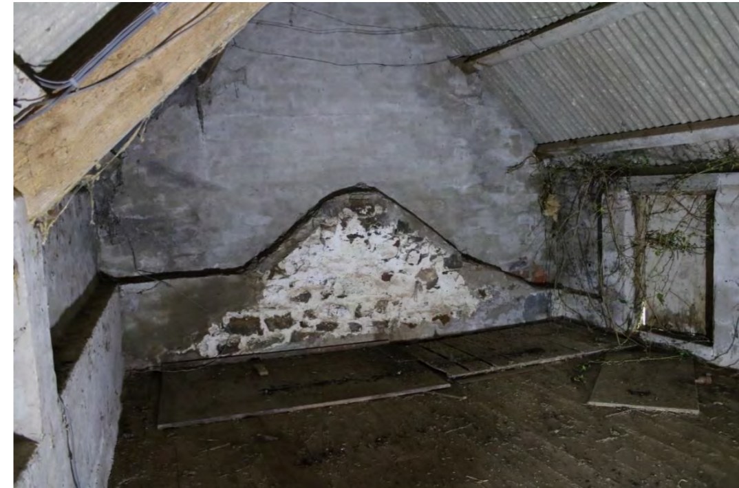
Photo 43: View of interior of southern gable end of Building D at first floor level showing original stone built gable and modern brick rebuild above, with blocked door to right
