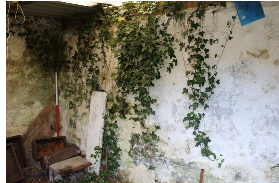
Photo 29: View northeast of eastern interior wall of Building C, which is probably a former revetment wall holding up the bank material to the east
