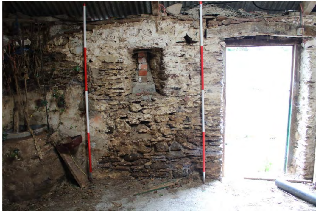
Photo 21: View of doorway and blocked splayed window in eastern half of southern interior wall of Building B
