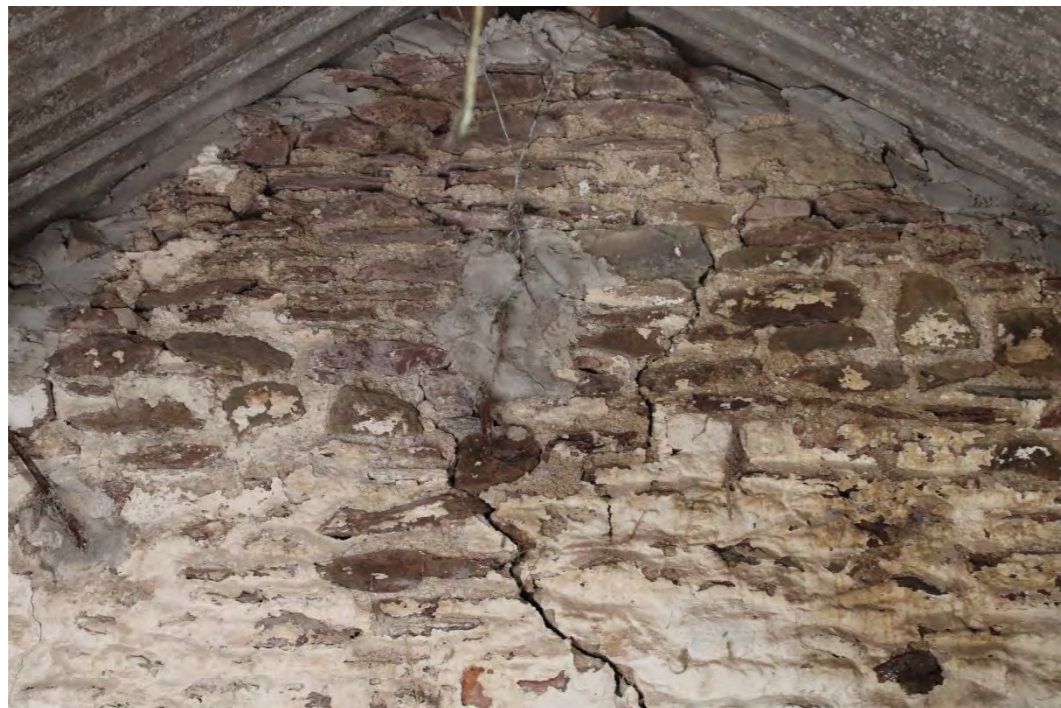
Photo 22: Detail of blocked light in upper part of interior western gable end wall of Building B
