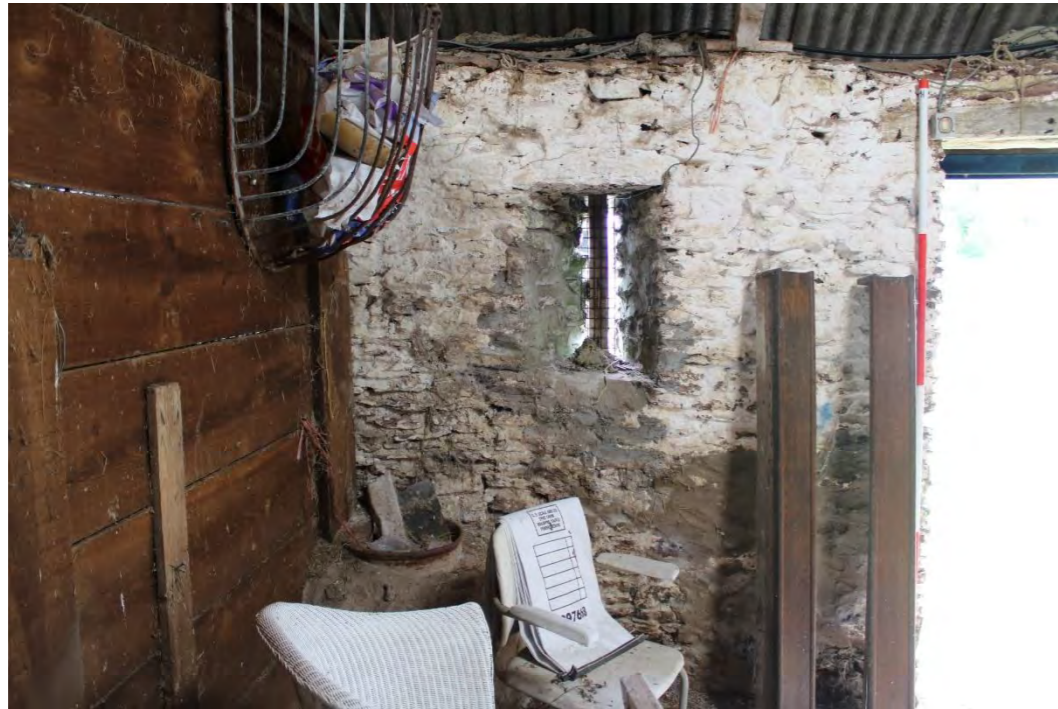
Photo 13: View of interior of southern wall of Building B showing doorway to right and central surviving splayed window with trough below and feeder above
