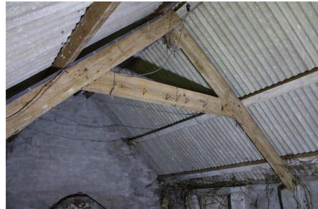
Photo 44: View south of roof structure of Building D comprising of simple A frame supported on later brick heightened walls
