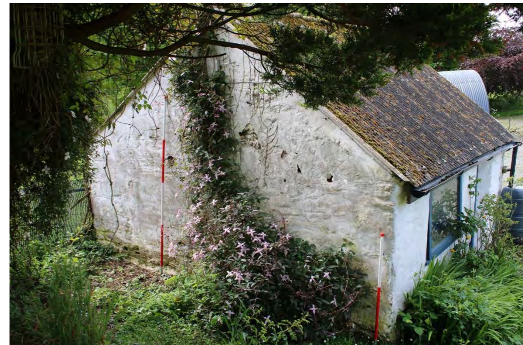
Photo 76: Northern gable end of Building G, with blocked window behind scale bar
