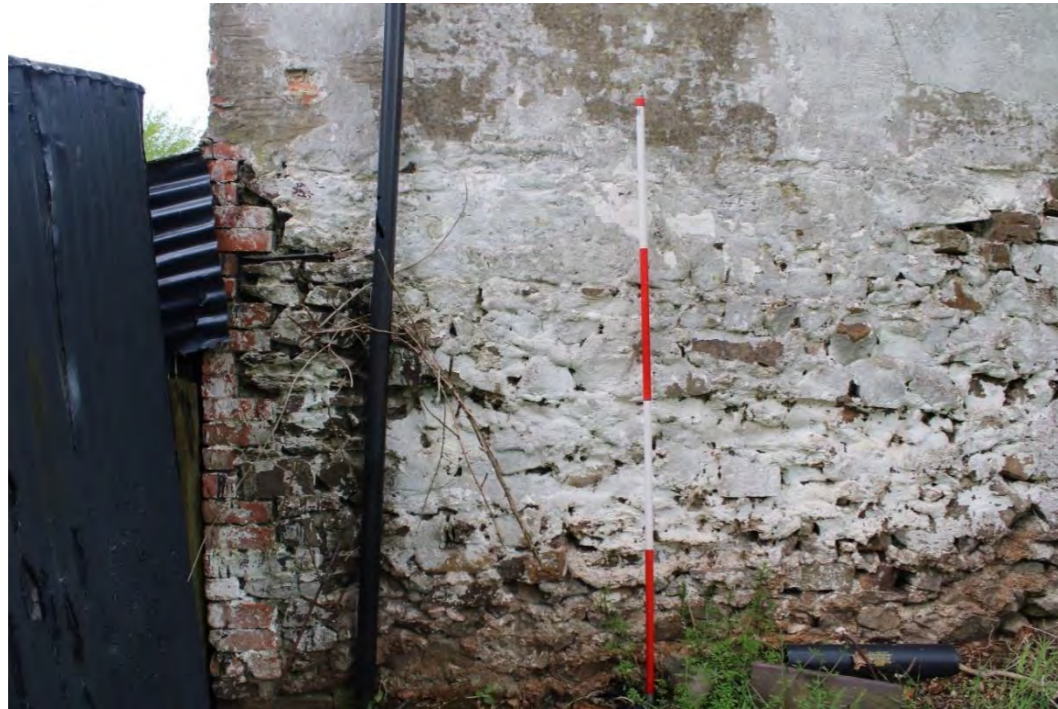
Photo 41: Detail of brick repairs on southeastern corner of Building D
