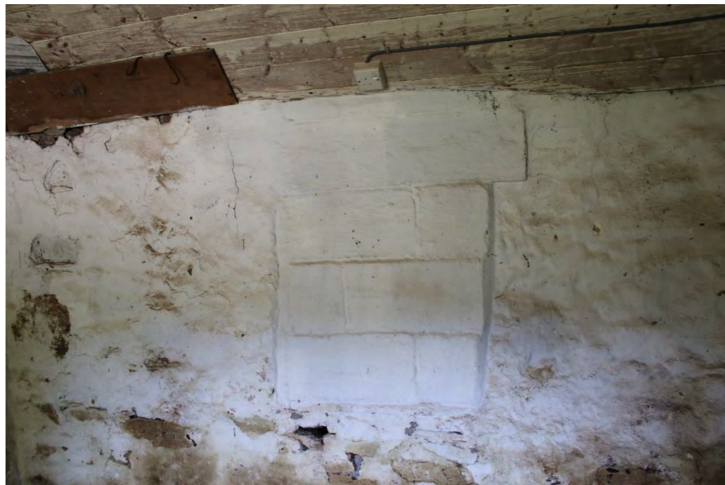
Photo 86: Interior view showing detail of blocked window in eastern wall of Building G
