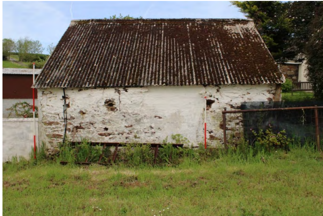
Photo 77: Eastern elevation of Building G from within main farm courtyard with blocked window to left of right hand scale bar
