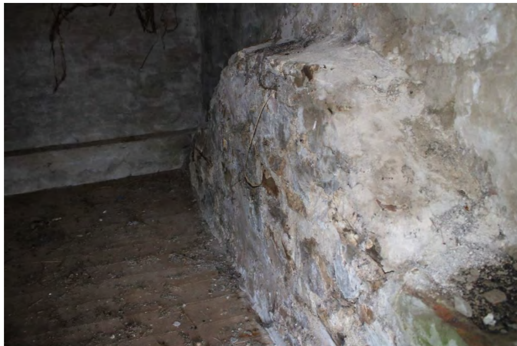
Photo 46: Top of original stone northern gable end wall, with brick heightening above
